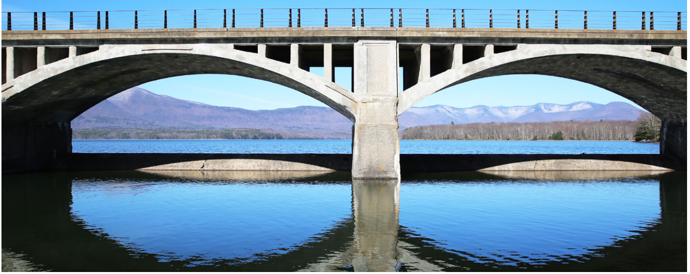
Dividing Weir Bridge from East Basin into West Basin, Ashokan Reservoir
