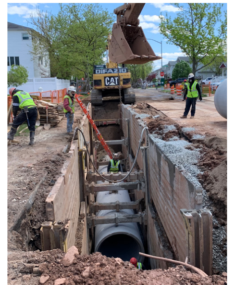
$10M Drainage Upgrade for Bay Terrace, Staten Island
