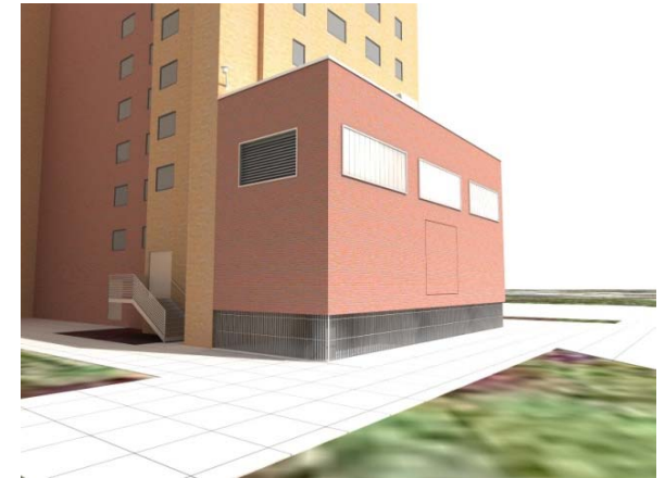
Electric Meter Room Extension
