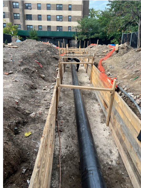
Linden - Steam Main Repaired
