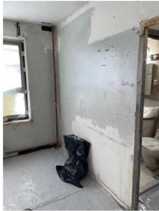
Abated bedroom wall (Building 3, Apt. 1A)
