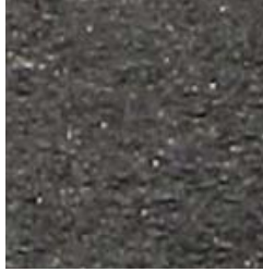
BIKE LANE PAVING
