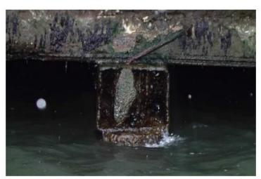
Deteriorating timber pile caps
