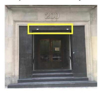
This picture shows the existing storefront. The soffit is highlighted below. When in the up position, gate will be fully covered by soffit.
