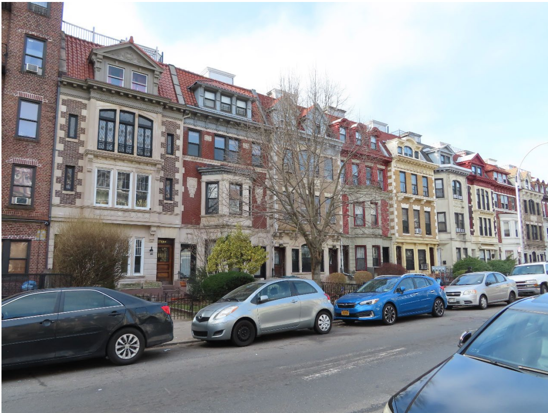
Parkside Avenue (south side) LPC 2021
