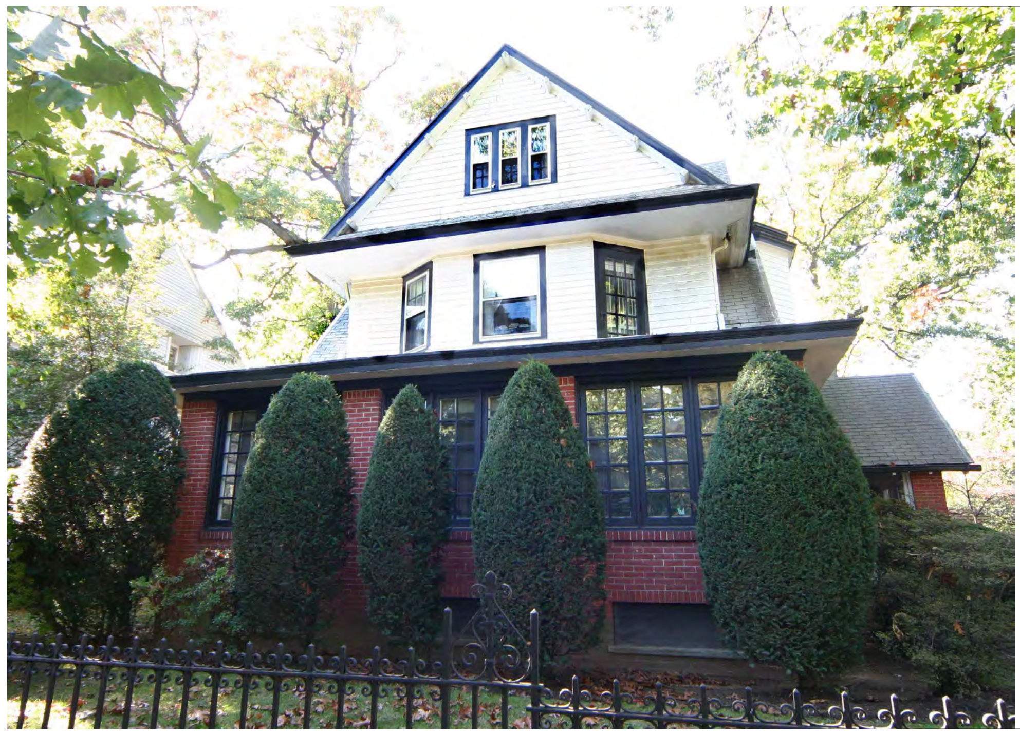
EAST FACADE DESIGNATION PHOTO
