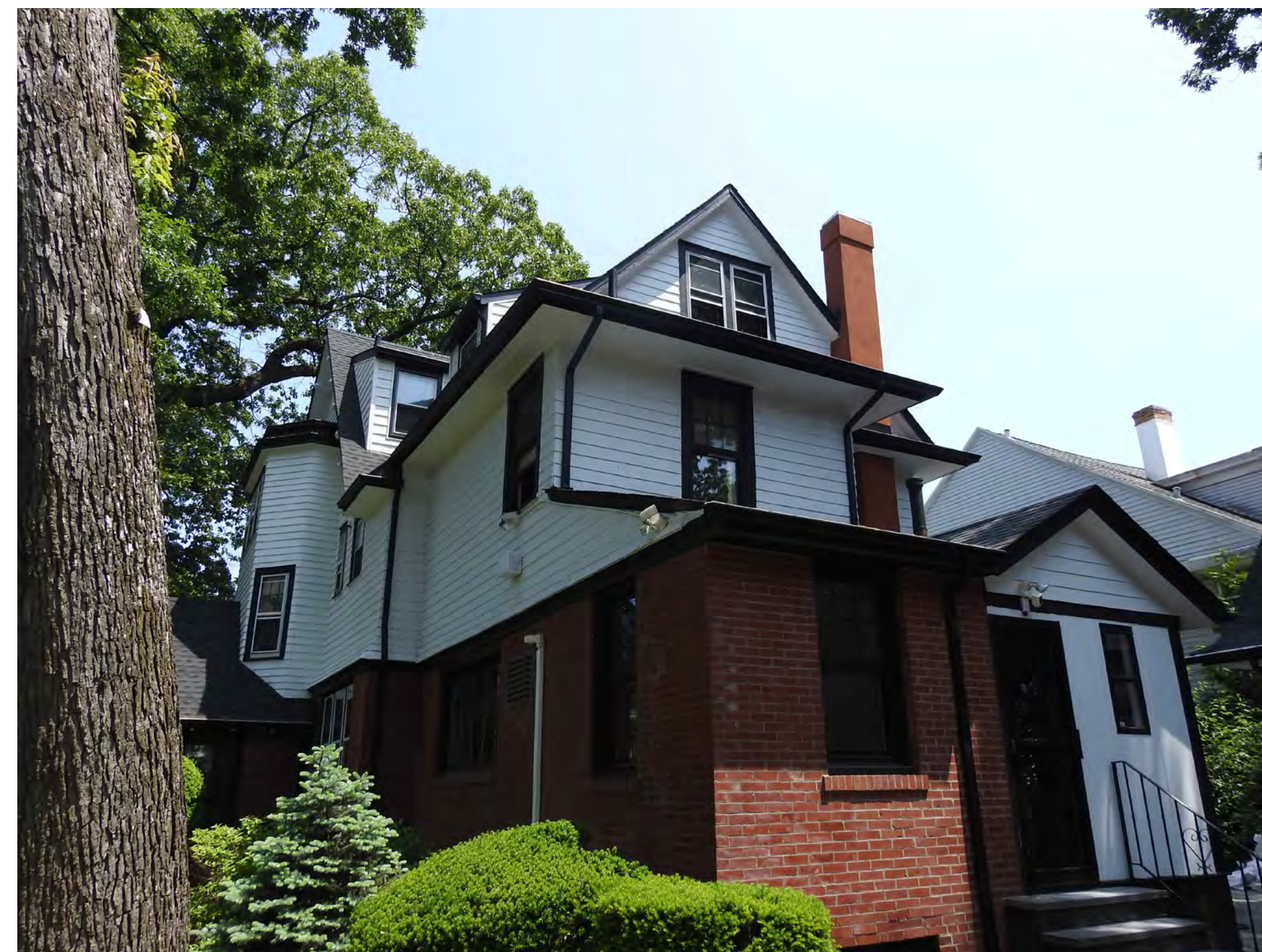
EXISTING BUILDING SIDE VIEW
