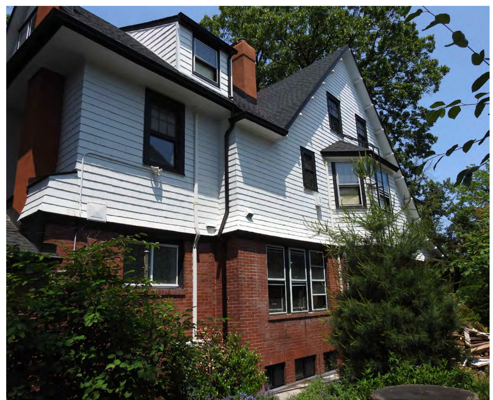
EXISTING BUILDING REAR PHOTO
