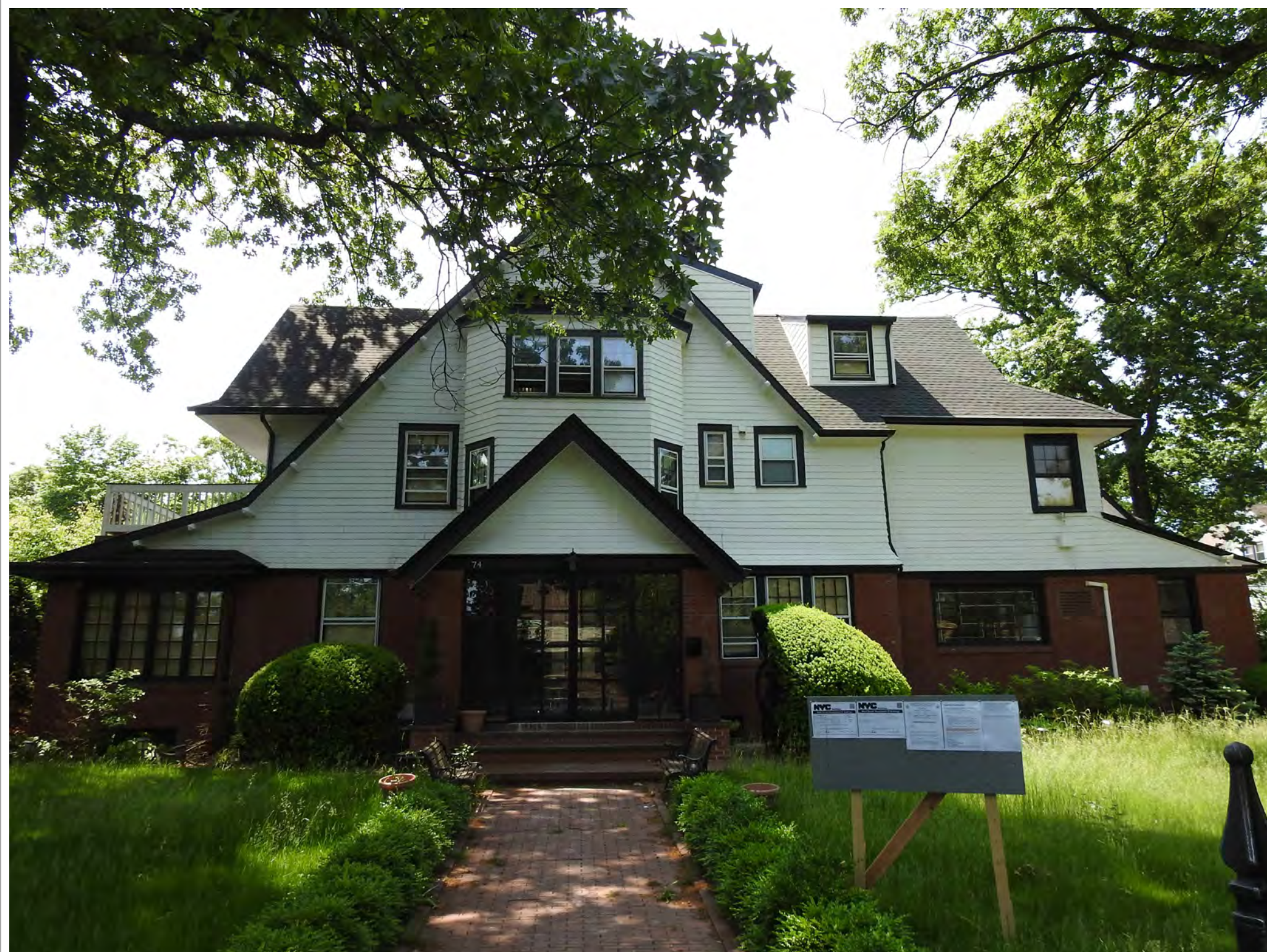
EXISTING BUILDING FRONT VIEW
