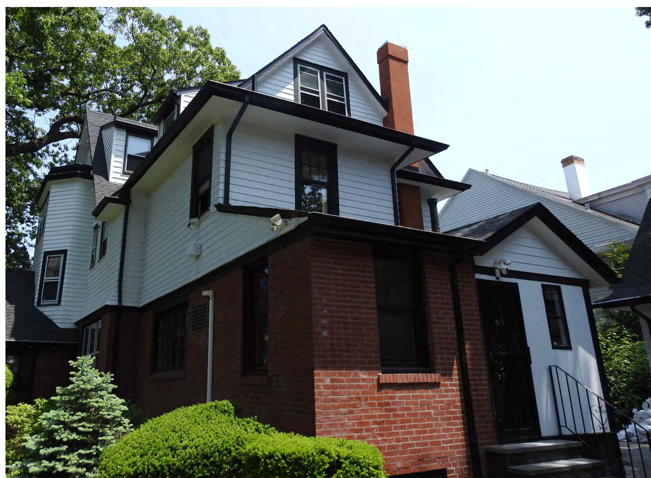
EXISTING BUILDING WEST SIDE PHOTO
