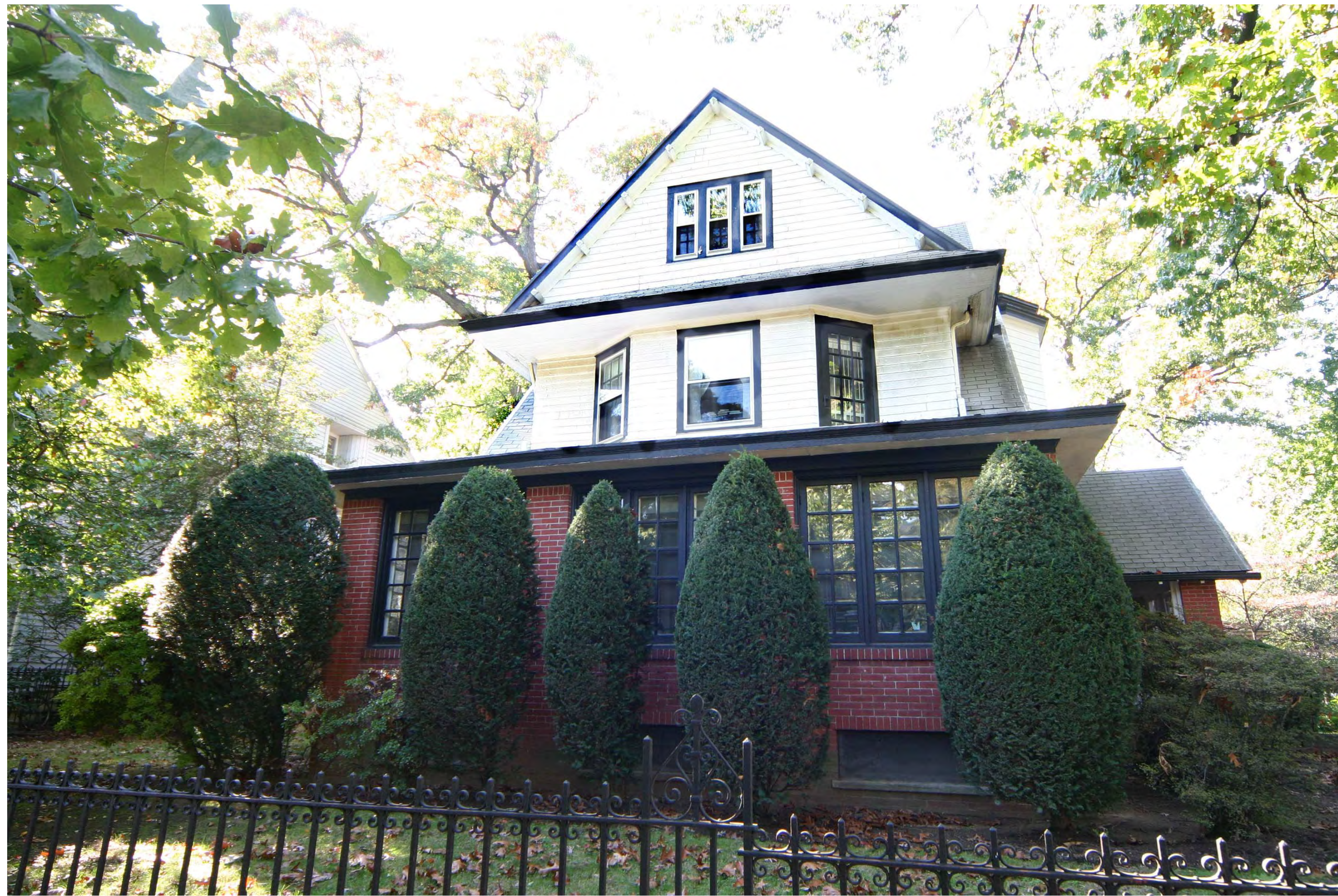
EAST FACADE DESIGNATION PHOTO
