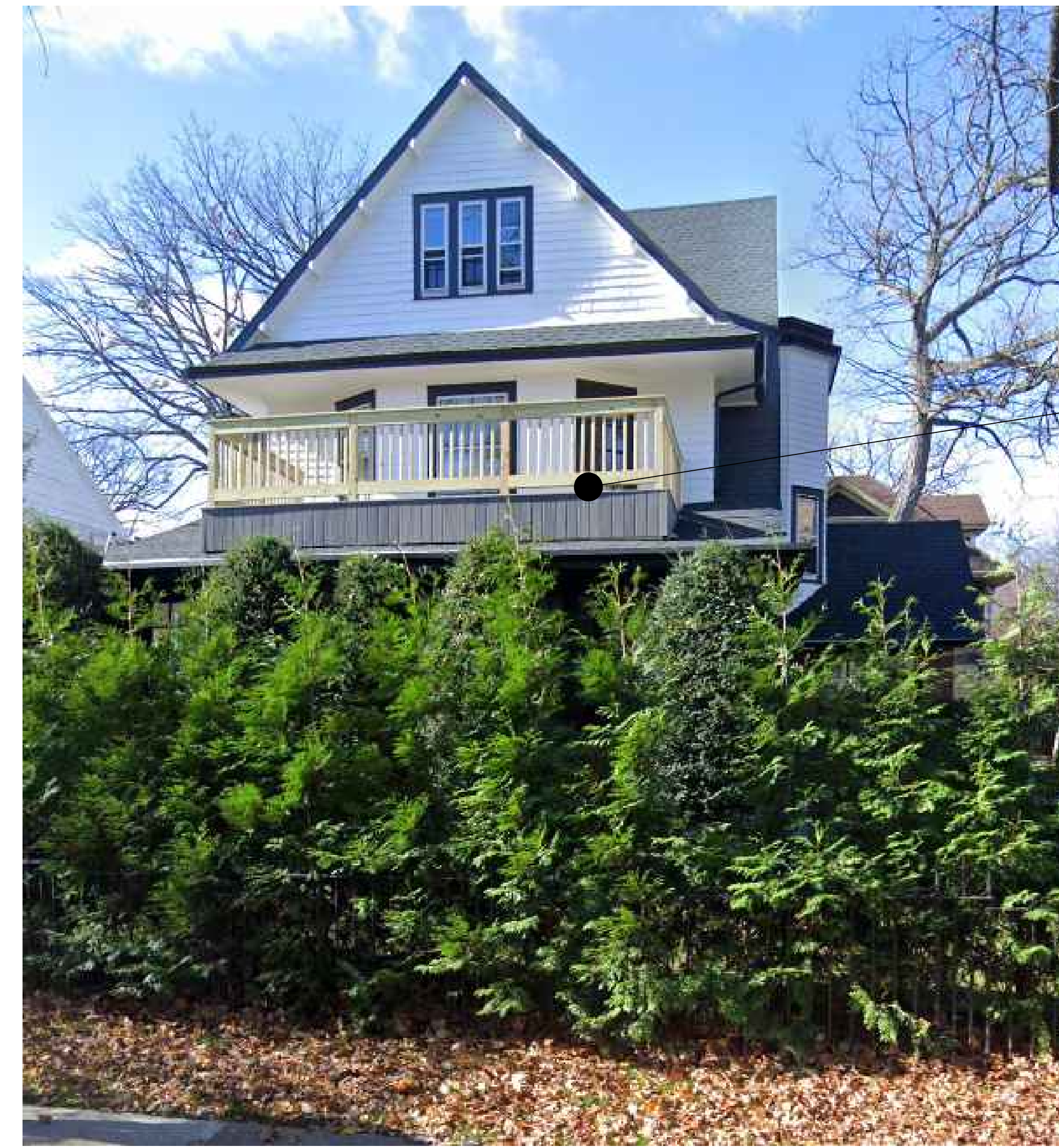
EAST FACADE EXISTING CONDITION PHOTO
