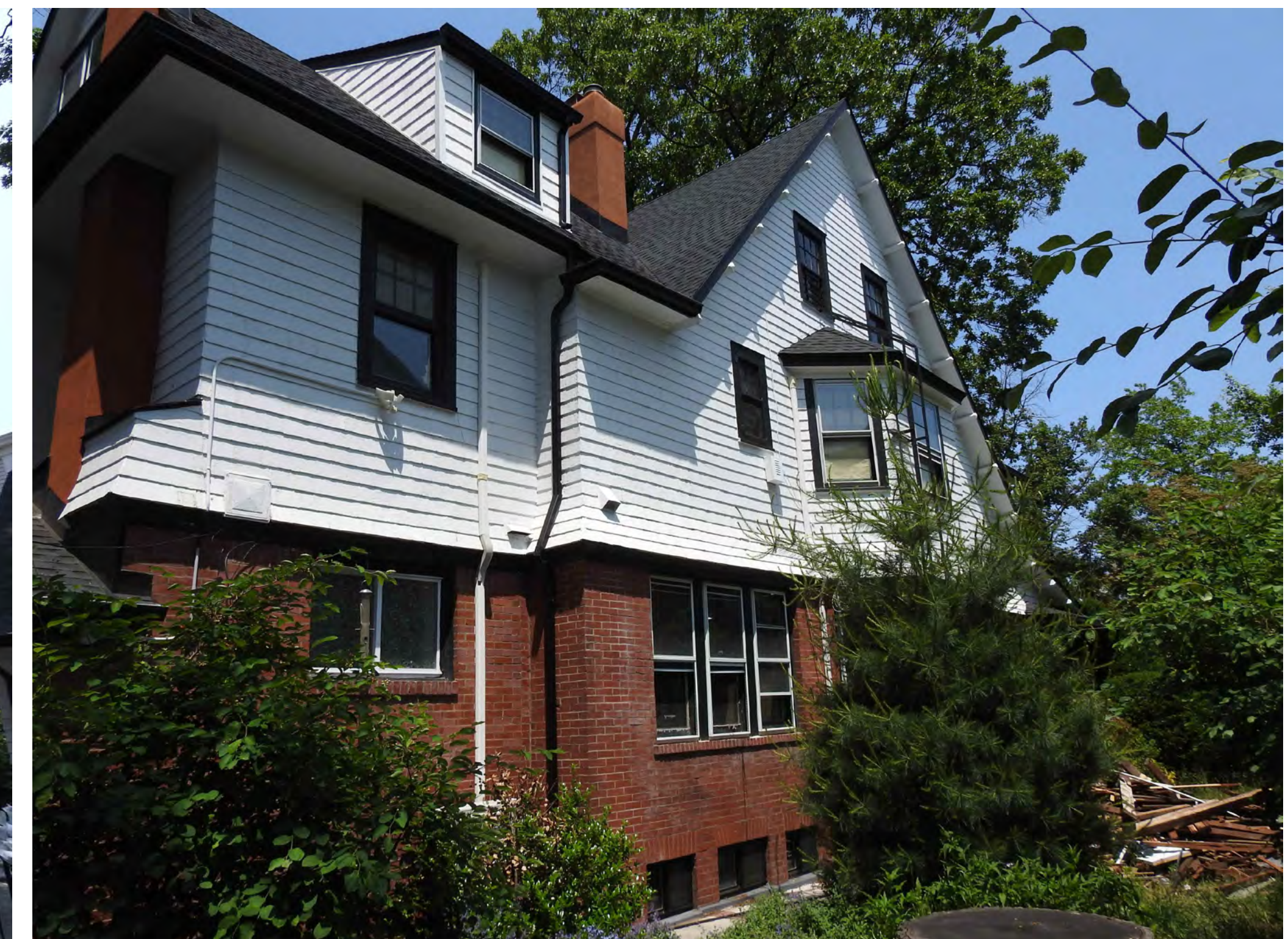
EXISTING BUILDING REAR VIEW
