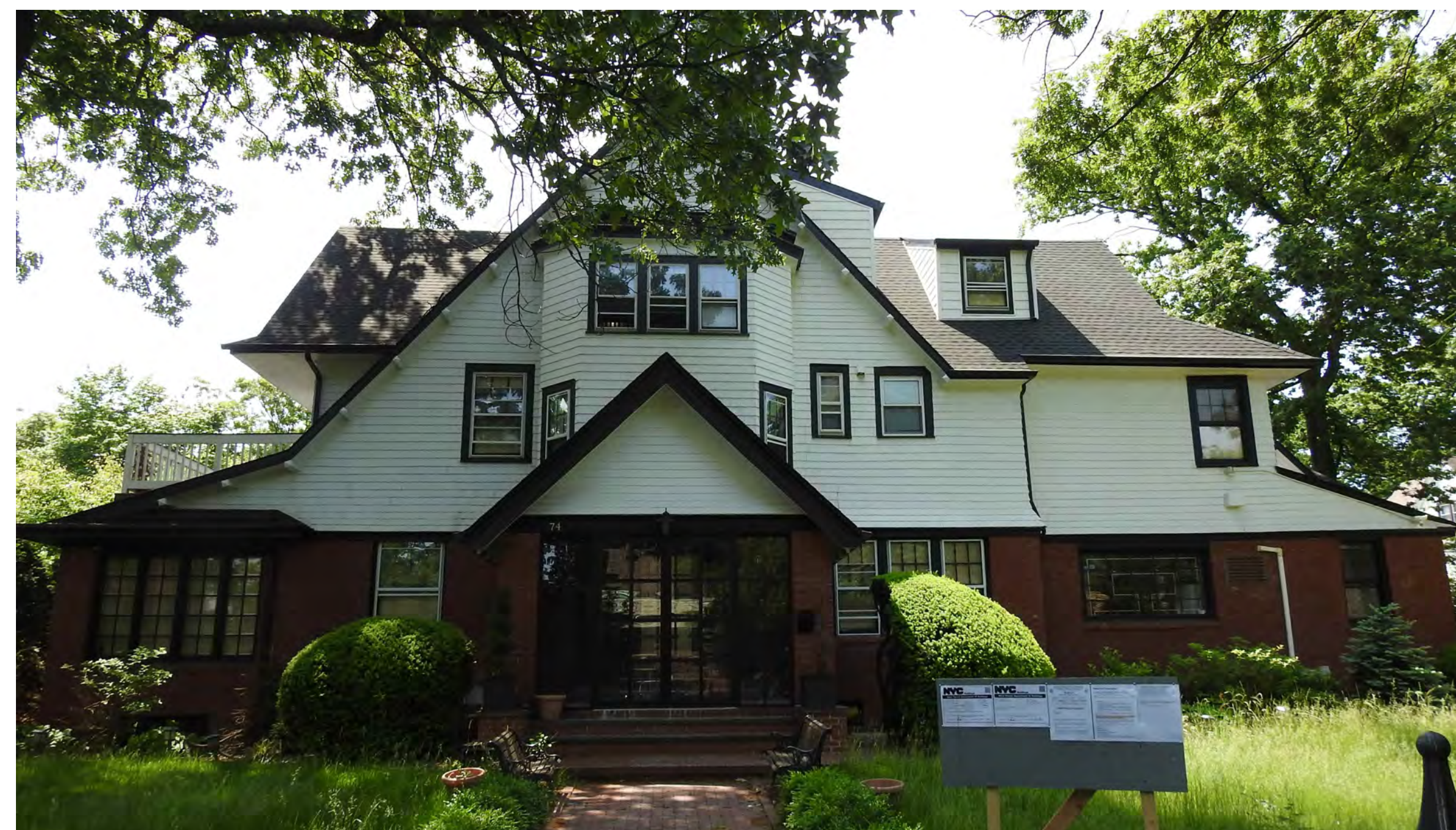
EXISTING BUILDING FRONT PHOTO
