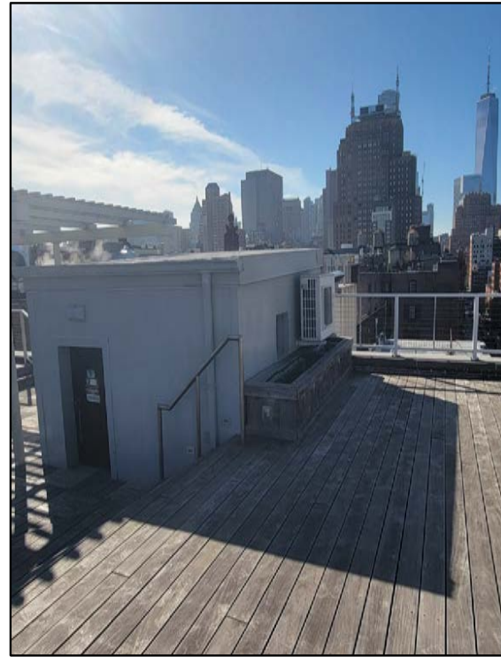
7 VIEW OF PASSENGER ELEVATOR FROM WEST SIDE
