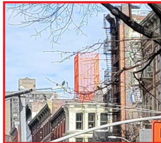
5* ENLARGED VIEW FROM NORTHWEST CORNER
