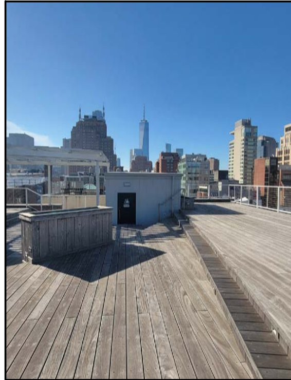
1 VIEW OF PASSENGER ELEVATOR FROM NORTH SIDE
