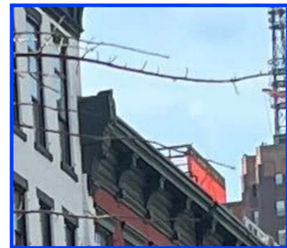
6* ENLARGED VIEW FROM CORNER
