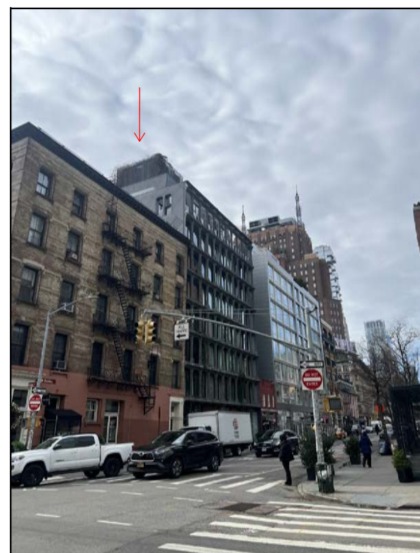
23 VIEW FROM CORNER OF W BROADWAY & GRAND ST NEW CONSTRUCTION
