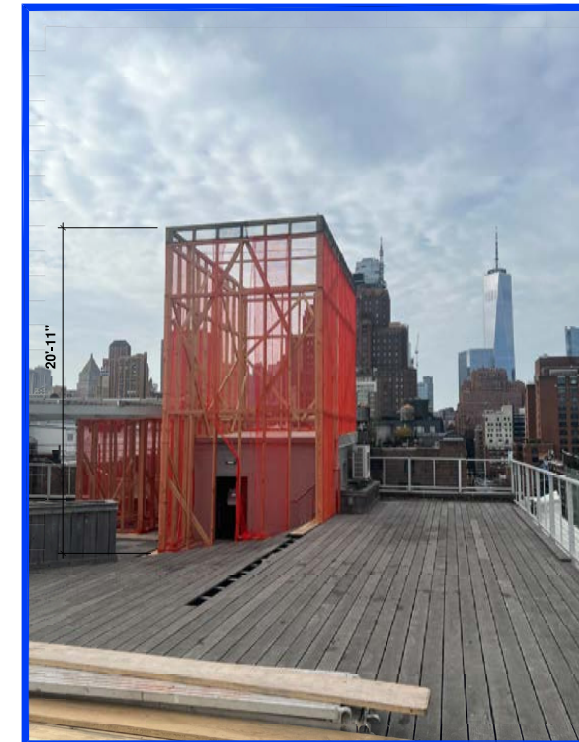
7' VIEW OF PASSENGER ELEVATOR FROM WEST SIDE
