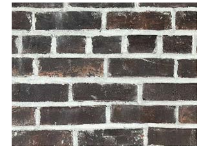
MATERIAL 2: EXISTING BRICK WALL
