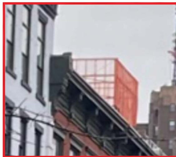
6* ENLARGED VIEW FROM CORNER
