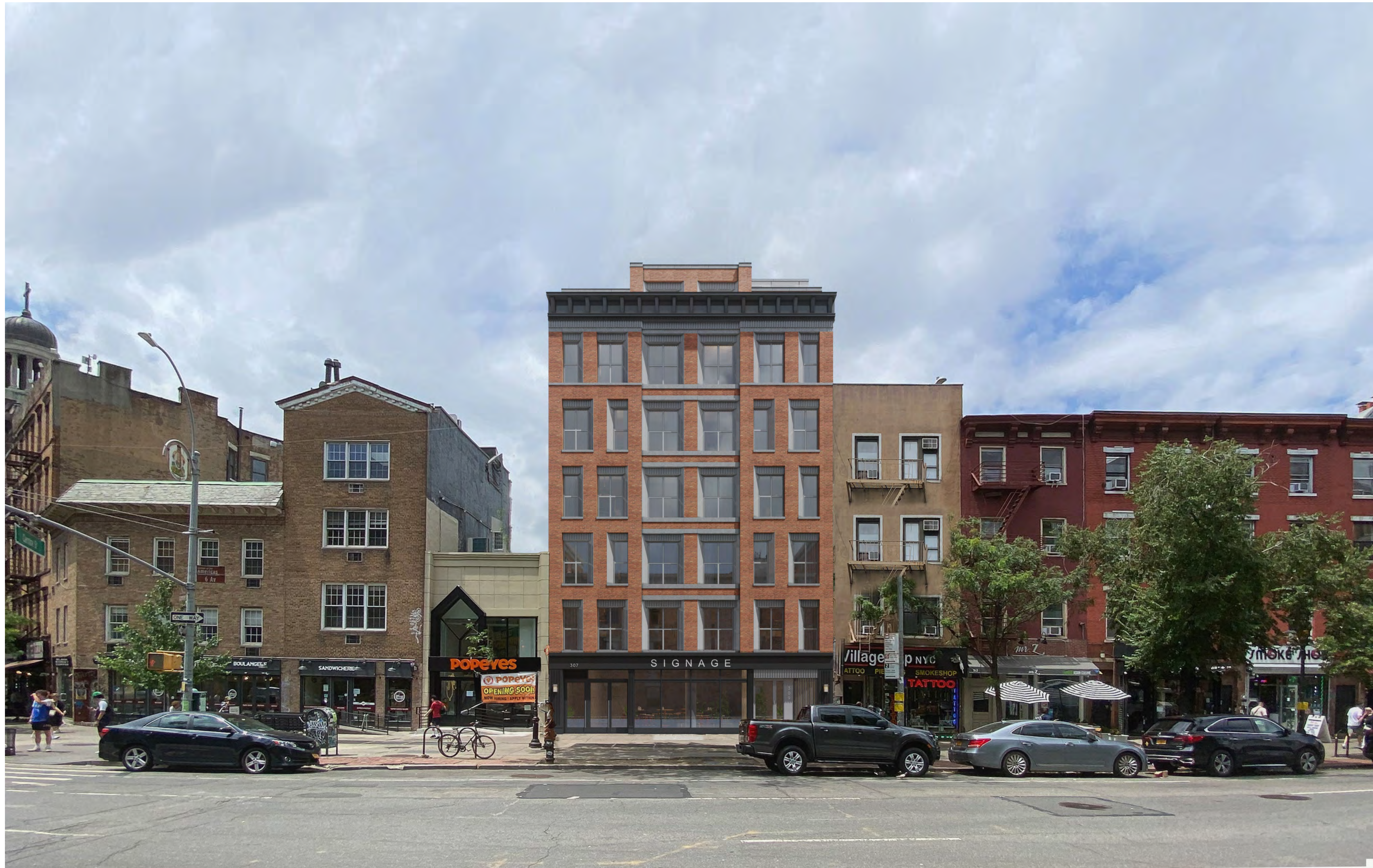
307-309 SIXTH AVENUE LANDMARKS PRESERVATION COMMISSION APRIL 16, 2024
