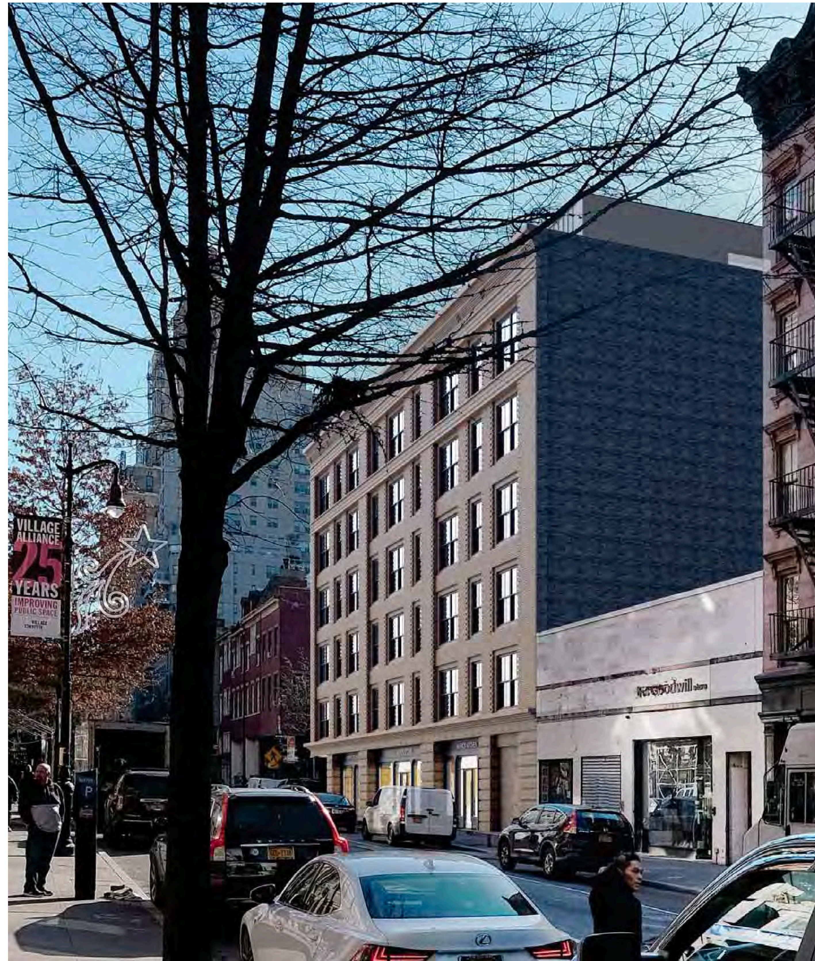
38 West 8th Street Approved 2019 (currently under construction)
