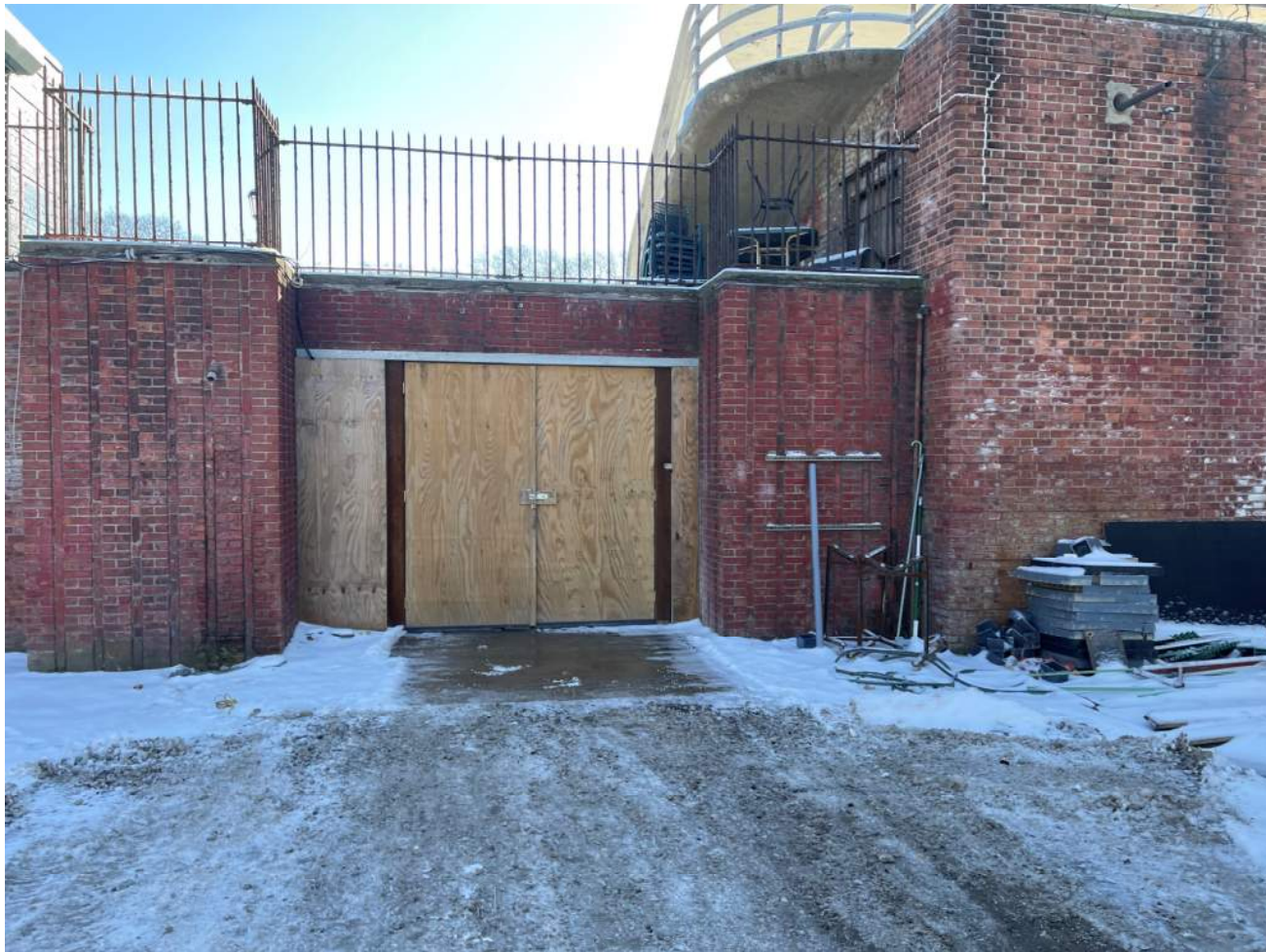
EXISTING FILTER BUILDING – TEMPORARY DOORS
