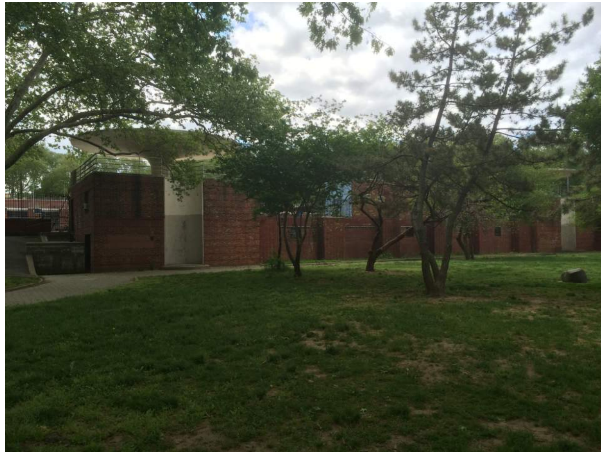
EXISTING FILTER BUILDING
