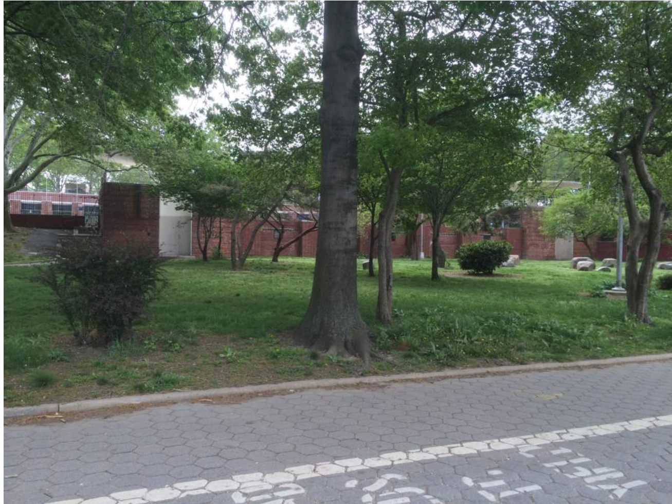
EXISTING FILTER BUILDING
