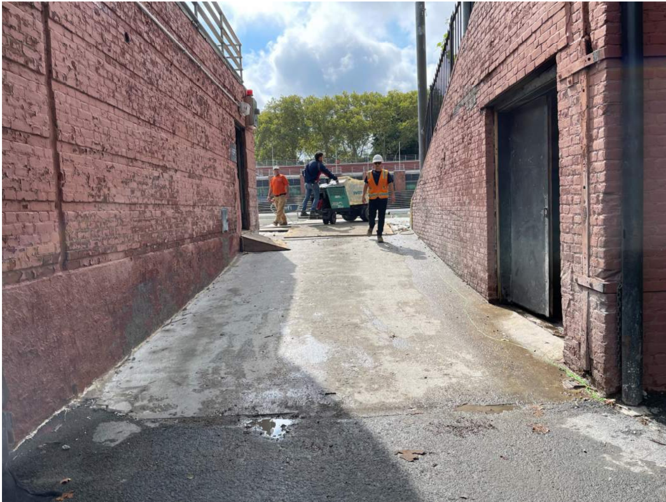
EXISTING DOUBLE DOORS ALONG THE SERVICE RAMP TO THE POOL
