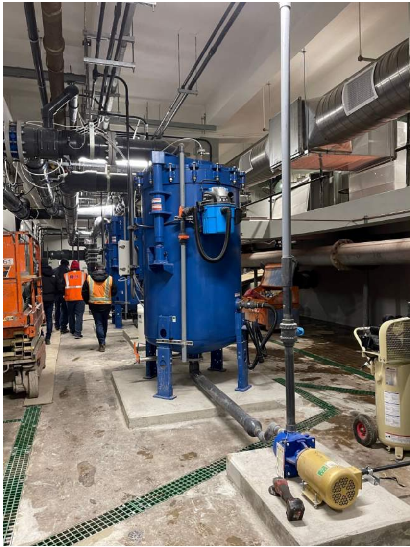
PHOTO A: INTERIOR OF FILTER BUILDING
