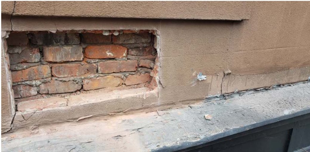
Exterior View: showing proposed enlargement probe #3
