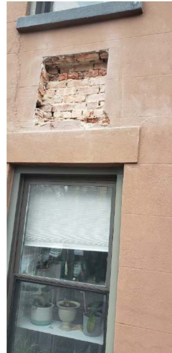
Exterior View: showing proposed enlargement probe # 2
