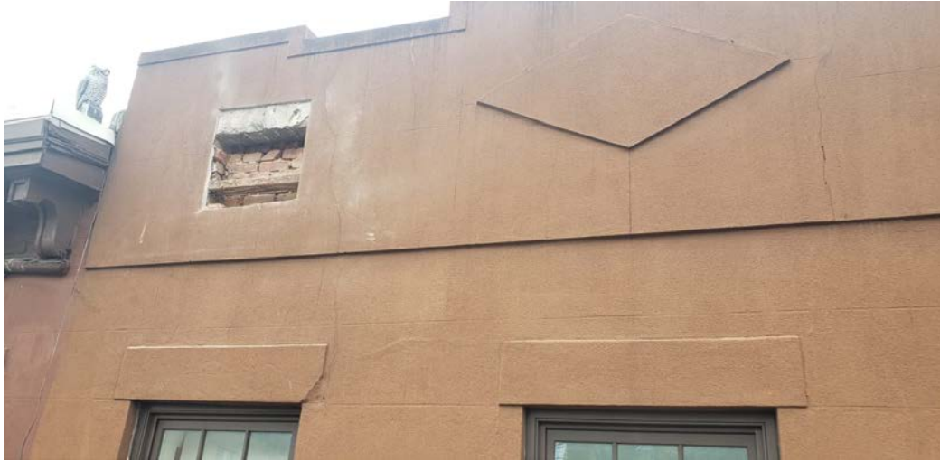
Exterior View: showing proposed probe #1
