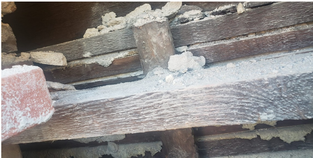
Exterior View: showing proposed enlargement probe #2
