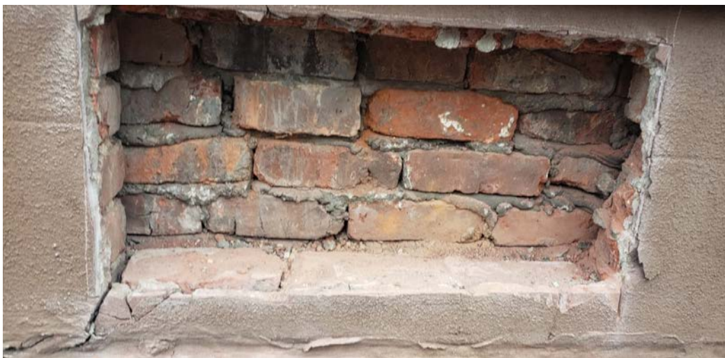
Exterior View: showing proposed enlargement probe #3
