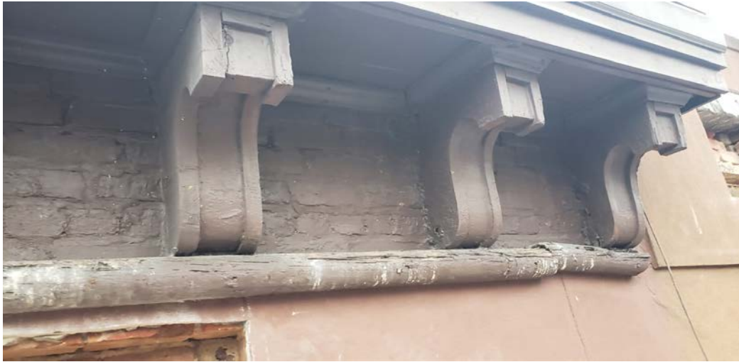
Exterior View: showing proposed probe #1 & cornice
