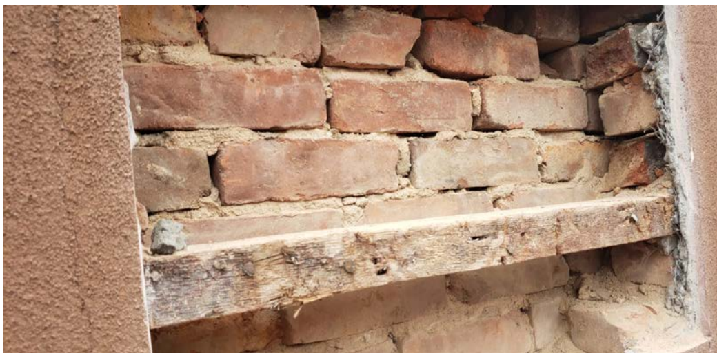
Exterior View: showing proposed enlargement probe #1
