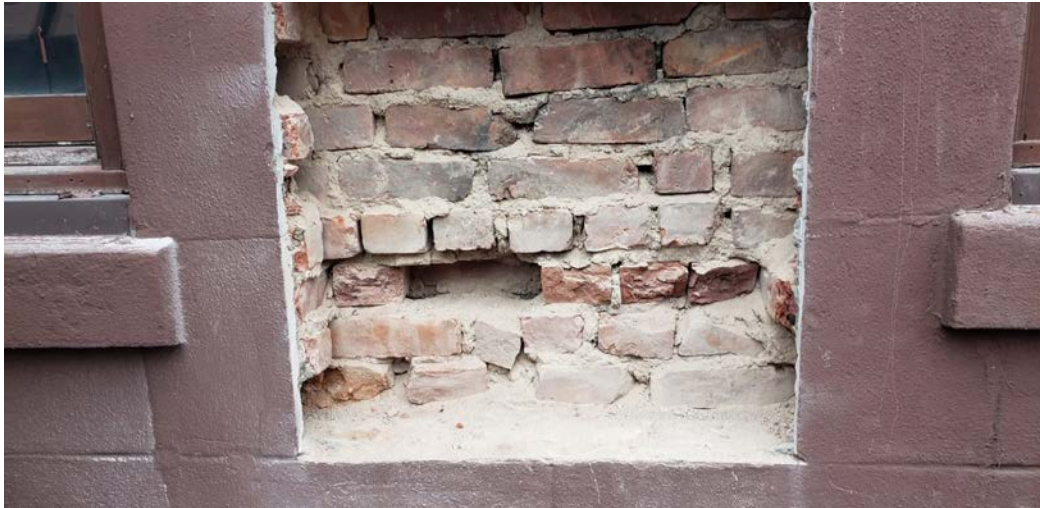
Exterior View: showing proposed enlargement probe #3
