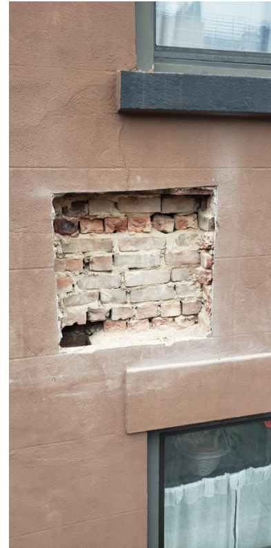
Exterior View: showing proposed enlargement probe # 3
