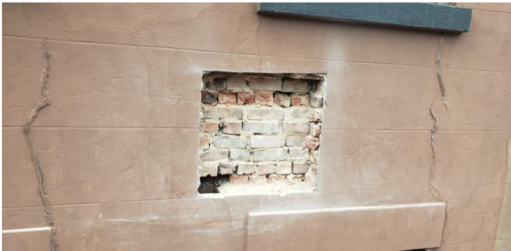
Exterior View: showing proposed enlargement probe # 3
