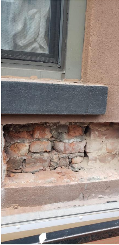
Exterior View: showing proposed enlargement probe # 1
