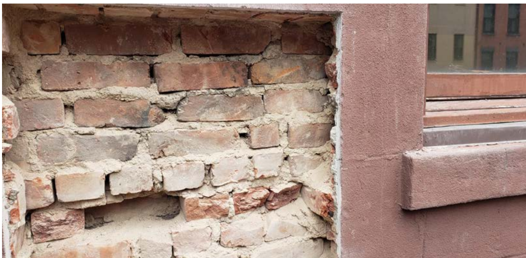
Exterior View: showing proposed enlargement probe #3
