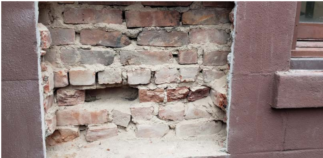
Exterior View: showing proposed enlargement probe #3
