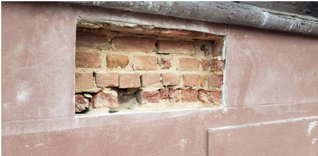
Exterior View: showing proposed enlargement probe #1
