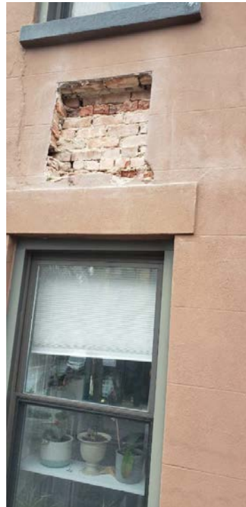
Exterior View: showing proposed enlargement probe # 2
