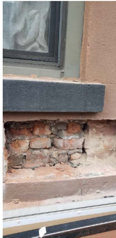
Exterior View: showing proposed enlargement probe # 1
