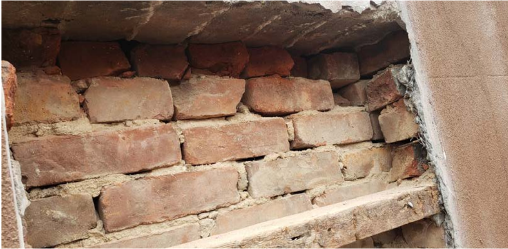
Exterior View: showing proposed enlargement probe #1
