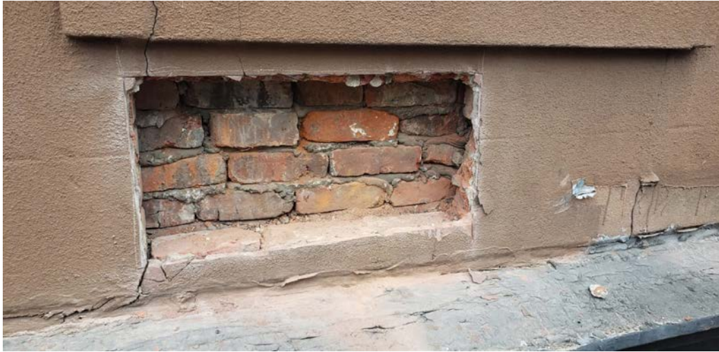
Exterior View: showing proposed enlargement probe #3
