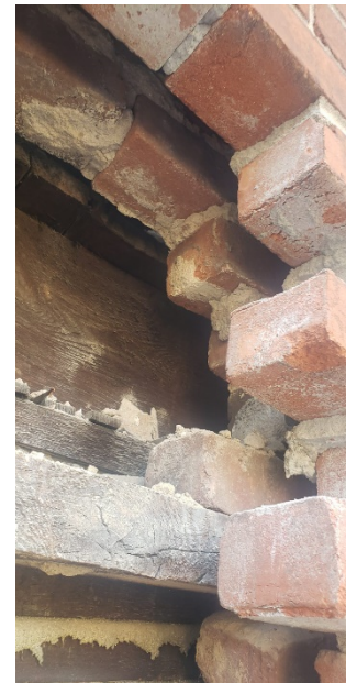
Exterior View: showing proposed enlargement probe #2
