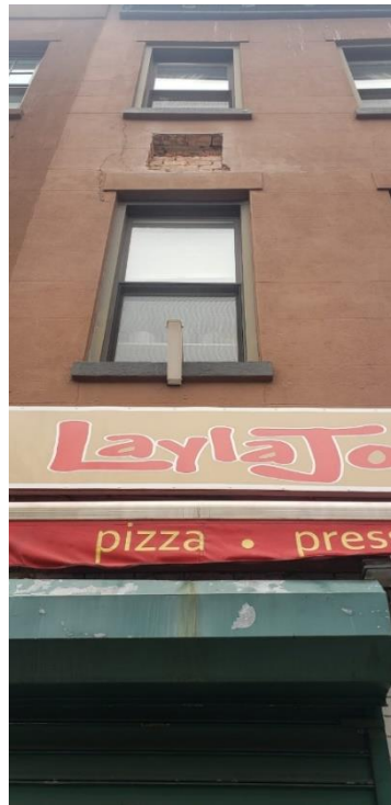
Exterior View: showing proposed probe # 2 location
