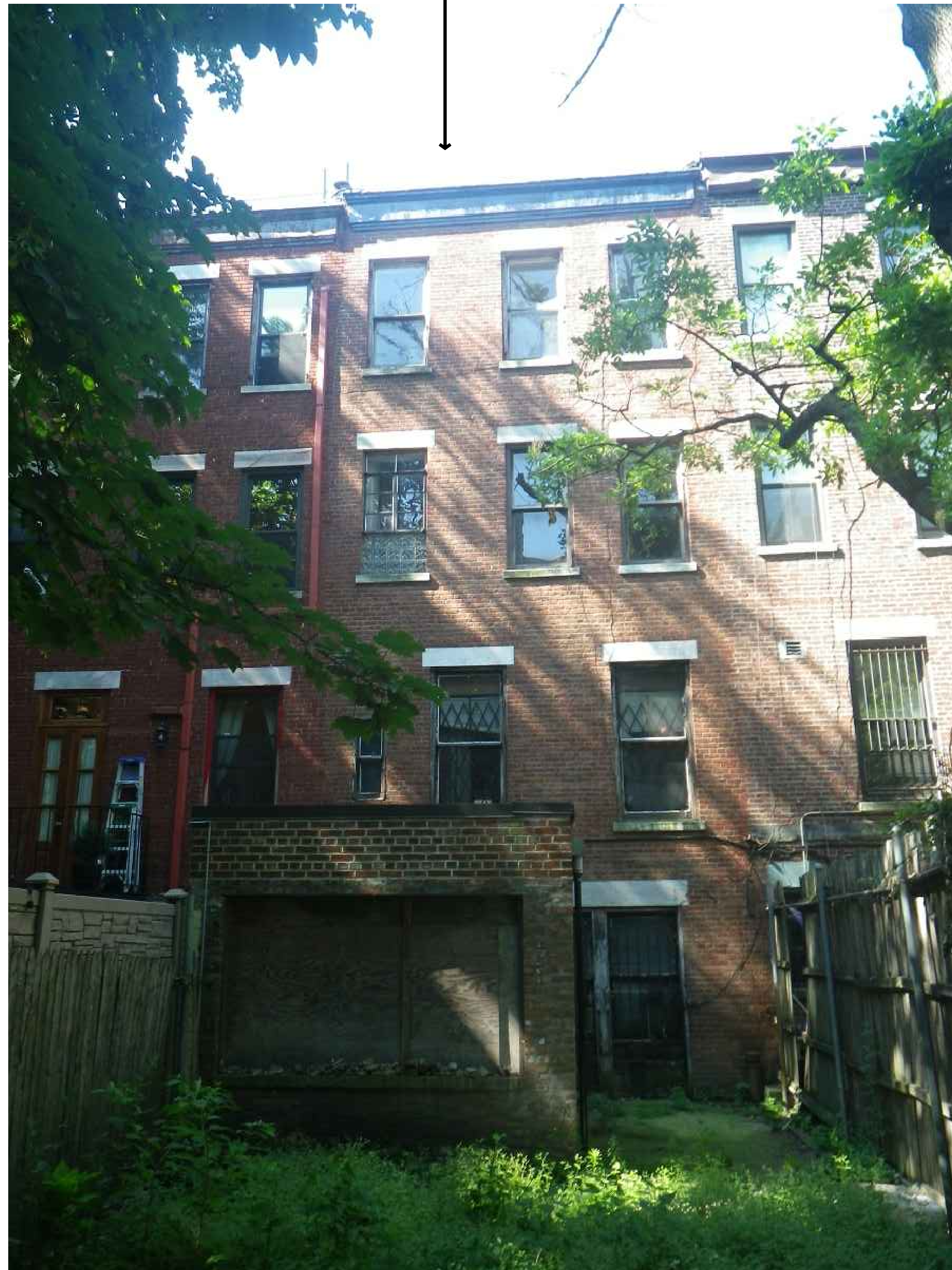
PHOTO 1: REAR / SECONDARY FACADE
