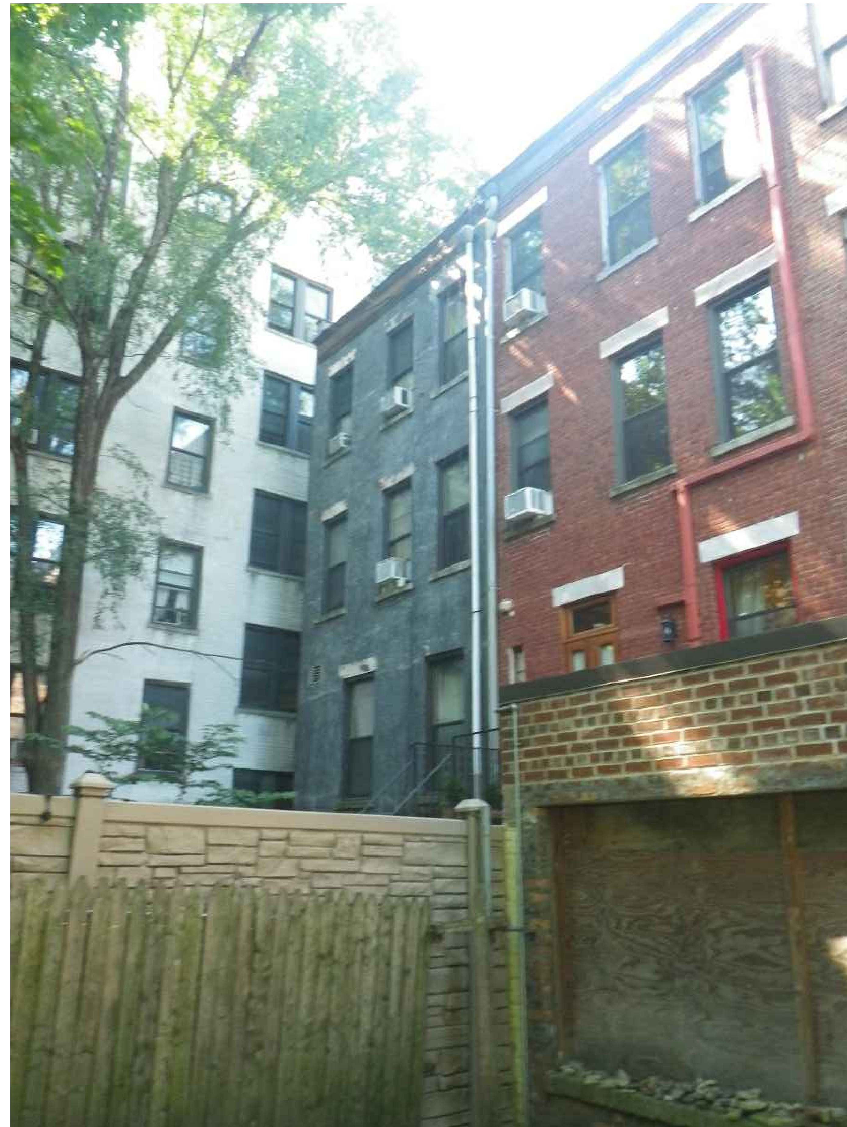
PHOTO 2: REAR / SECONDARY FACADE & ADJACENT BUILDING
