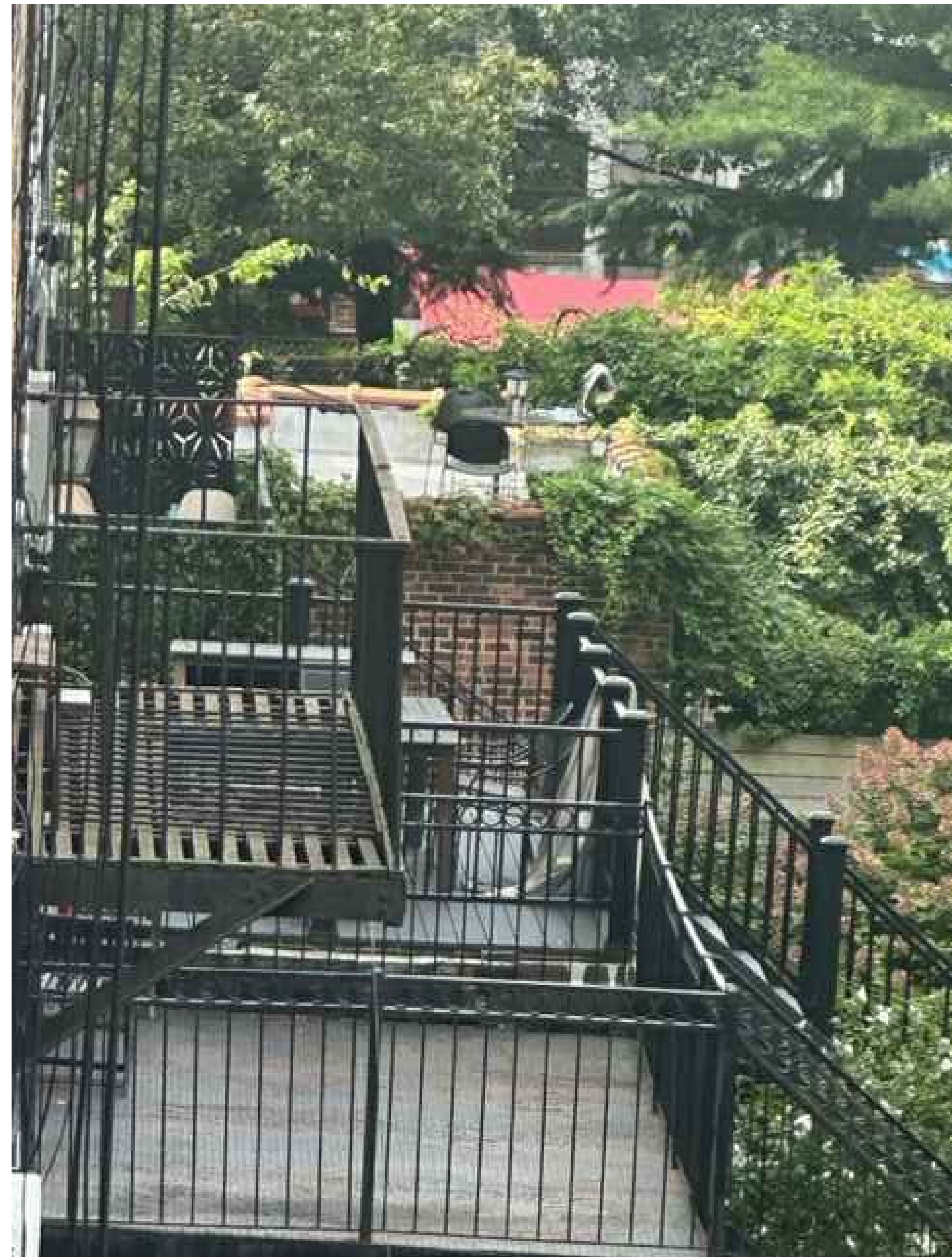
PHOTO 2: ADDITION @ NEIGHBORING PROPERTY
