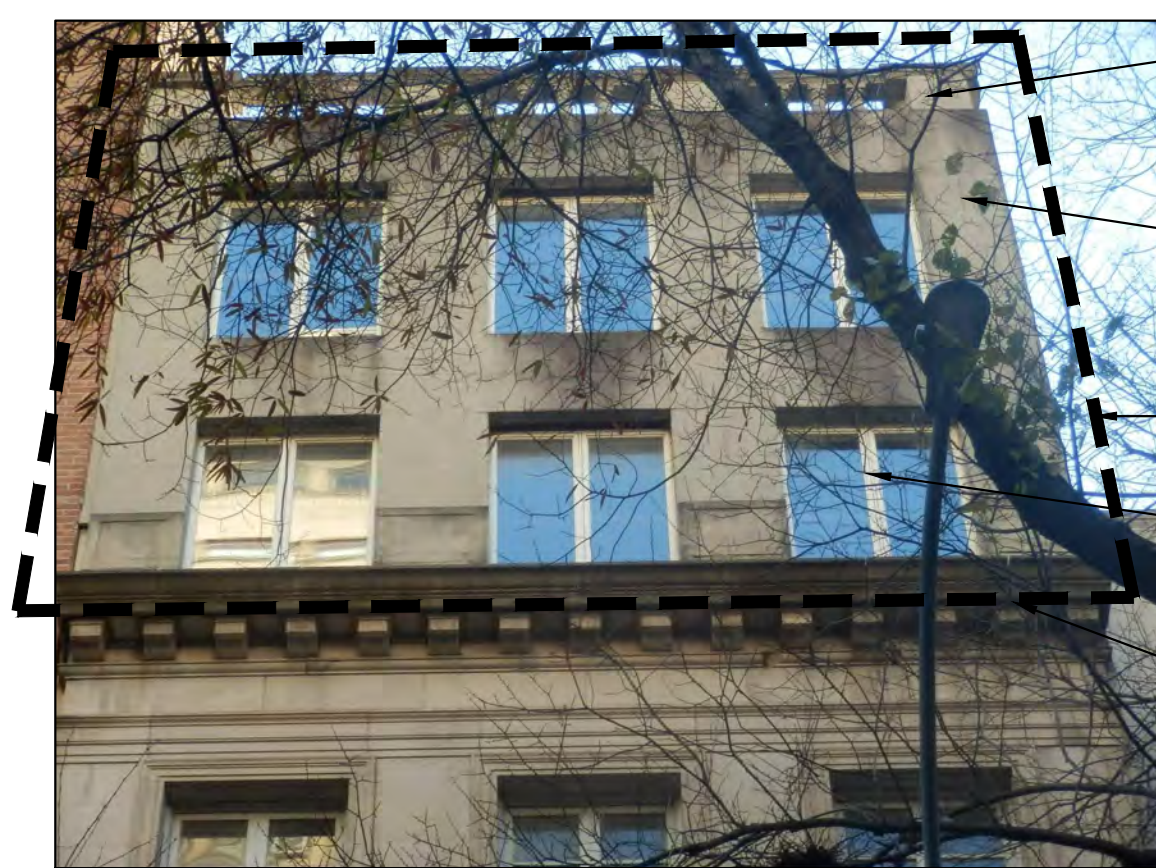
4 Existing North Facade Photo 5th and 6th Floors Scale: NA
