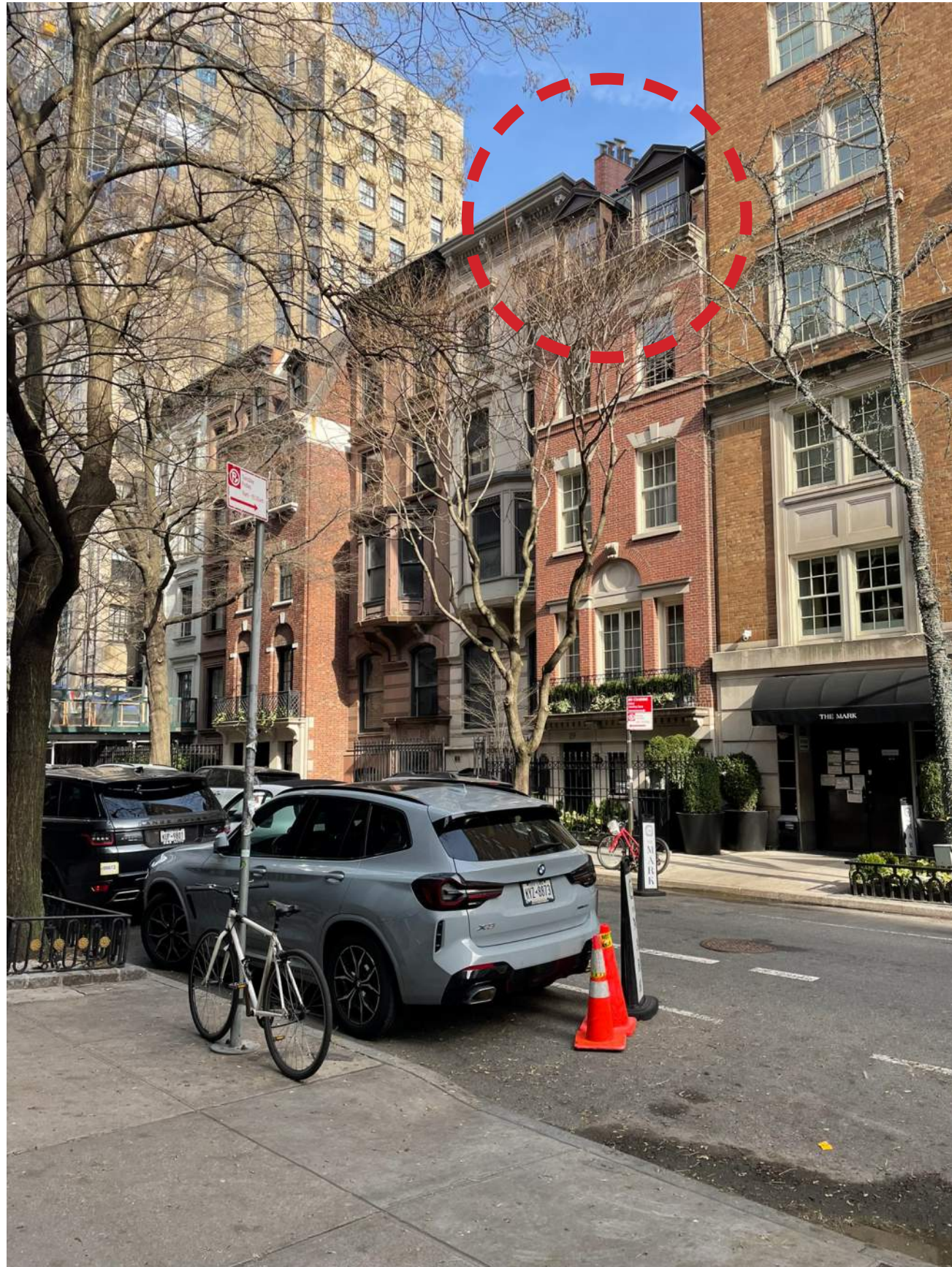
Rendered Flues: View from 77th Street
