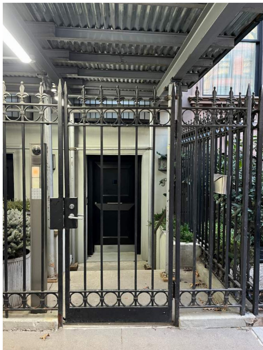
Areaway at 9 E77th Street
