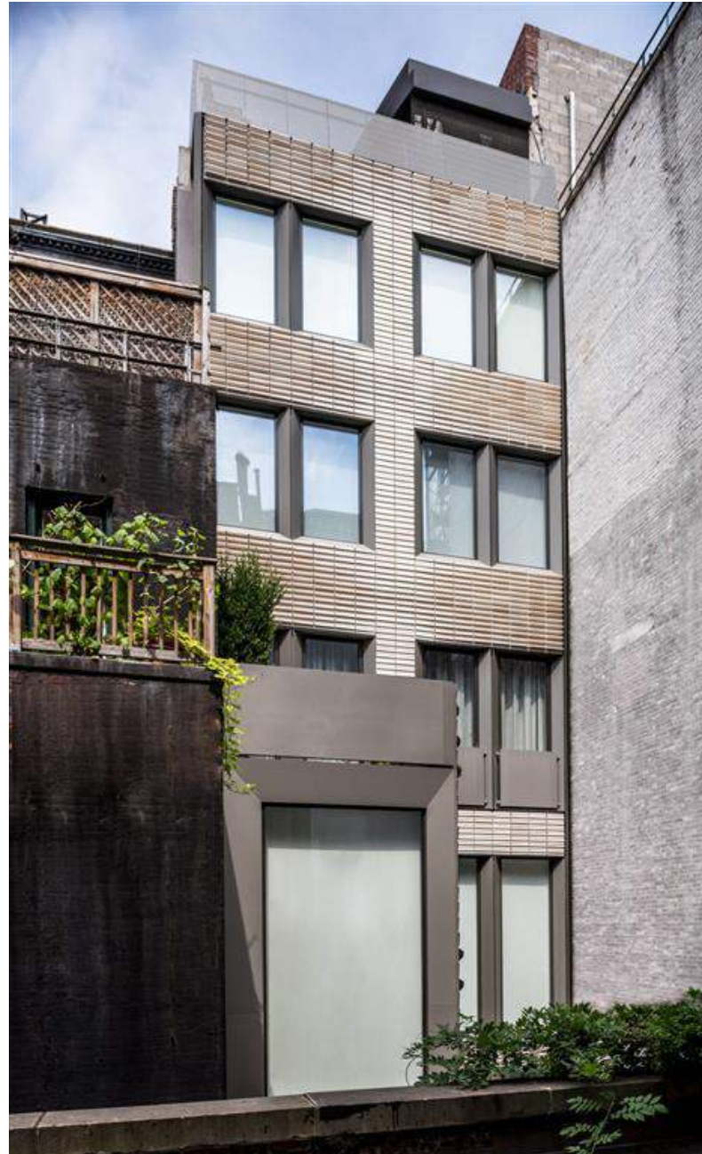
34 East 68th Street Terra-cotta rear elevation, COFA 16-3349
