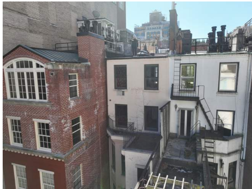
Existing Rear Facade at 15-17 E77th Street
