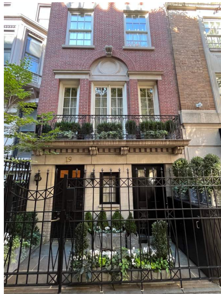
Areaway at 19 E77th Street
