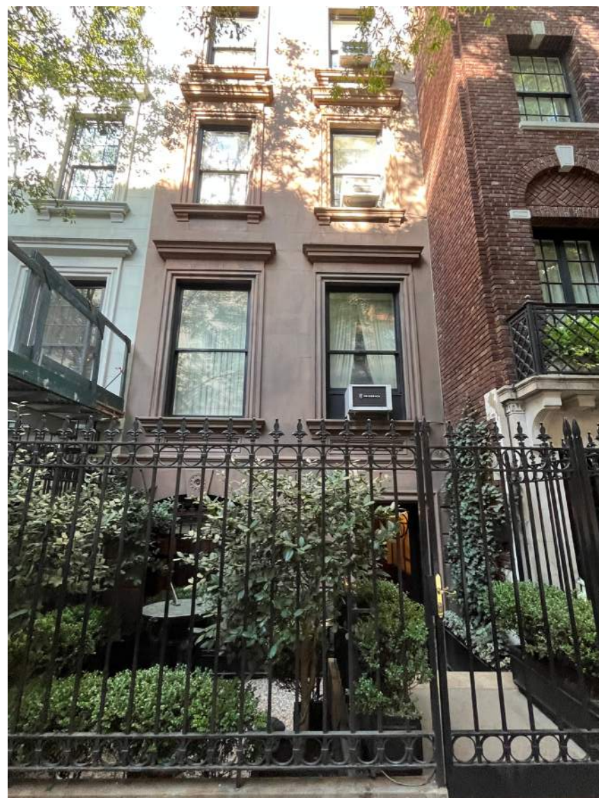
Areaway at 11 E77th Street
