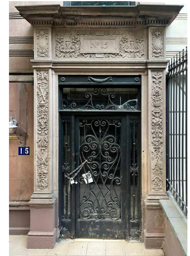
Existing Stone Door Surround at 15 E77th Street
