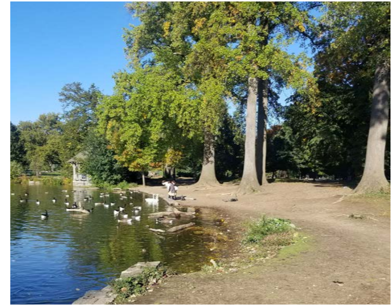
Broken retaining wall and eroded soil
