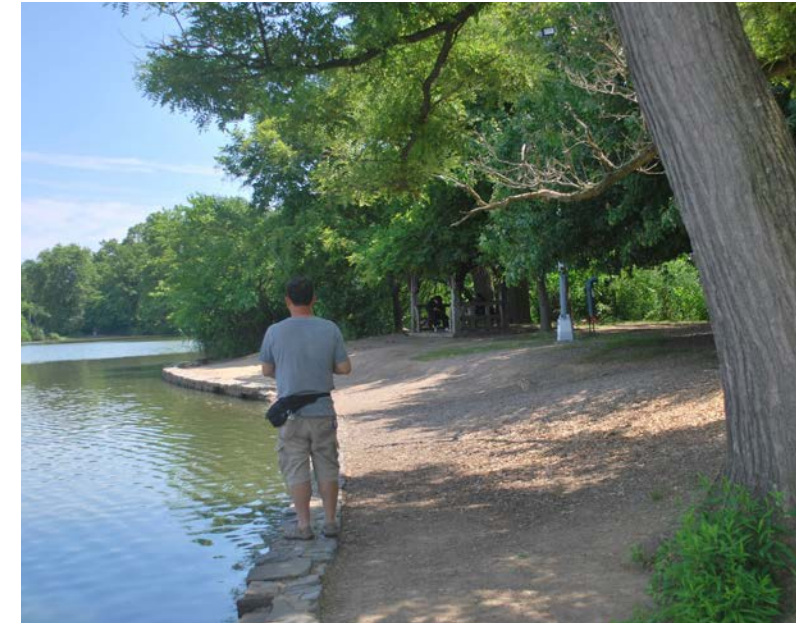
Erosion and compaction due to foot traffic
