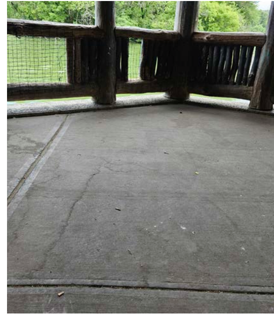
Concrete (at rustic shelter)
