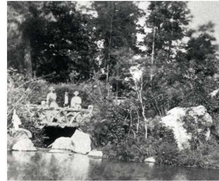
4. Fallkill Bridge (c. 1873) Historic bridge.
