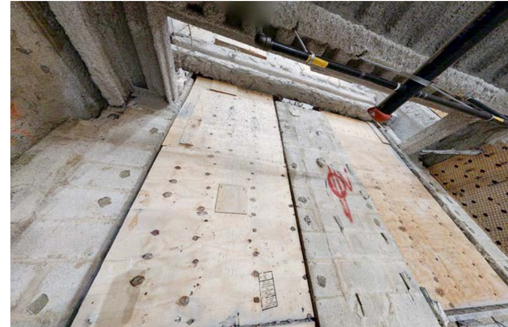
716 3rd floor - view looking up at 4th floor opening
