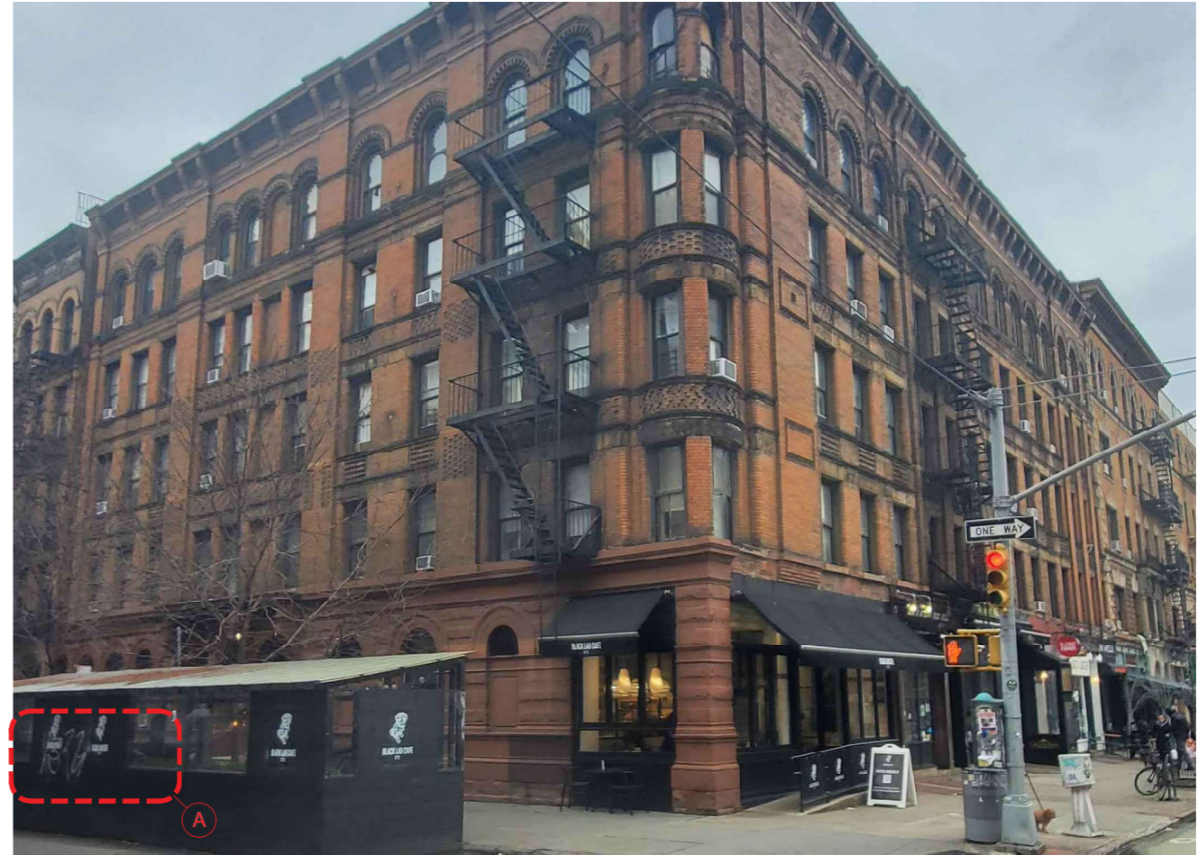
2 EXISTING CONDITIONS - CORNER OF 80TH & AMSTERDAM FACADE A-003 SCALE: NA
