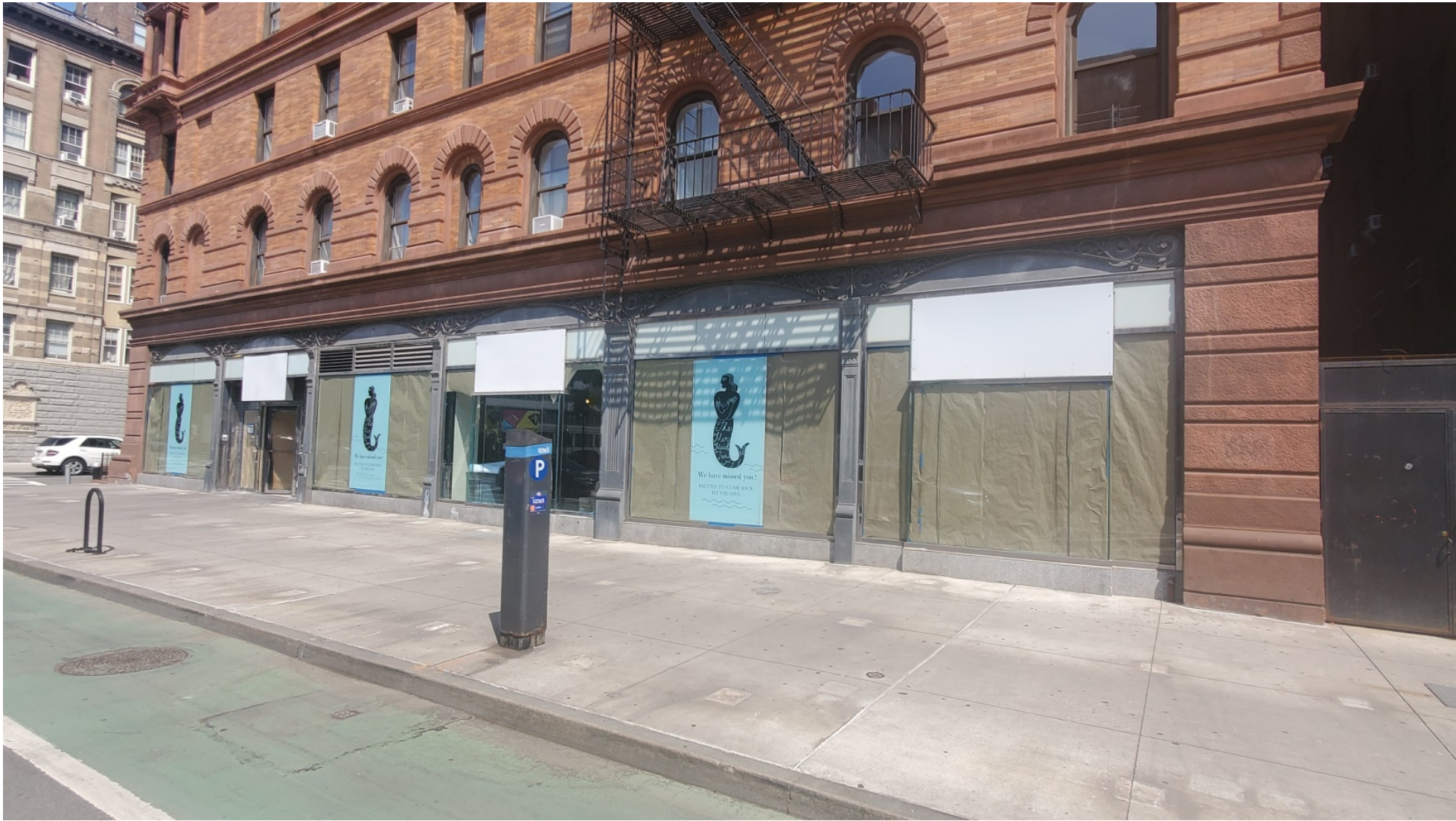
Note panels where former Chase signs were erected without permits
