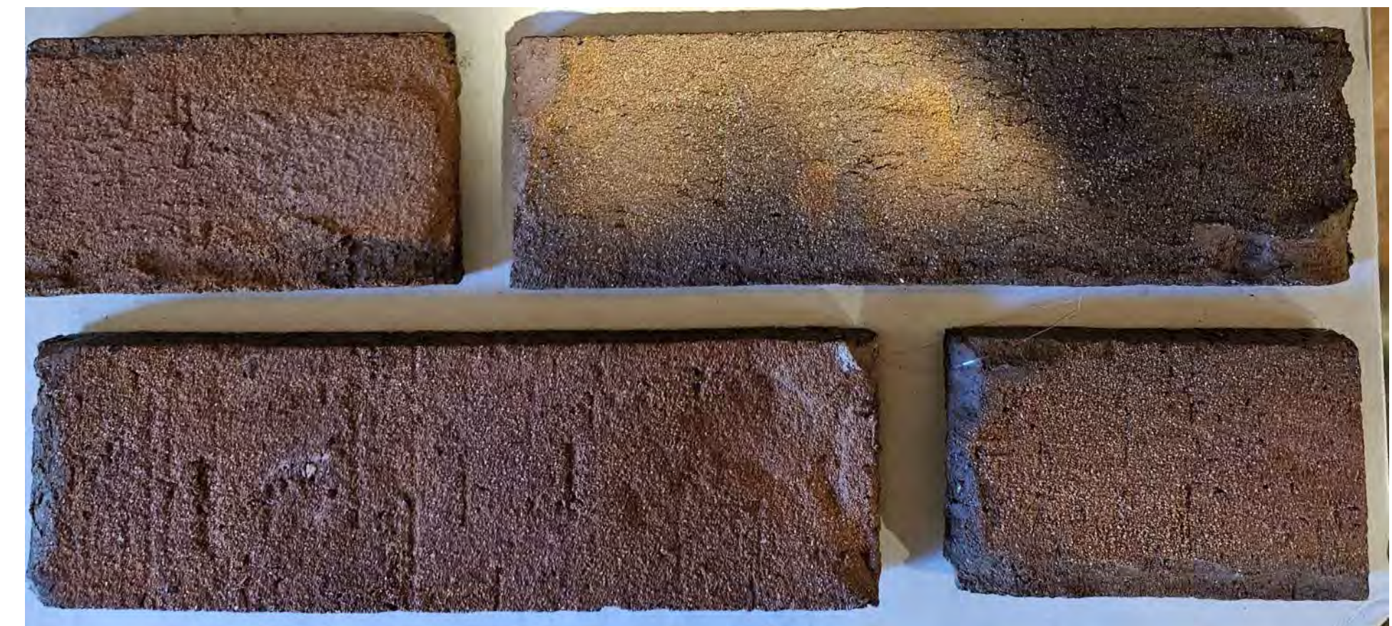
FULL BRICK AT REAR EXTENSION FACADE
