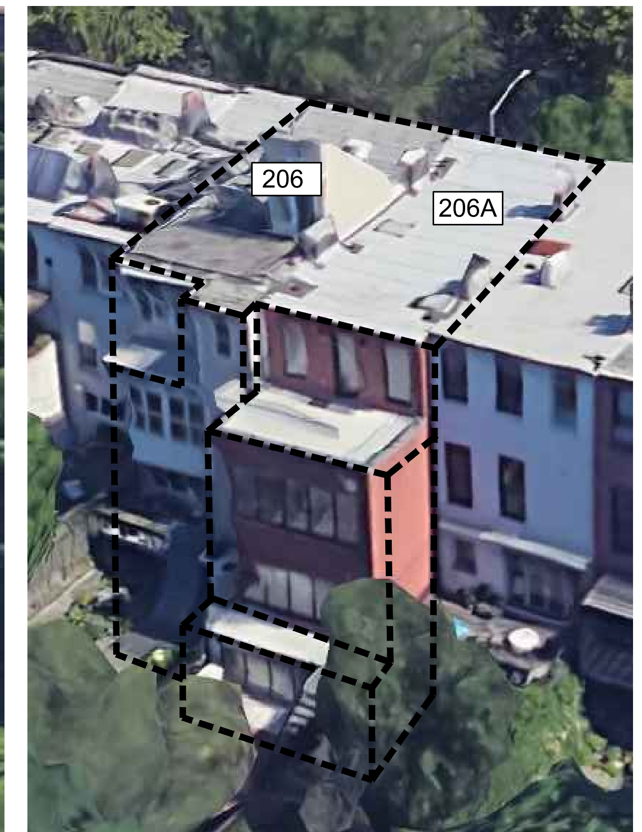
206 & 206A BERGEN STREET - ADDITION
