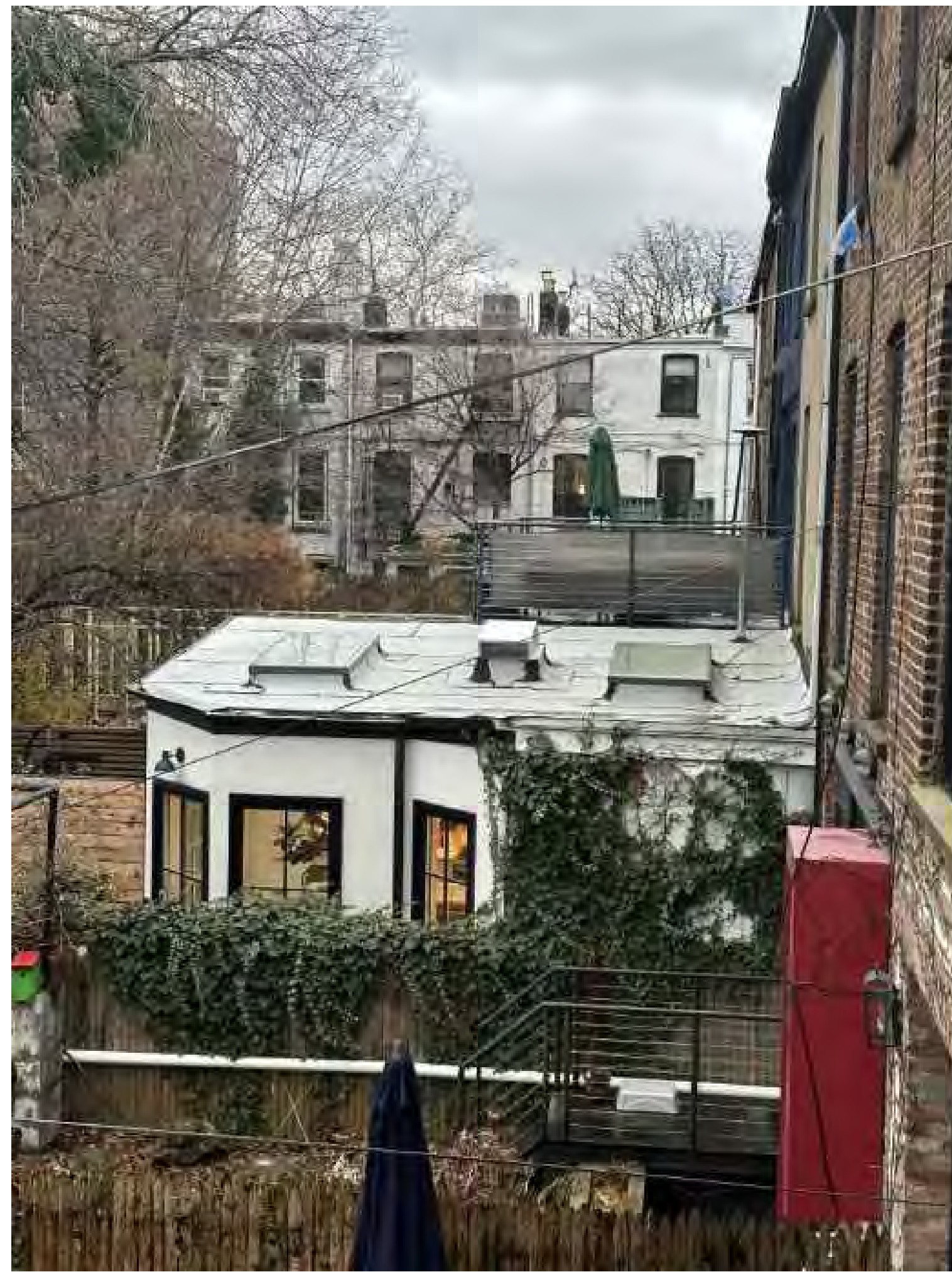
233 WYCKOFF ST - ELEVATED VIEW TO NEVINS ST SCALE: NTS
