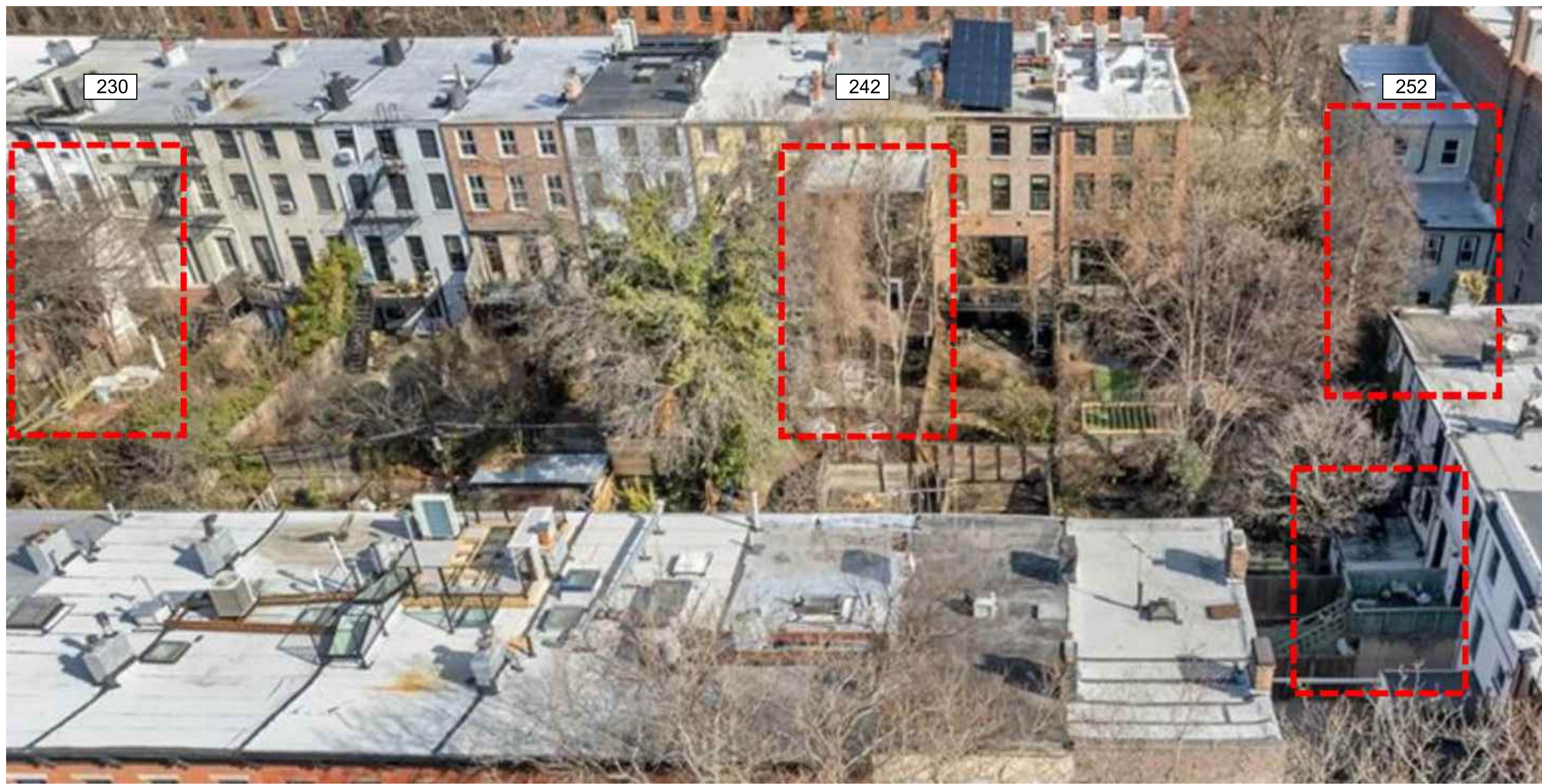
BERGEN STREET REAR YARD AERIAL PHOTO
