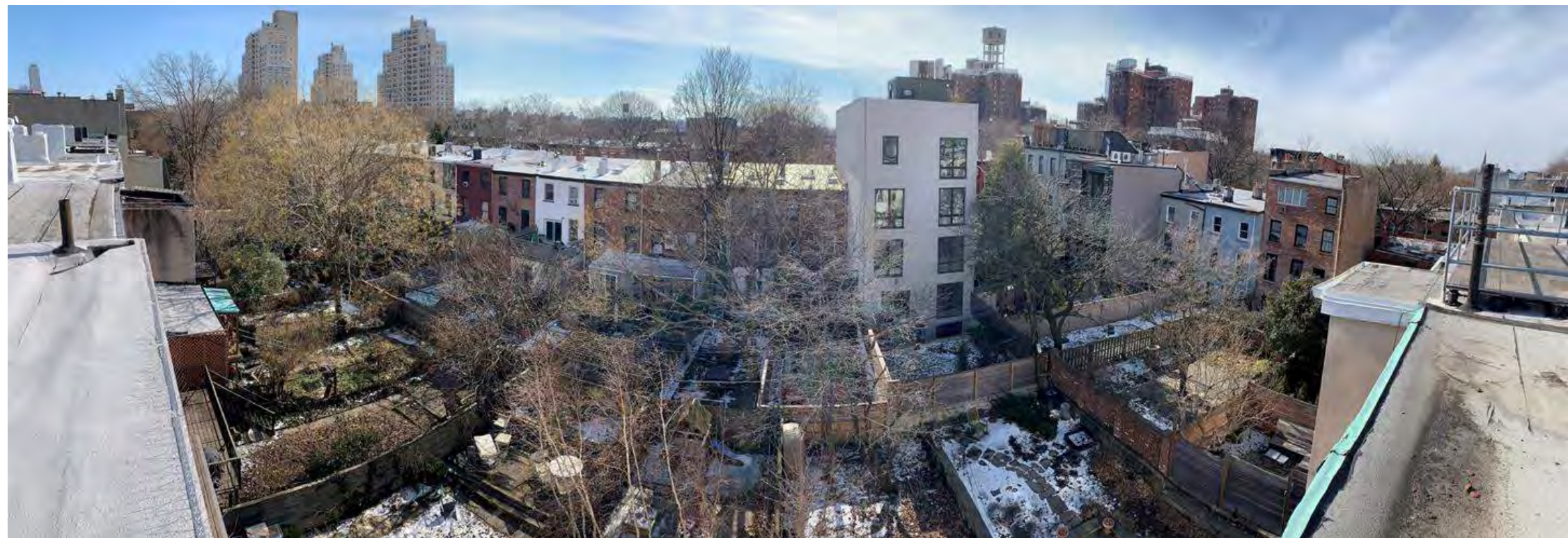
Existing Rear Yard view from rear grade level
