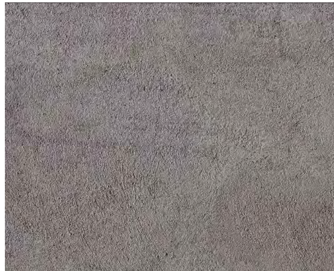
STUCCO FINISH AT SIDE OF EXTENSION
