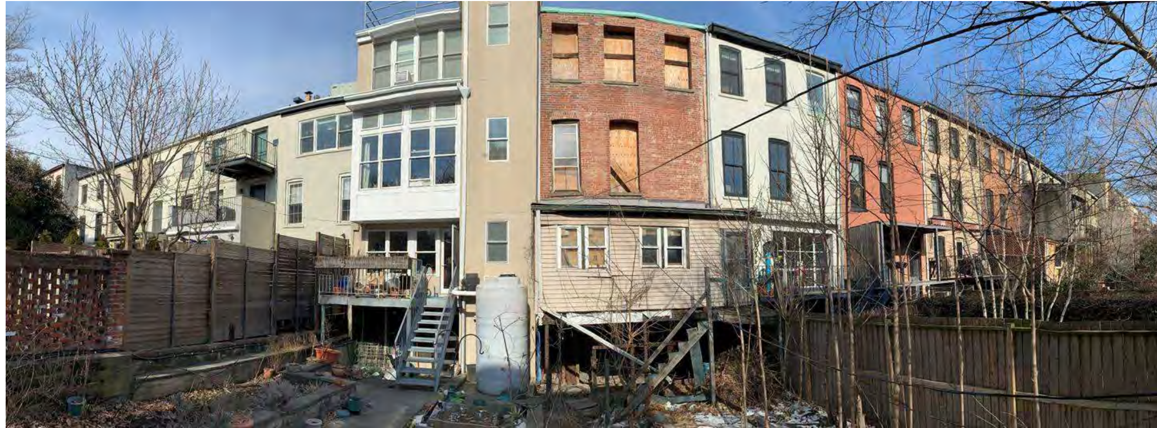
Existing Rear Yard view from rear grade level
