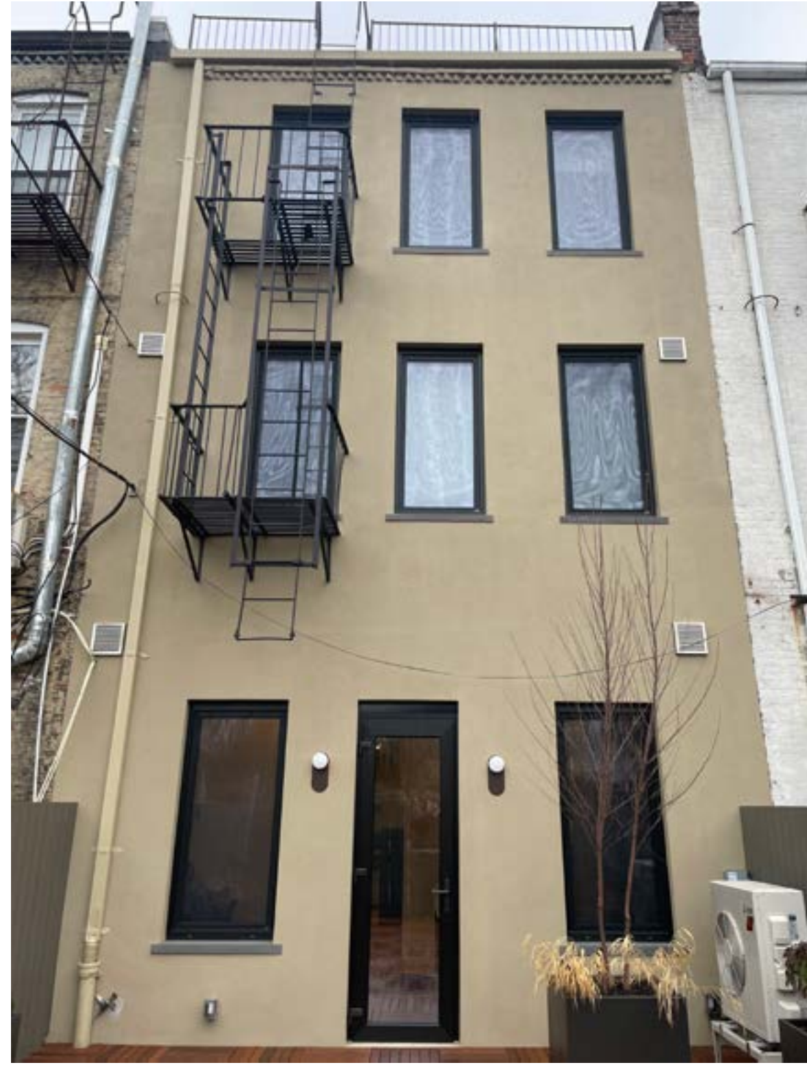
2023 Existing Condition Rear Facade
