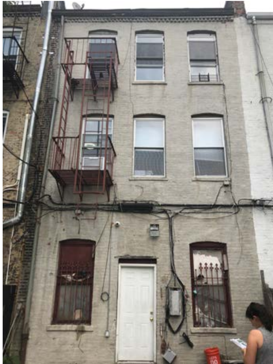
2020 Existing Condition Rear Facade - Parge Coat
