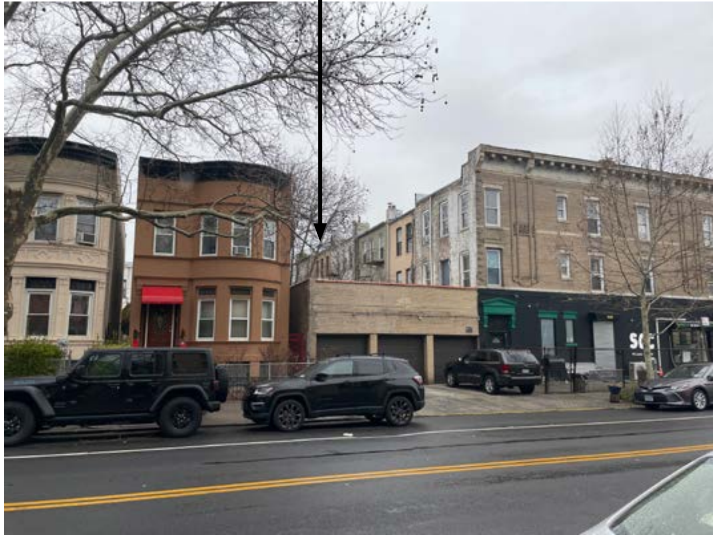
View of 418 Rogers Rear Facade from Lefferts Avenue Minimal Visibility
