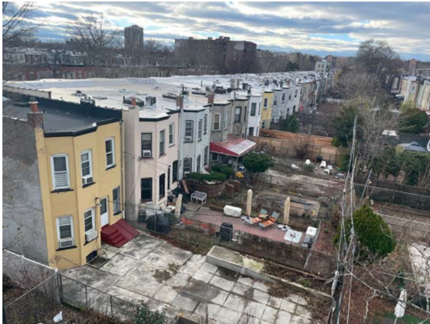
View of Rear Facades of Houses on Lefferts Avenue Taken from 418 Rogers Roof
