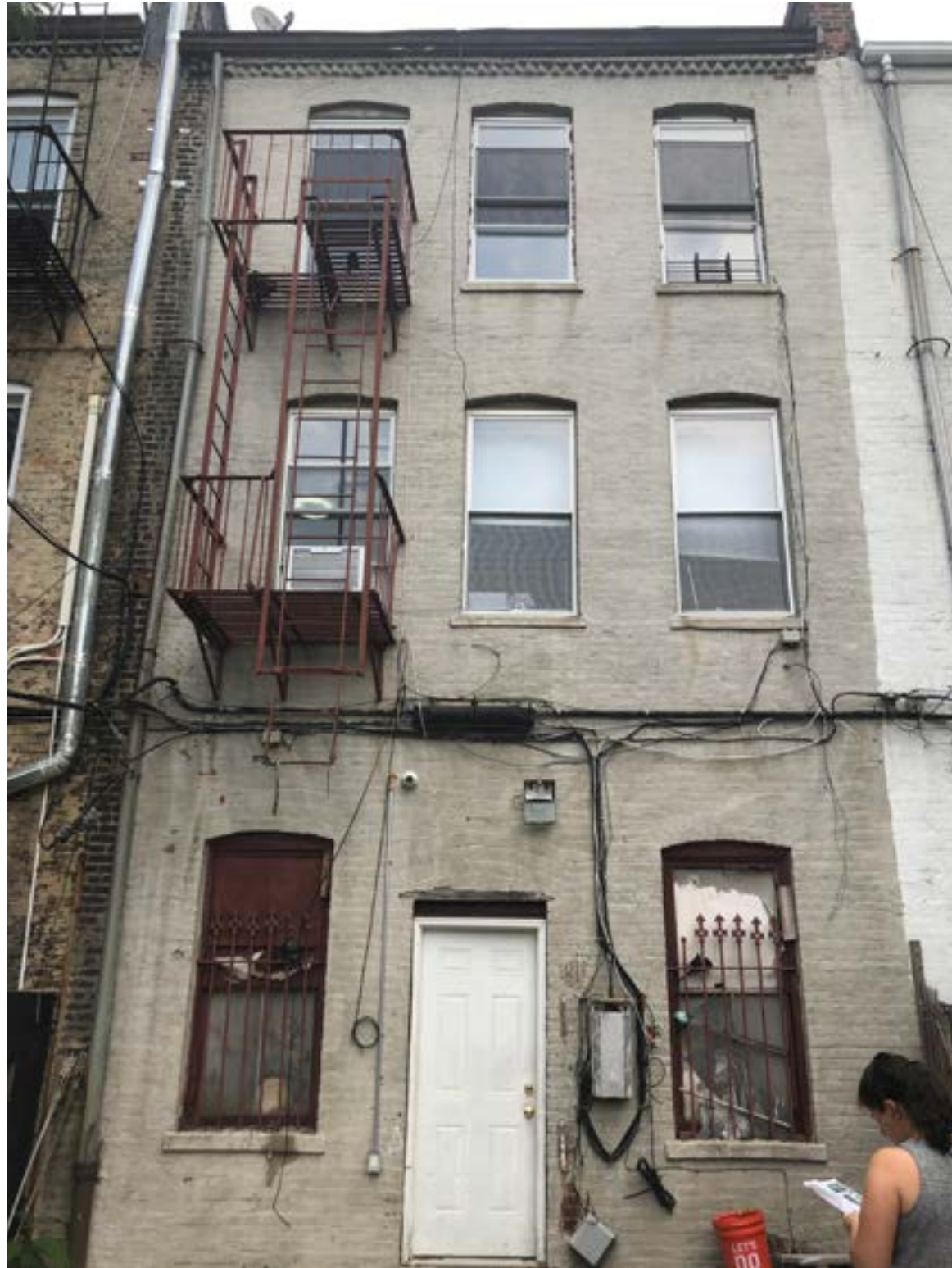
2020 Existing Condition Rear Facade
