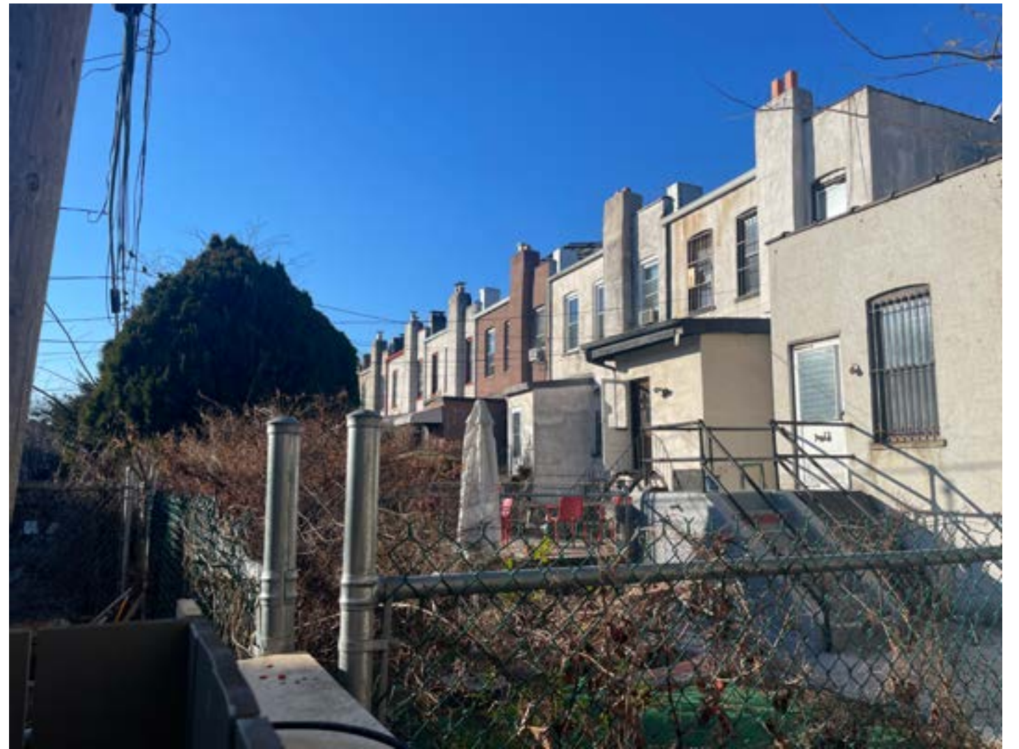
View of Rear Facades of Houses on Sterling St Taken from 418 Rogers Backyard
