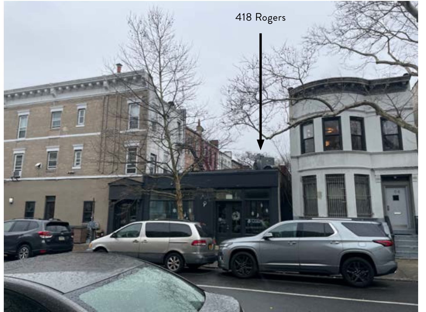
View of 418 Rogers Rear Facade from Sterling Street No Visibility
