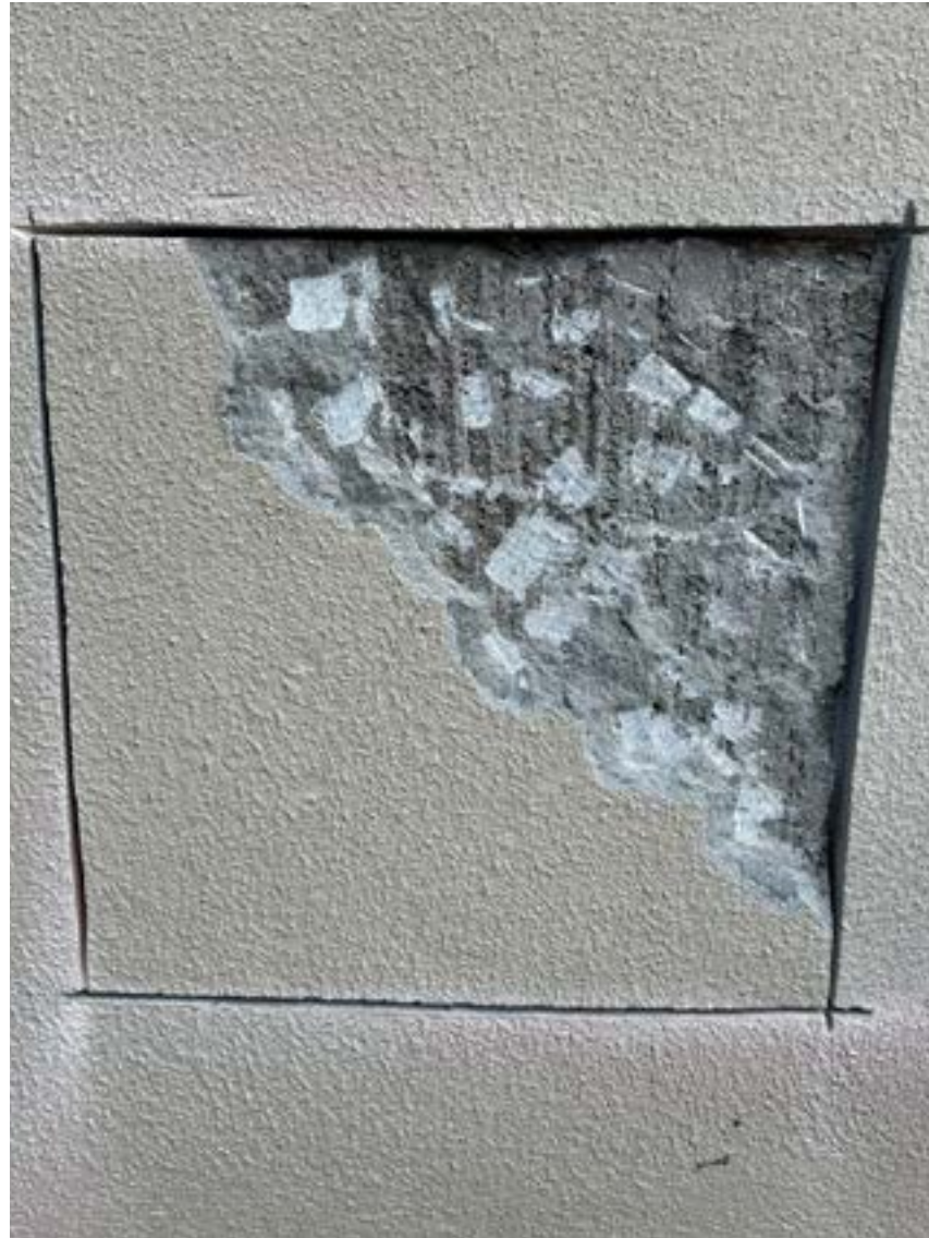
Removal of Parge Coat Using Chisel 12" x 12" Test Patch
