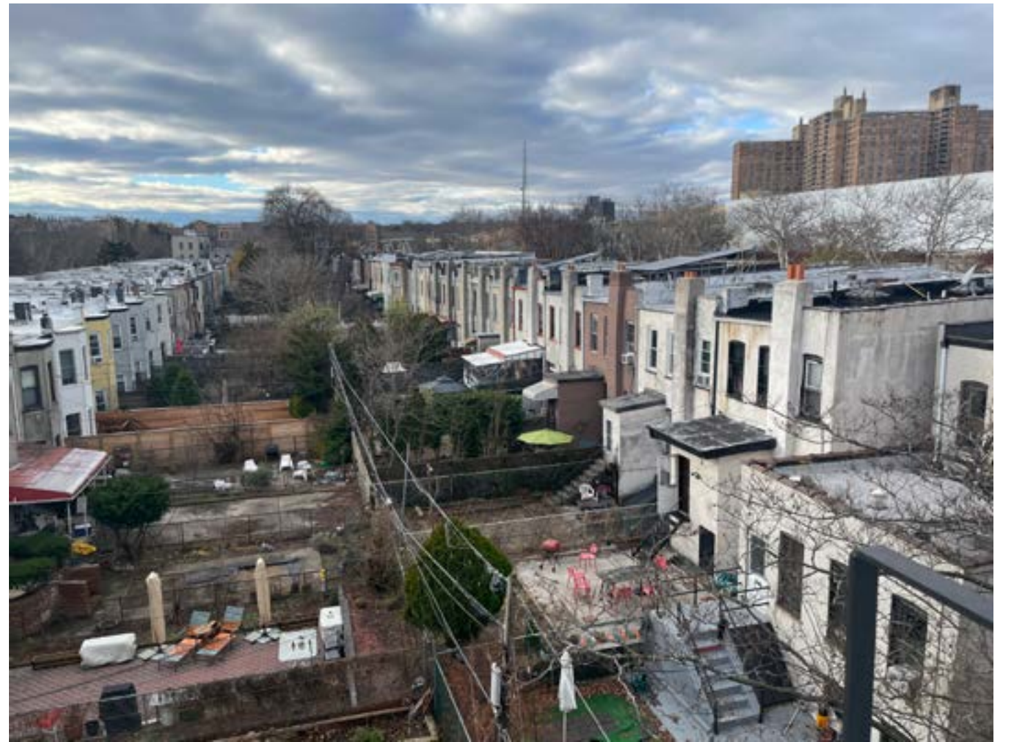
View of Rear Facades of Houses on Sterling St Taken from 418 Rogers Roof
