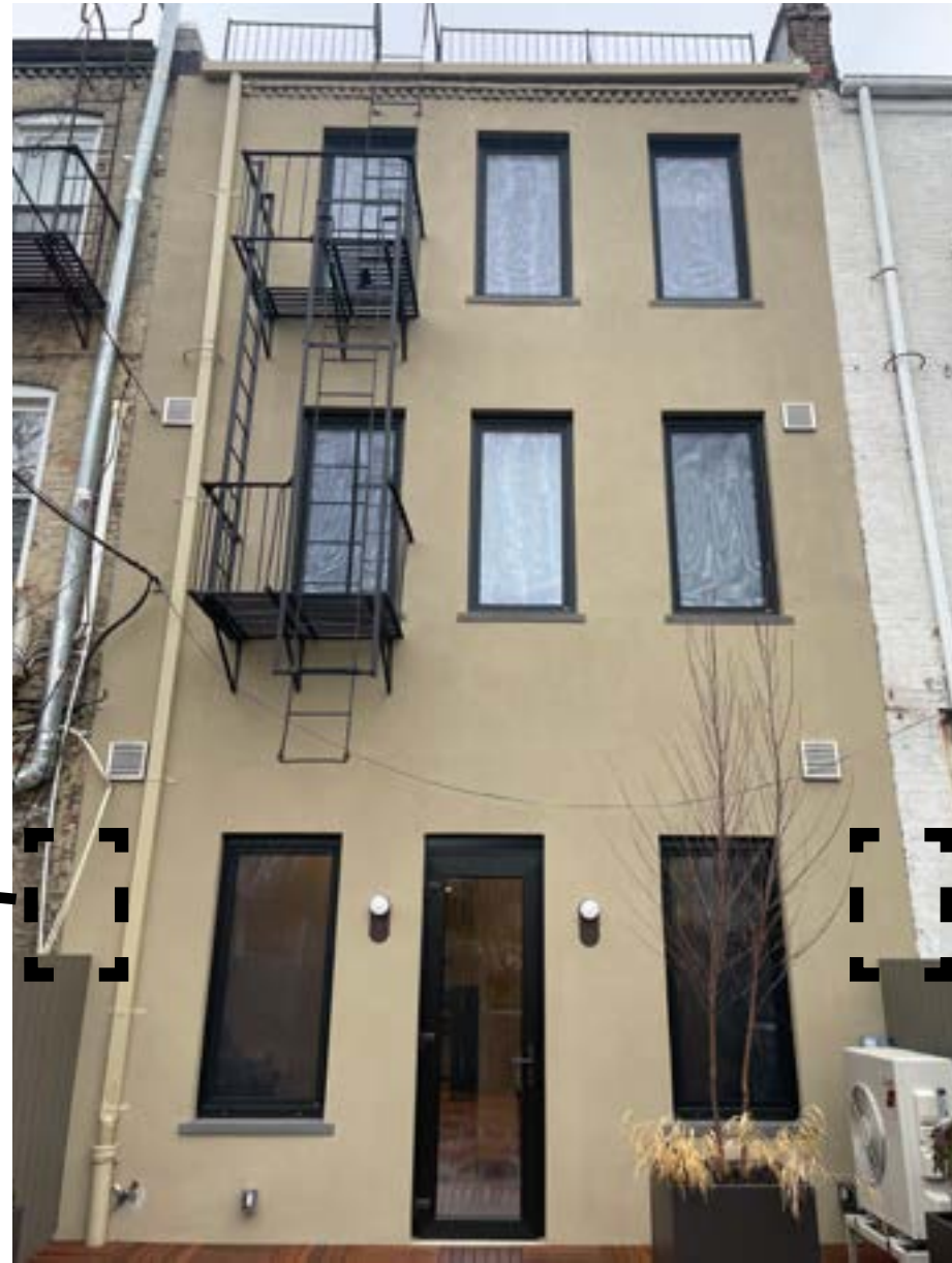
2023 Existing Condition Rear Facade - Finished
