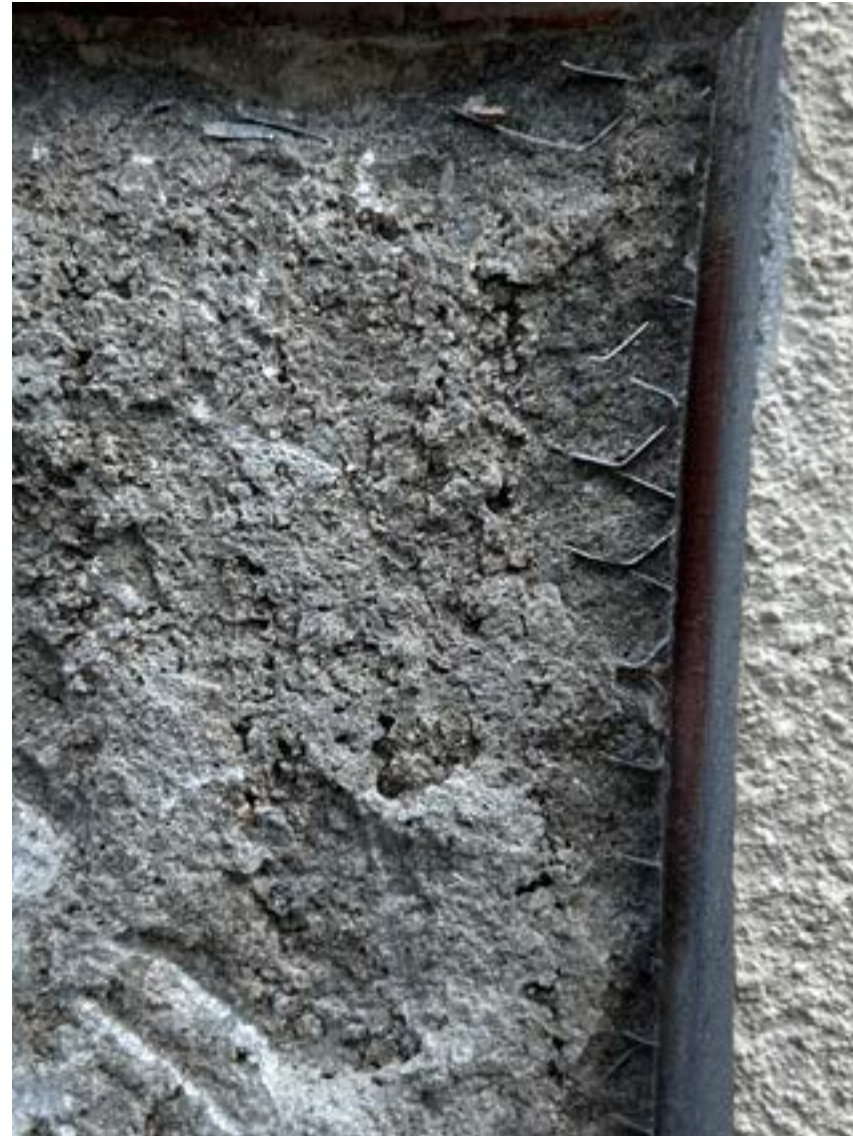
Removal of Stucco Until Steel Mesh Layer
