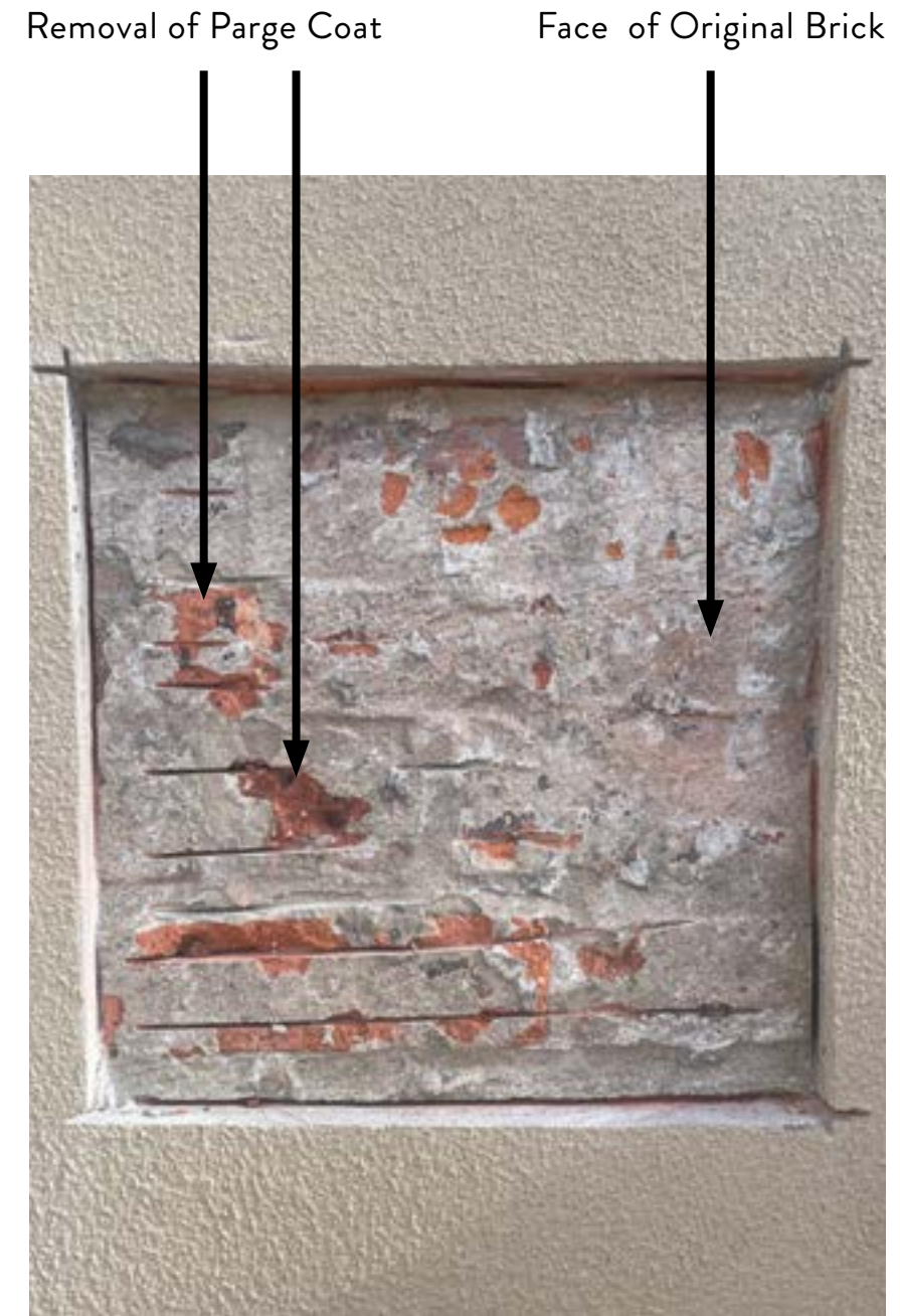
Removal of Existing Parge Coat on Brick
