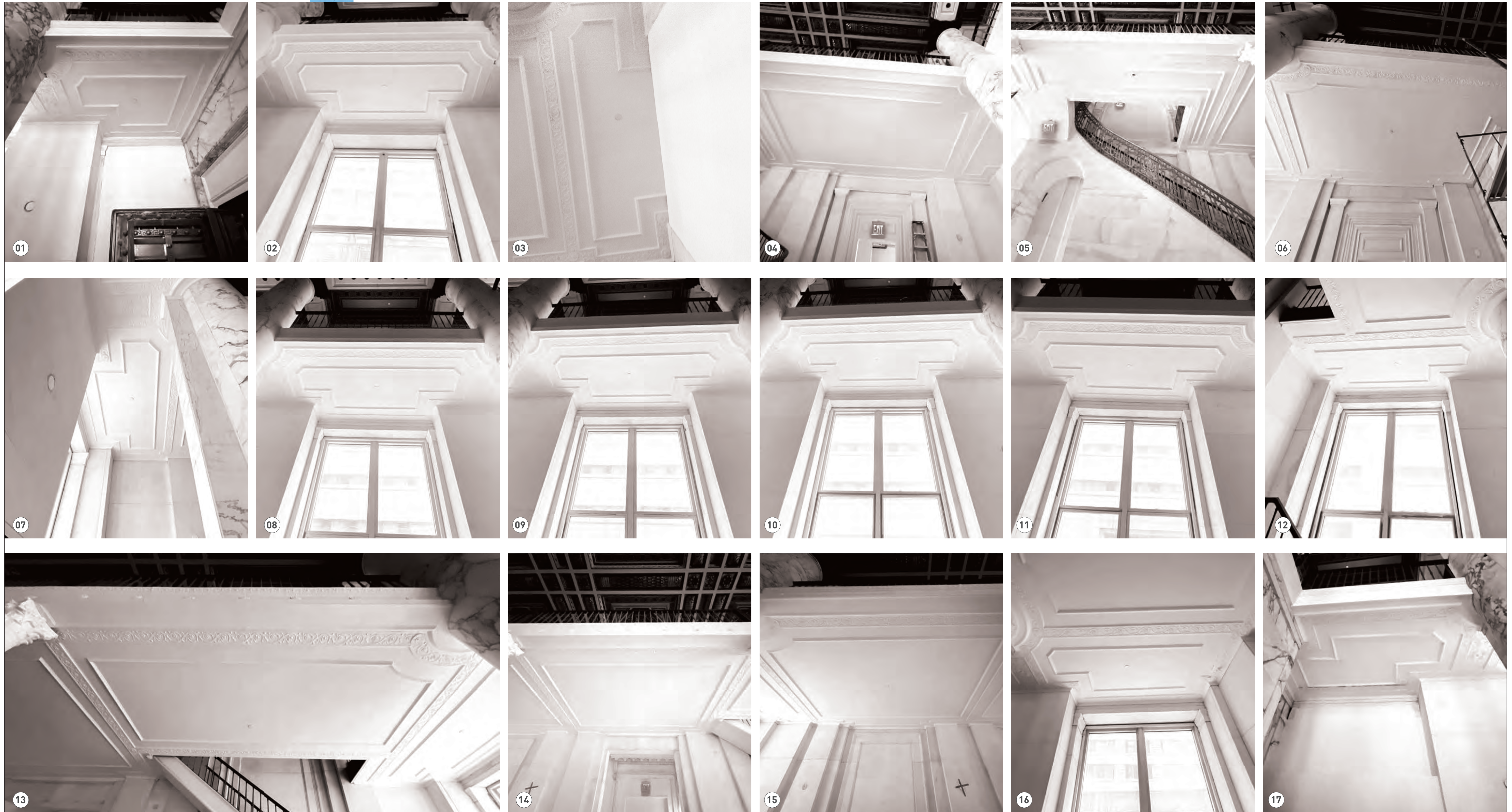
Existing Ceiling Mouldings
