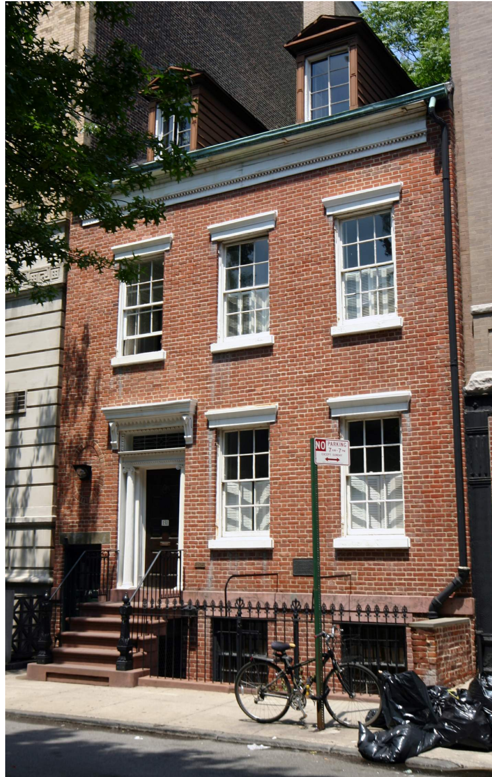
FRONT BUILDING - FRONT FACADE
