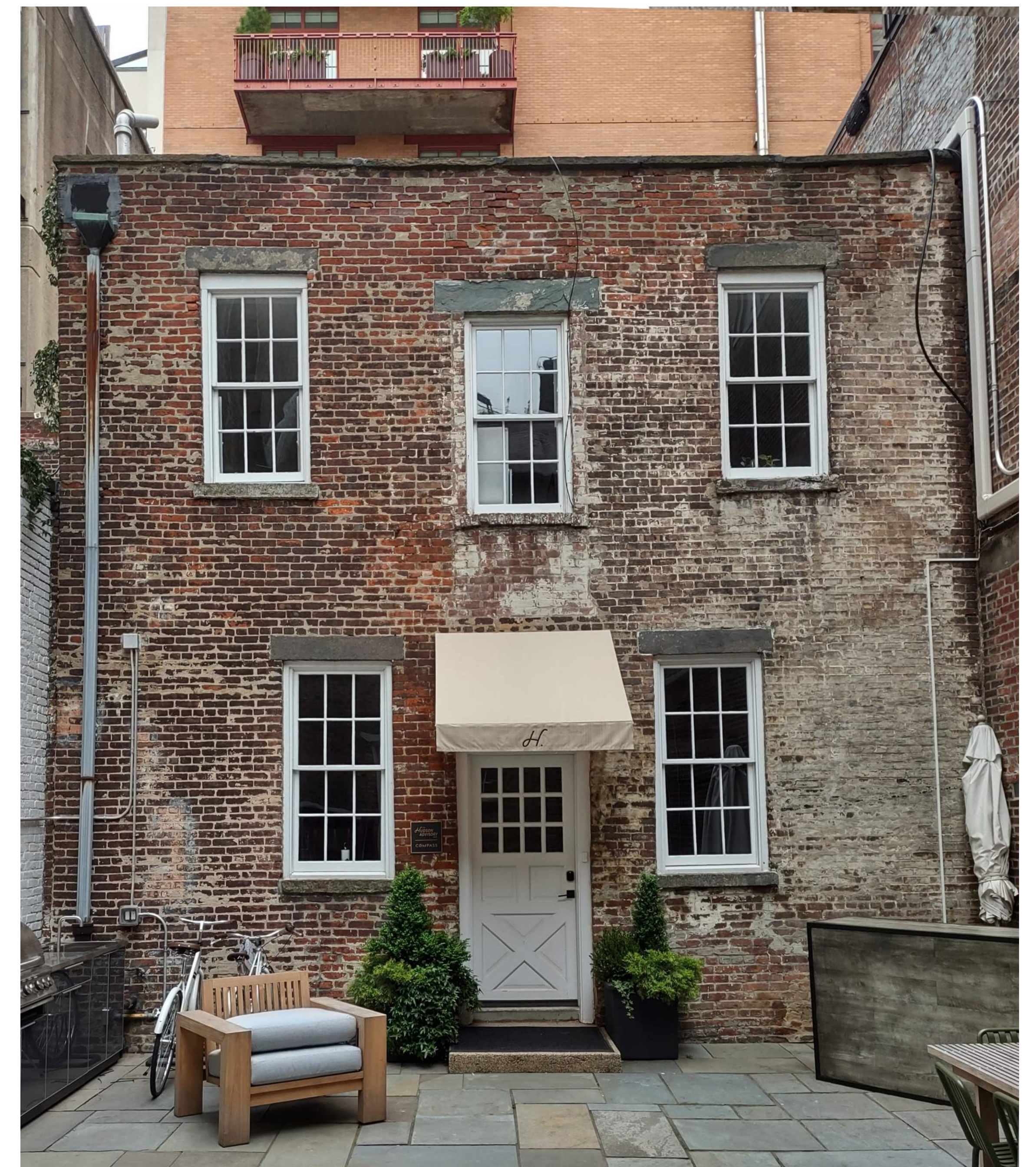
REAR BUILDING - FRONT FACADE
