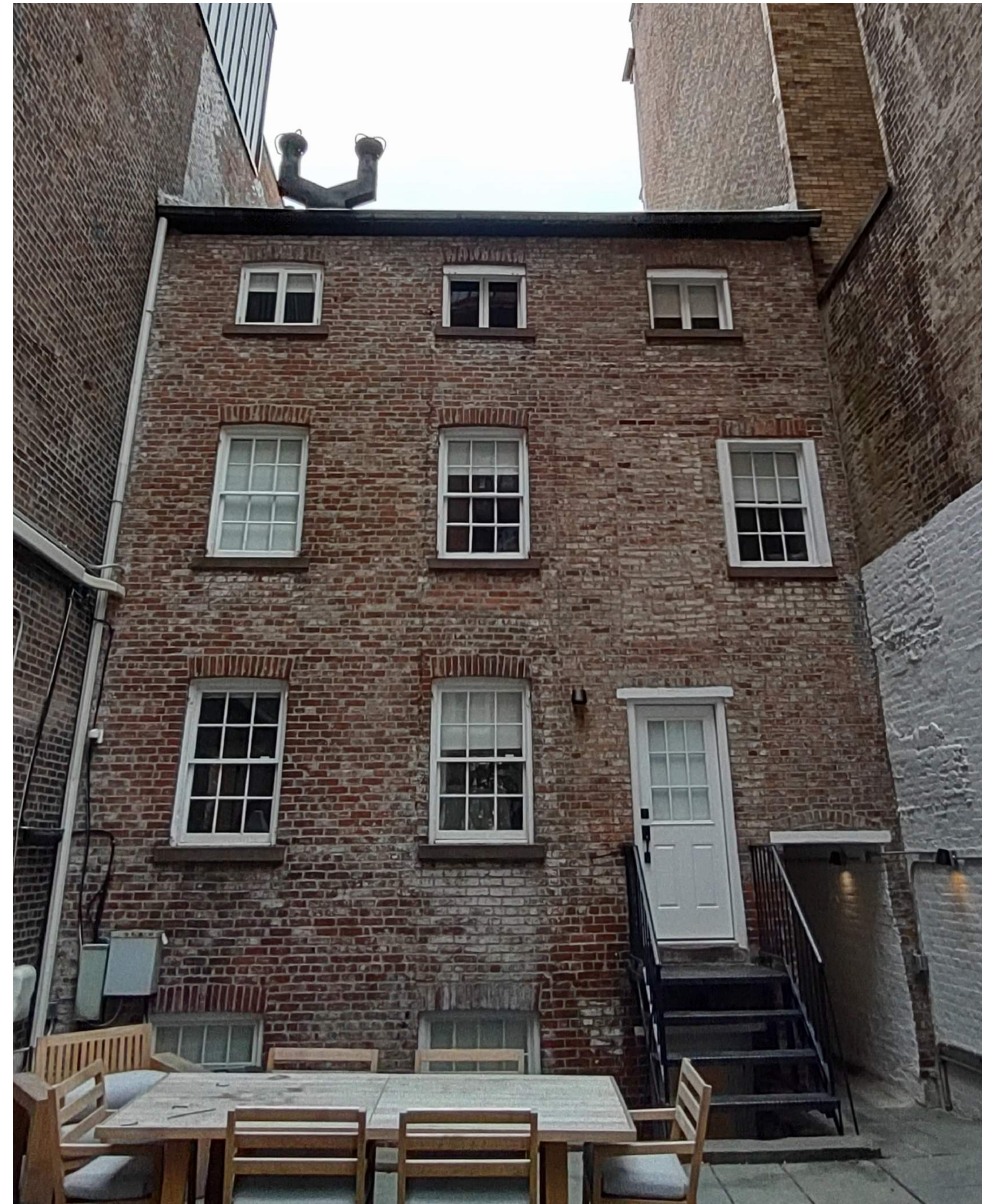
FRONT BUILDING - REAR FACADE
