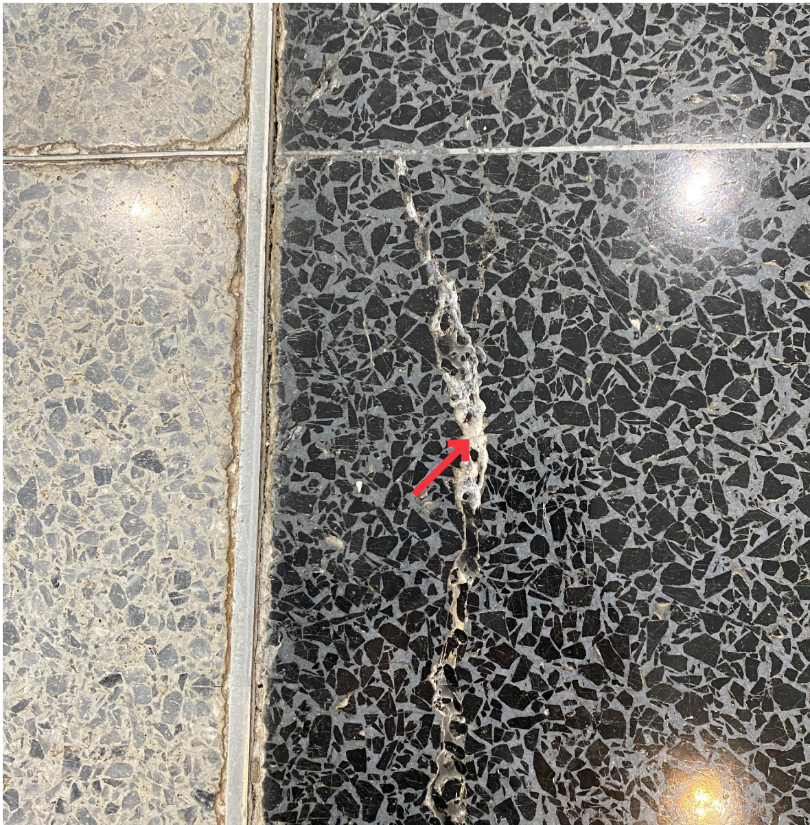
Cracking within Panels
