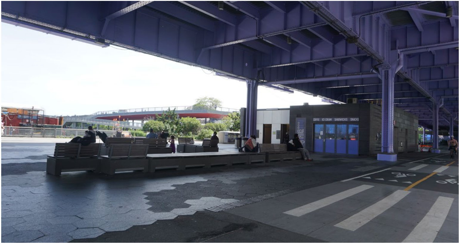
04 VIEW FROM SOUTH STREET
