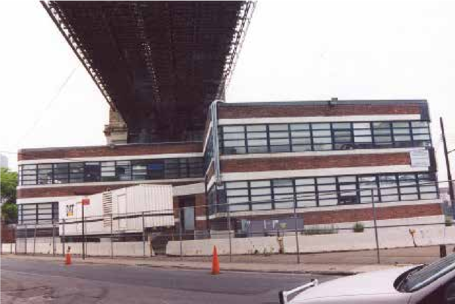
① View of Purchase Building from Water Street
