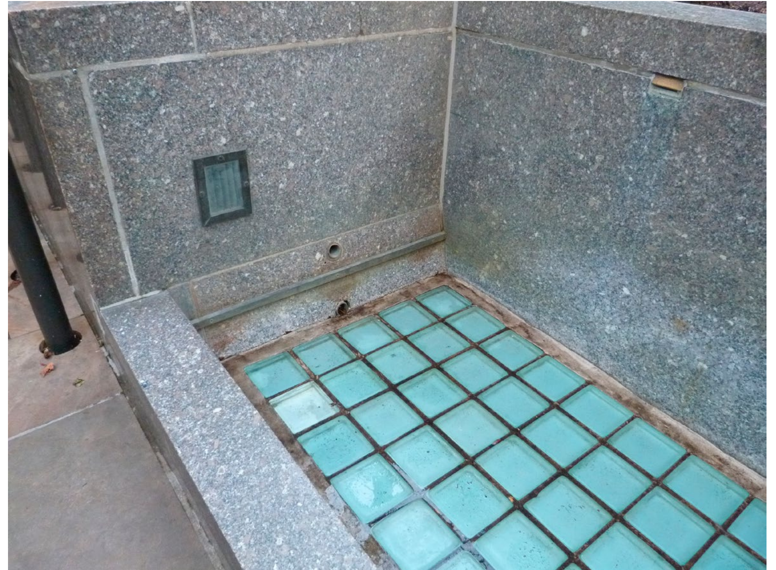
2 EXISTING CONDITION VIEW FACING SOUTH / EAST
