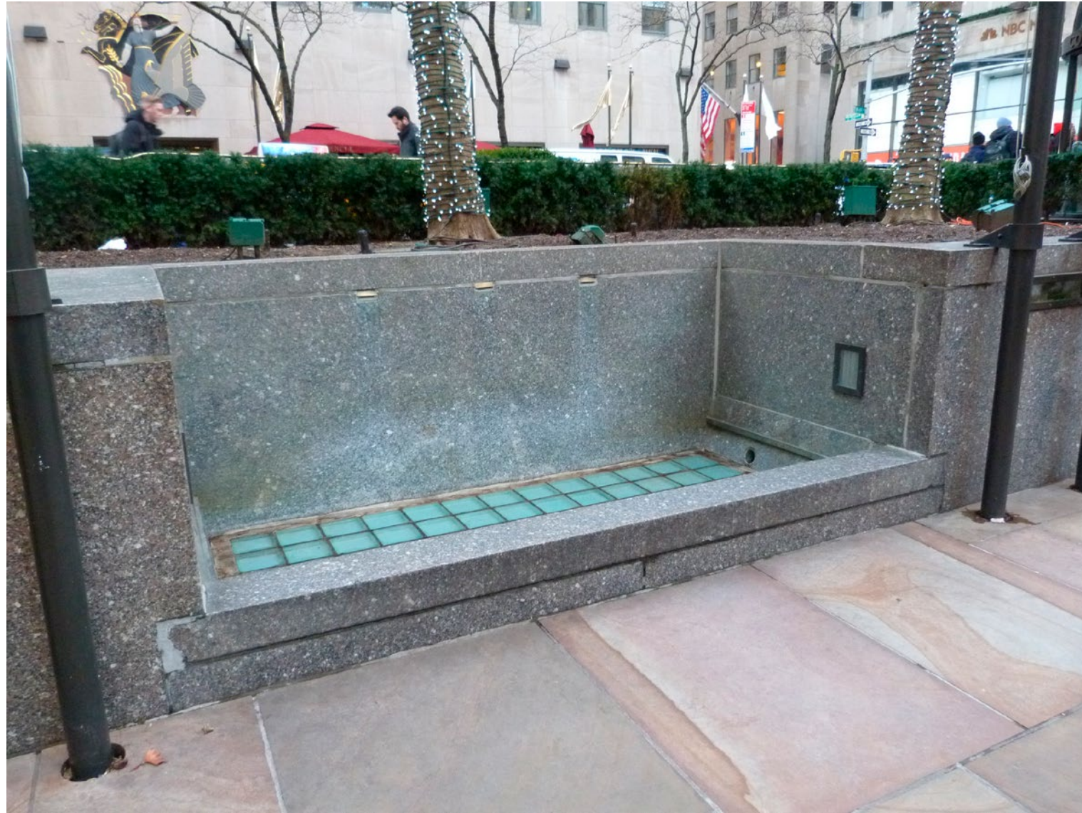
1 EXISTING CONDITION VIEW FACING SOUTH / WEST
