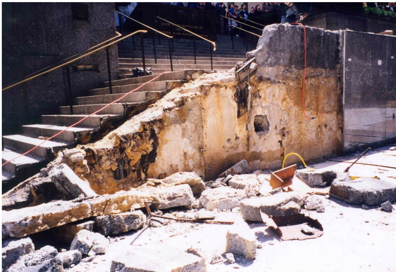
RINK RENOVATION (LOOKING SOUTH EAST), C.1998
