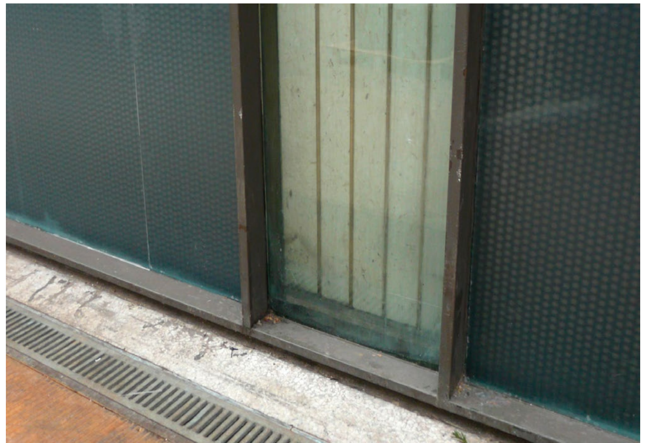
2 EXISTING CONDITIONS - PRESENT SUNKEN PLAZA - SOUTH ELEVATION DETAIL
