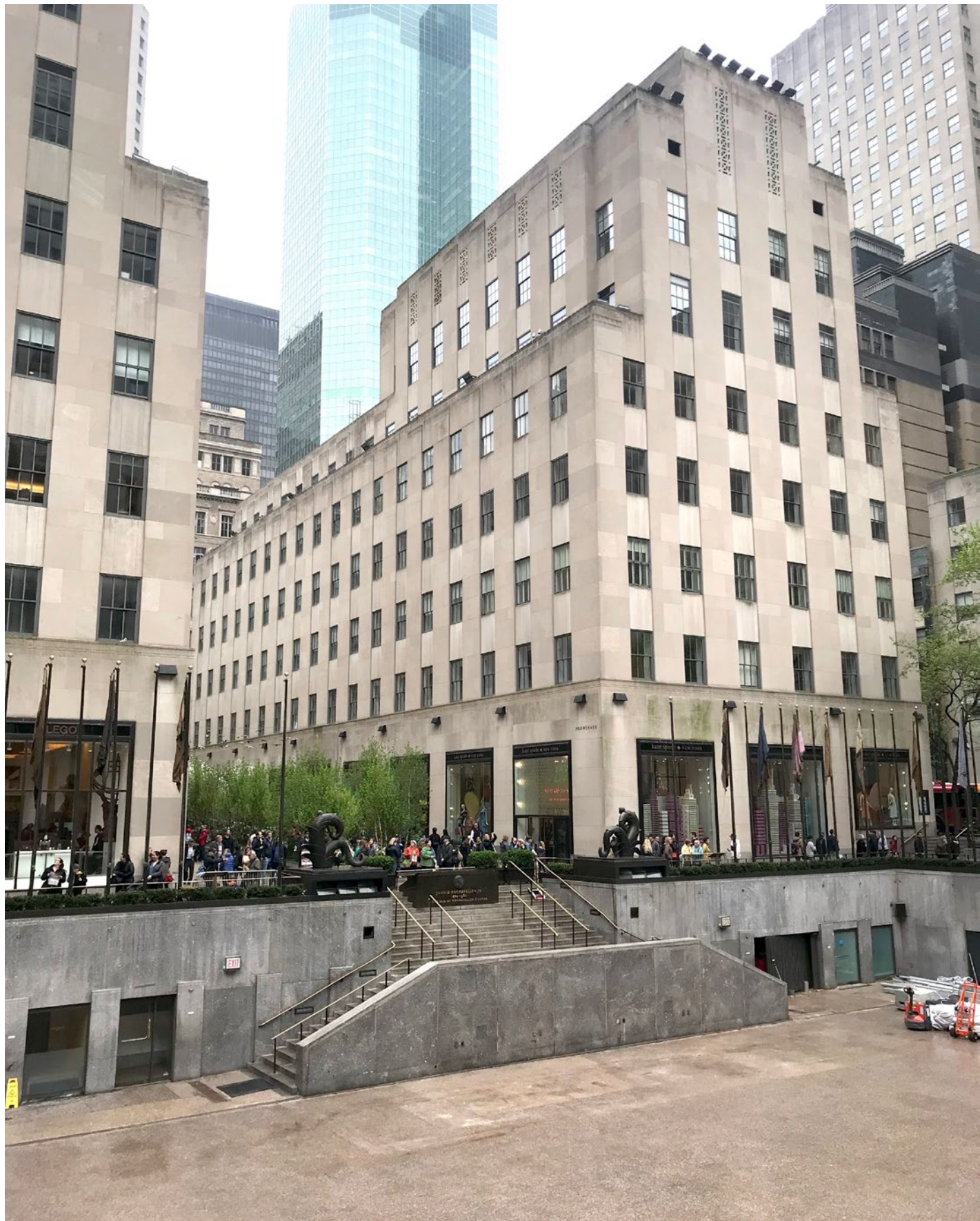
2 EXISTING CONDITION PRESENT - 2019
