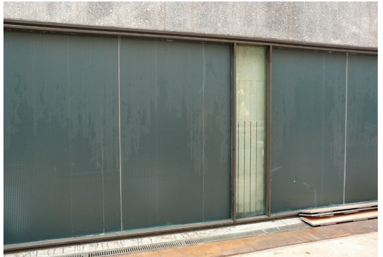
4 EXISTING CONDITIONS - PRESENT SUNKEN PLAZA - SOUTH ELEVATION DETAIL
