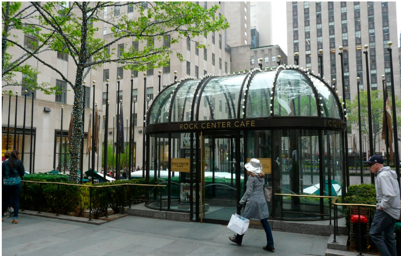
1 EXISTING CONDITIONS - PRESENT NORTH/SOUTH GARDENS, VIEW LOOKING SOUTH
