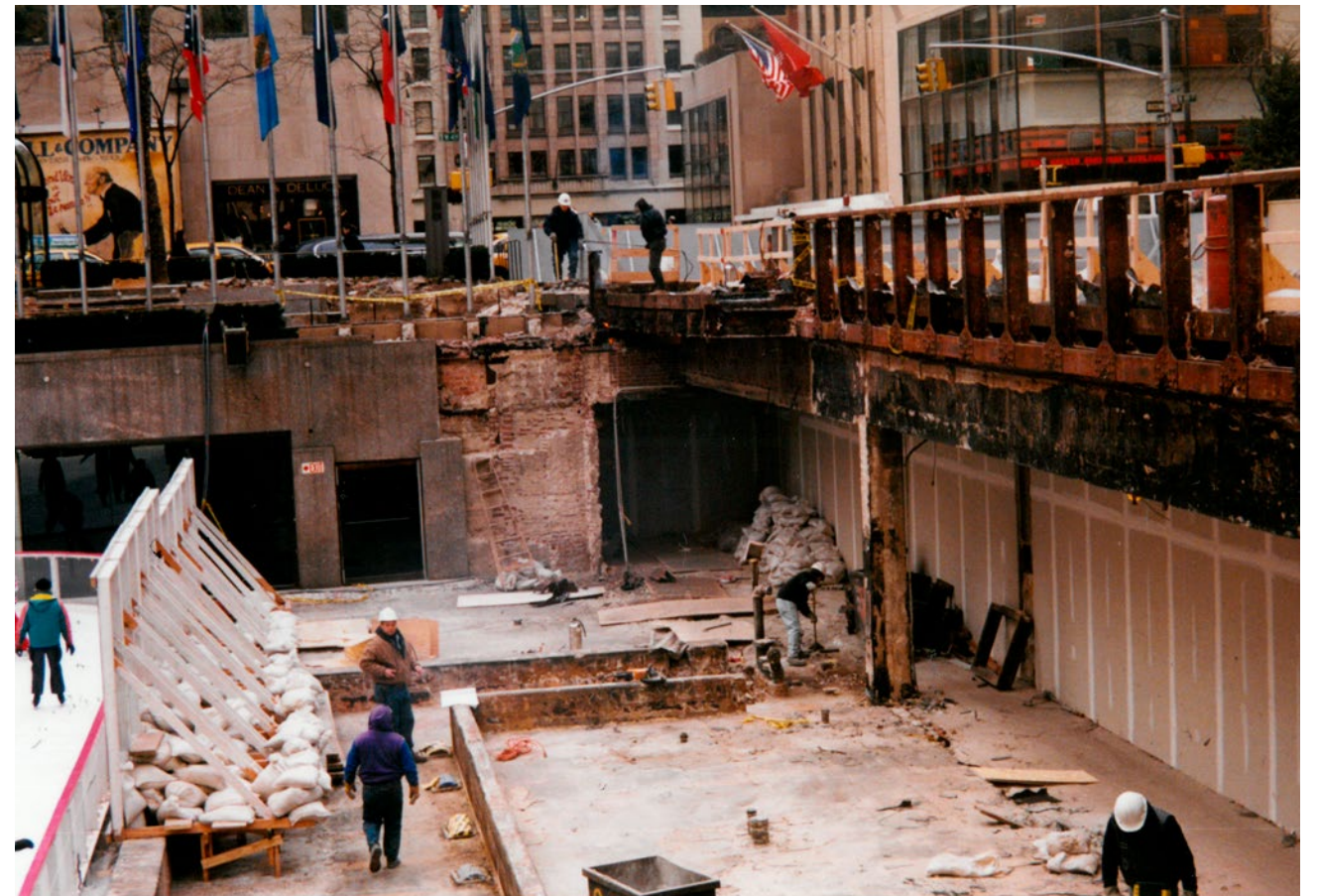
RINK RENOVATION (LOOKING SOUTH WEST), C.1998
