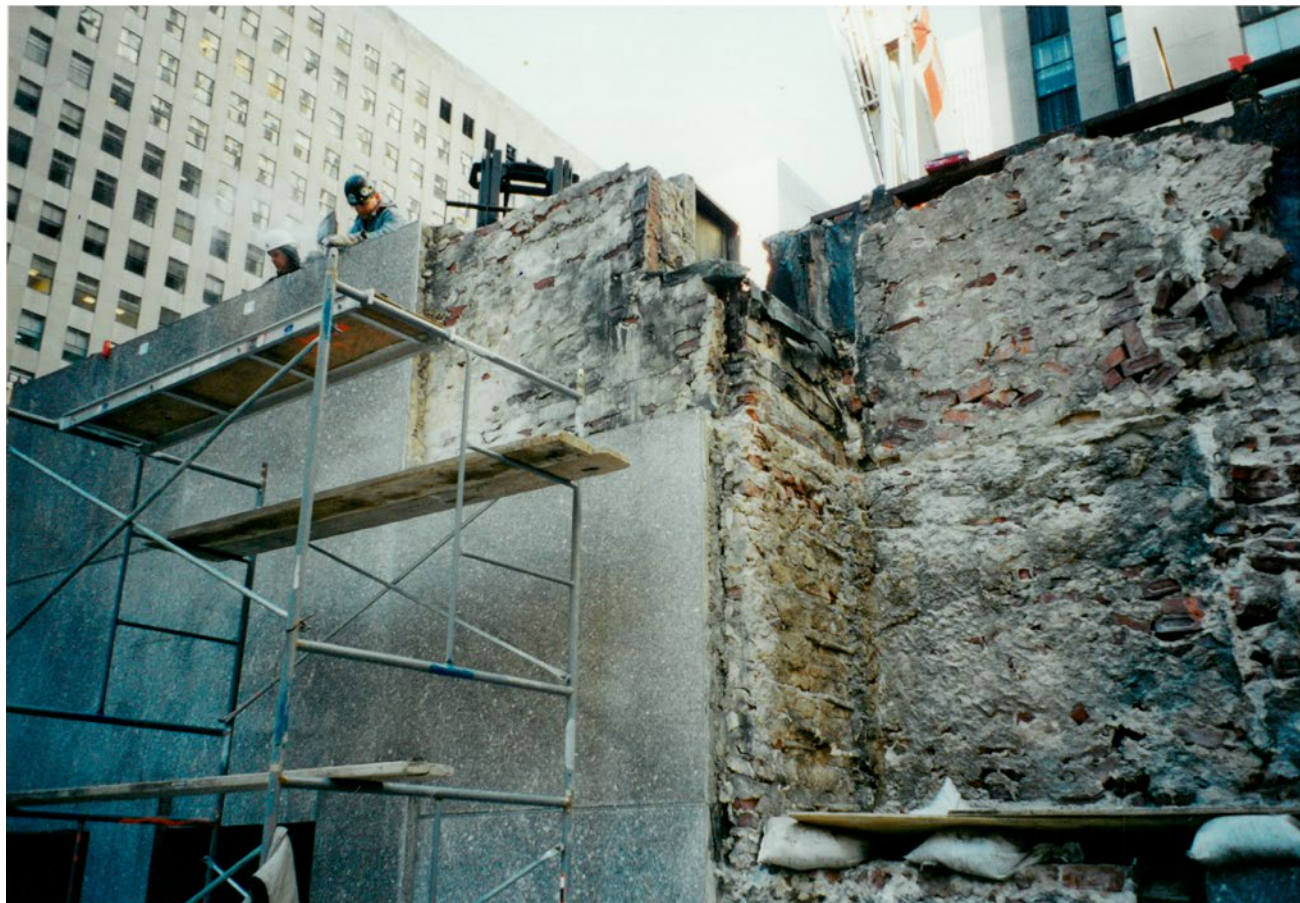
RINK RENOVATION (LOOKING WEST), C.1998
