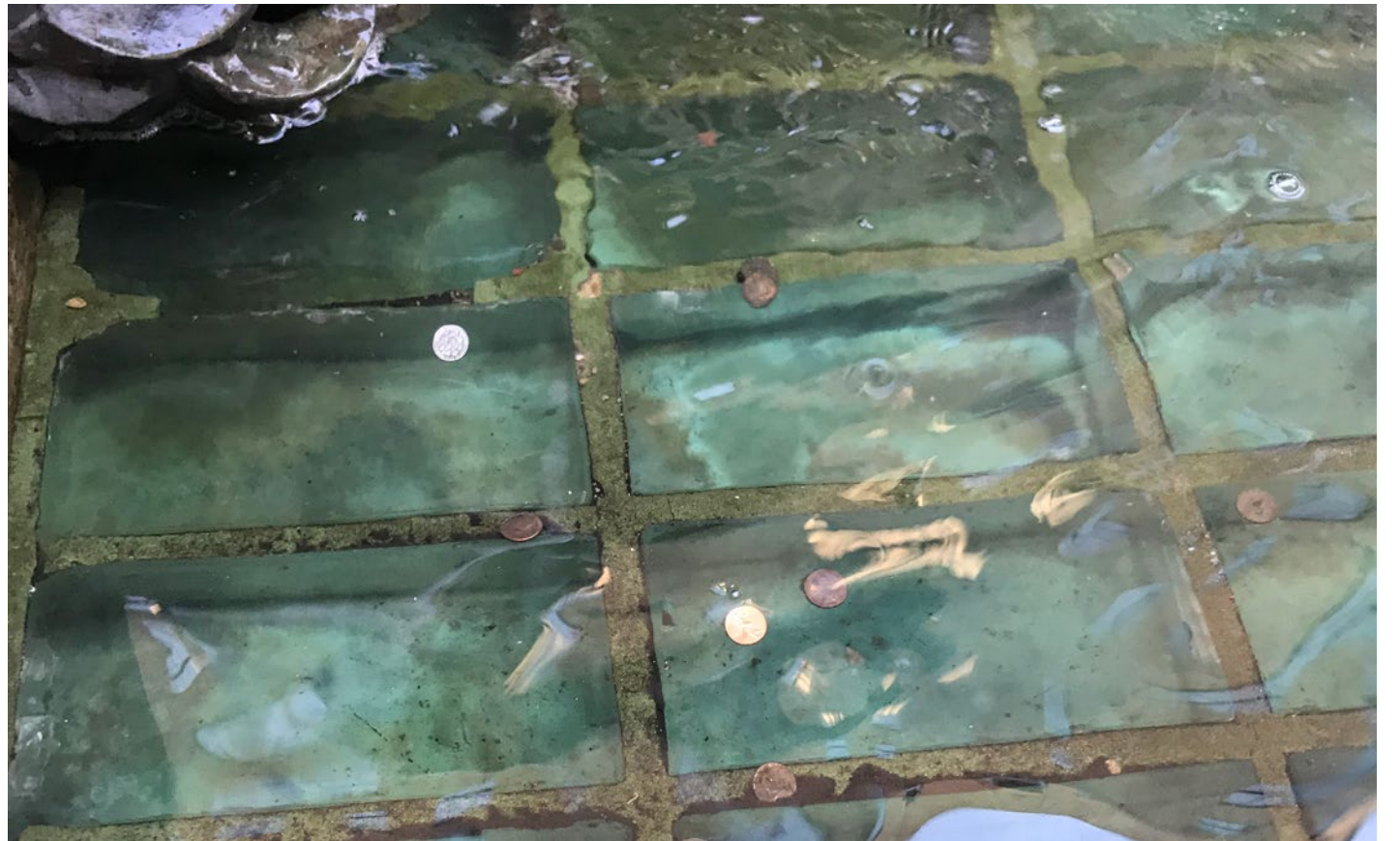
2 EXISTING CONDITIONS DETAIL VIEWS OF FOUNTAIN POOLS
