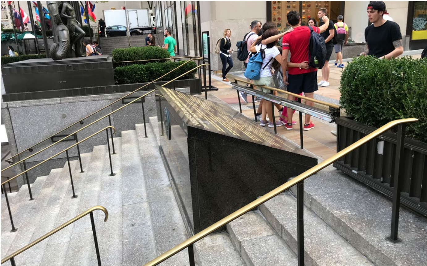
CREDO RELOCATION - EXISTING PHOTOS
