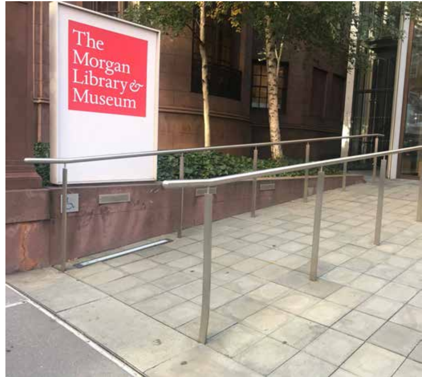
REFERENCE IMAGE EXISTING RAILING AT EXPANSION BUILDING RAMP, MADISON AVENUE
