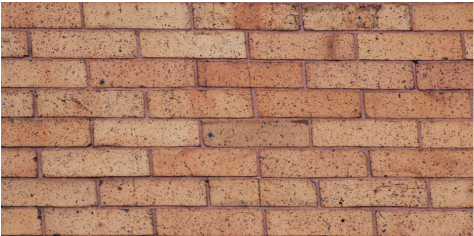
Englehardt Building: Atlantic Avenue & Schenck Avenue Existing brick and mortar. All replacement brick and mortar to match.
