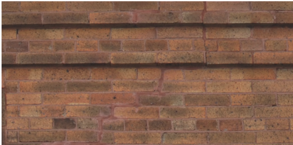
Strack Building: Barbey Street & Atlantic Avenue Existing ironspot brick and mortar. All replacement brick and mortar to match.
