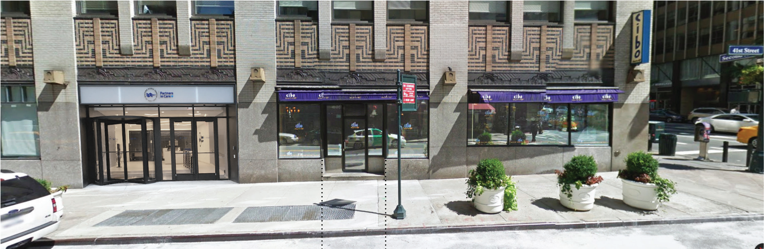
Existing 41st Street entrance showing slope of sidewalk and approximately 7” single step into the space.
