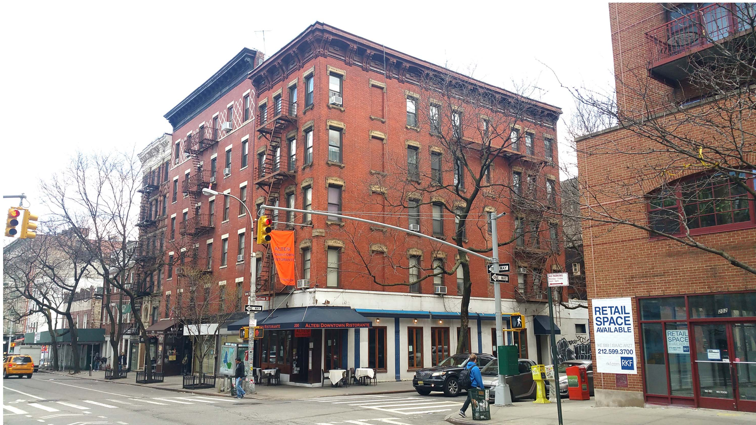
VIEW OF 196 & 198 SPRING STREET FROM THE NORTHWEST CORNER OF SPRING AND SULLIVAN STREETS
