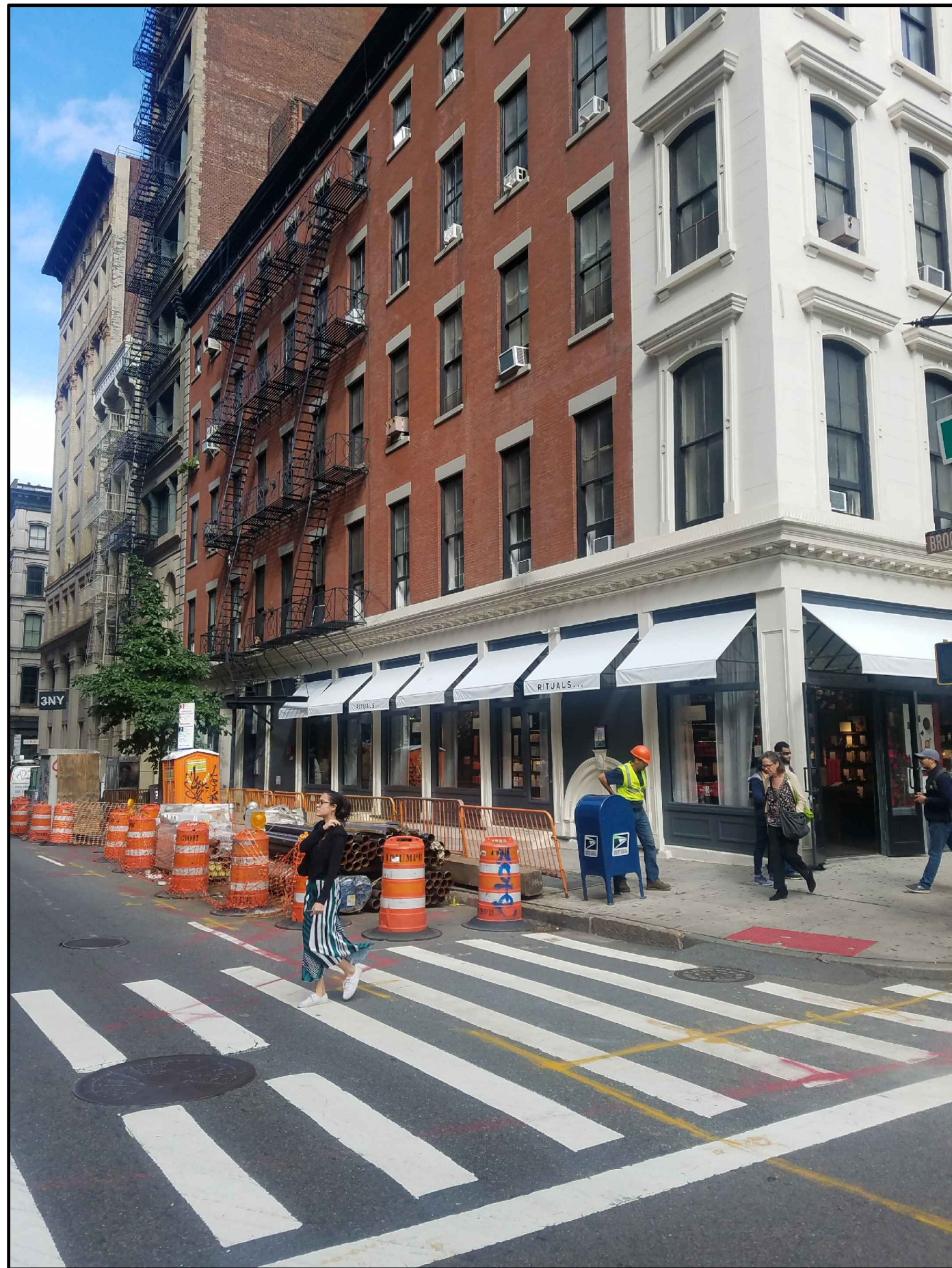
3 PHOTO - NORTH SIDE OF BROOME STREET NTS
