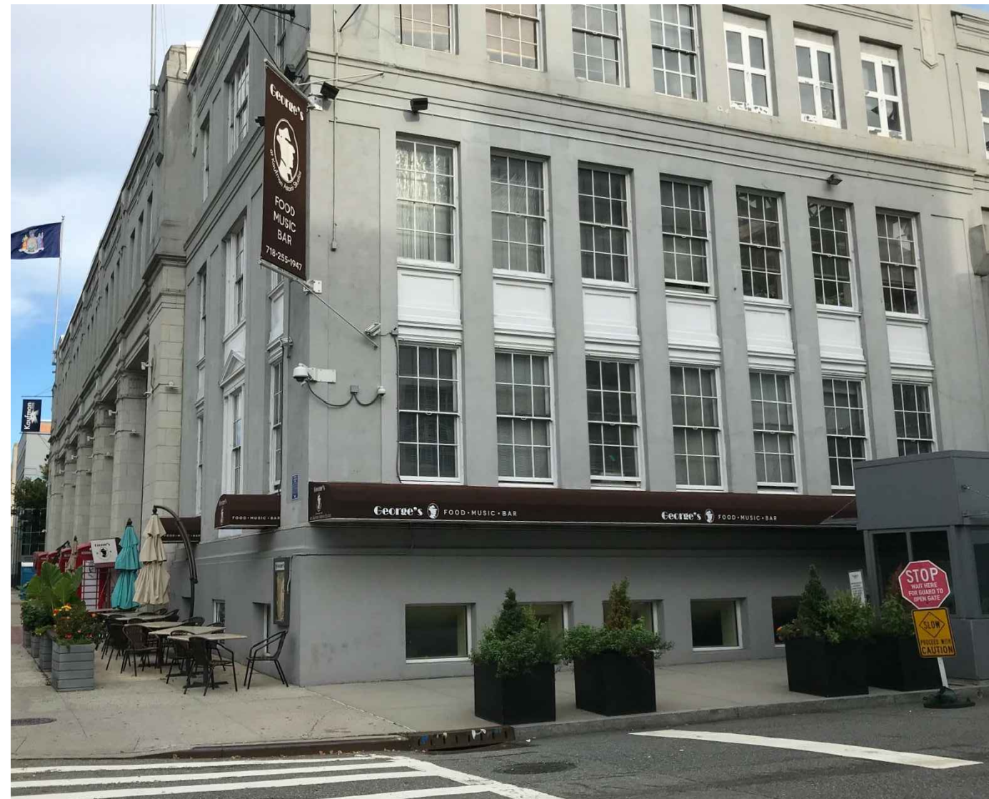
View of awnings from the corner of 36th Street & 35th Avenue
