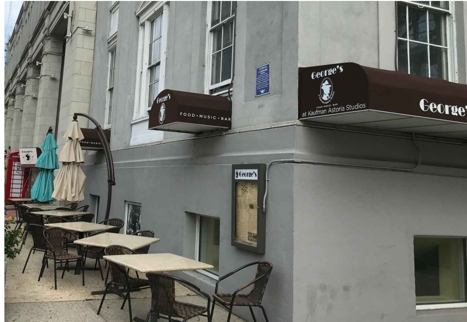
View of awnings from the corner of 36th Street & 35th Avenue
