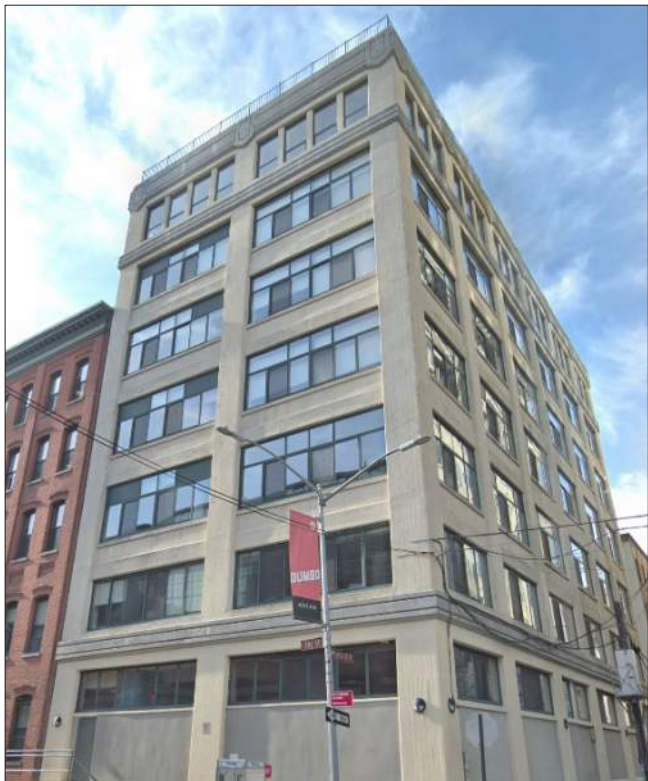
Reinforced Concrete. 42-44 Jay Street (1919-21).
