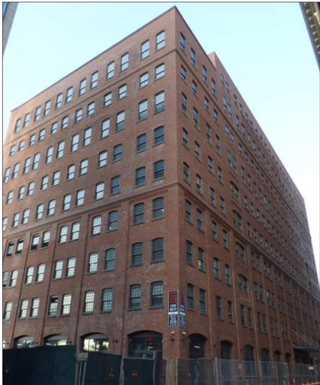
Steel Frame/Brick Curtain Wall. 10 Jay Street (1897-98).
