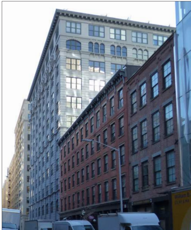
Slow-Burning Construction/Brick Facade. 66-72 Water Street (c.1850).
