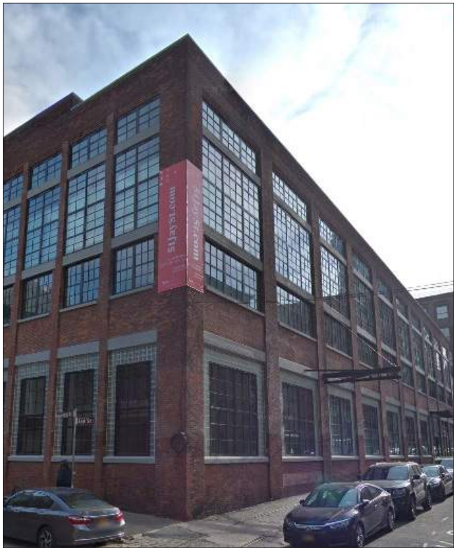
Steel Frame/Brick Curtain Wall. 51 Jay Street (1913, alt. 1930).
