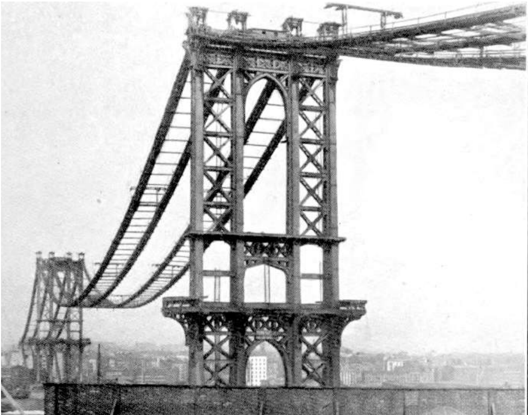
STEEL BRACED FRAME: MANHATTAN BRIDGE, 1909
