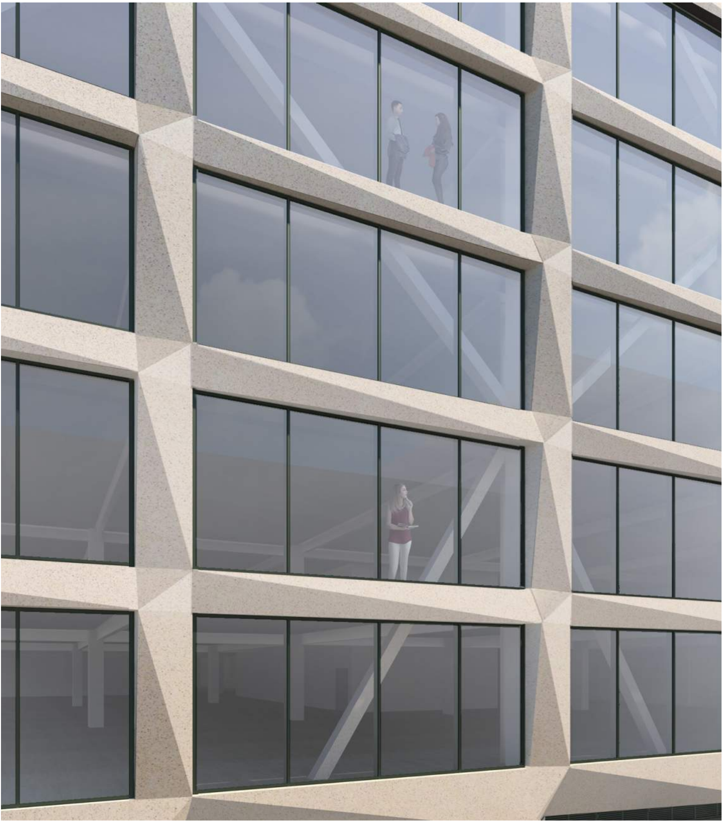
DETAIL VIEW. SHAPED PRECAST CONCRETE PANELS
