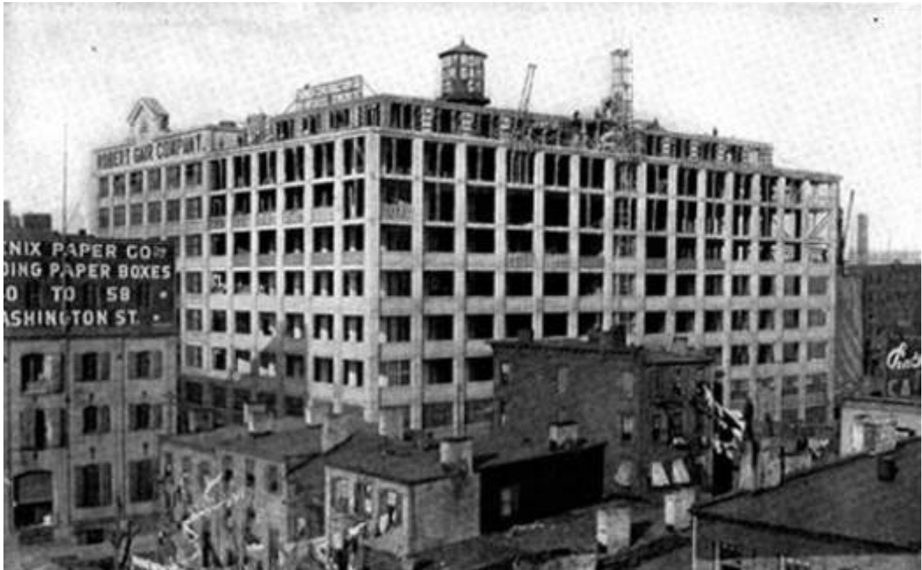
CAST IN PLACE CONCRETE: 55 WASHINGTON STREET, 1908
