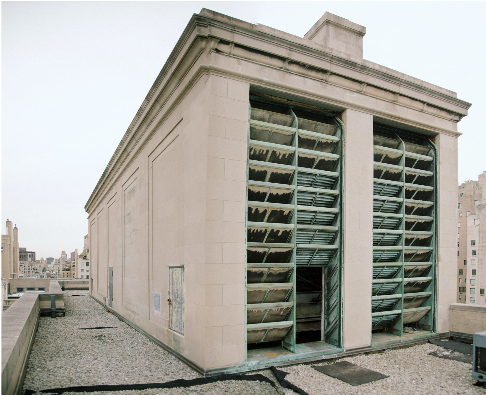
EXISTING BULKEAD, VIEW FROM SOUTH-EAST
