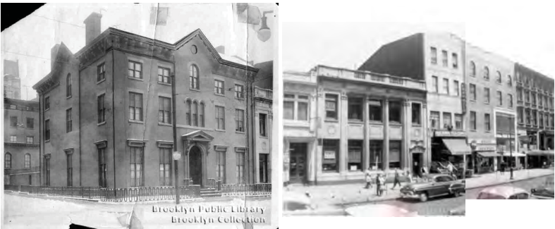
131 MONTAGUE STREET 135 MONTAGUE STREET
