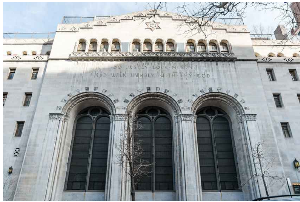
05 PRIMARY FACADE VIEW OF EXISTING
