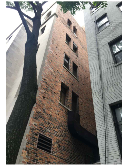
07 PRIMARY FACADE VIEW OF EXISTING
