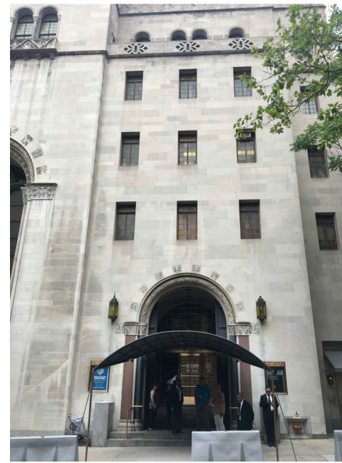
06 PRIMARY FACADE VIEW OF EXISTING
