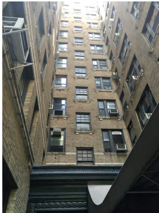
ENTRY COURTYARD FACADE: EXISTING N.T.S.
