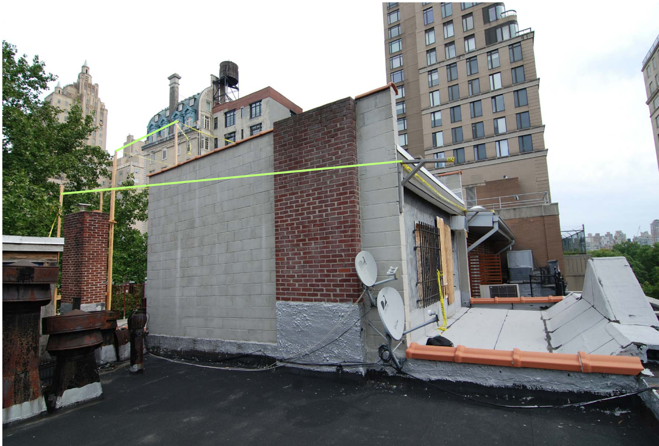
3 MOCK UP - VIEW LOOKING EAST ON ROOF 17-19 W + 21 W 88
