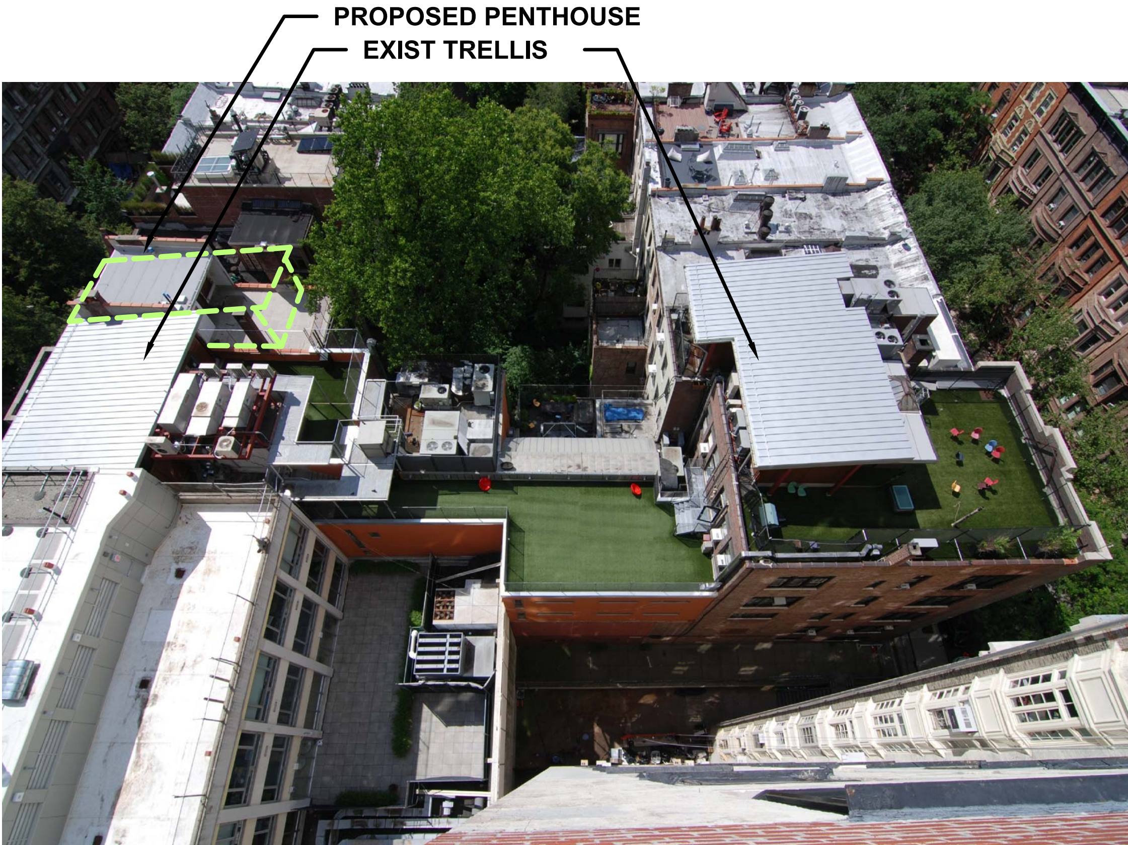
2 VIEW LOOKING DOWN ON SITE - PROPOSED 17-19W + 21W 88, 18W + 22W 89
