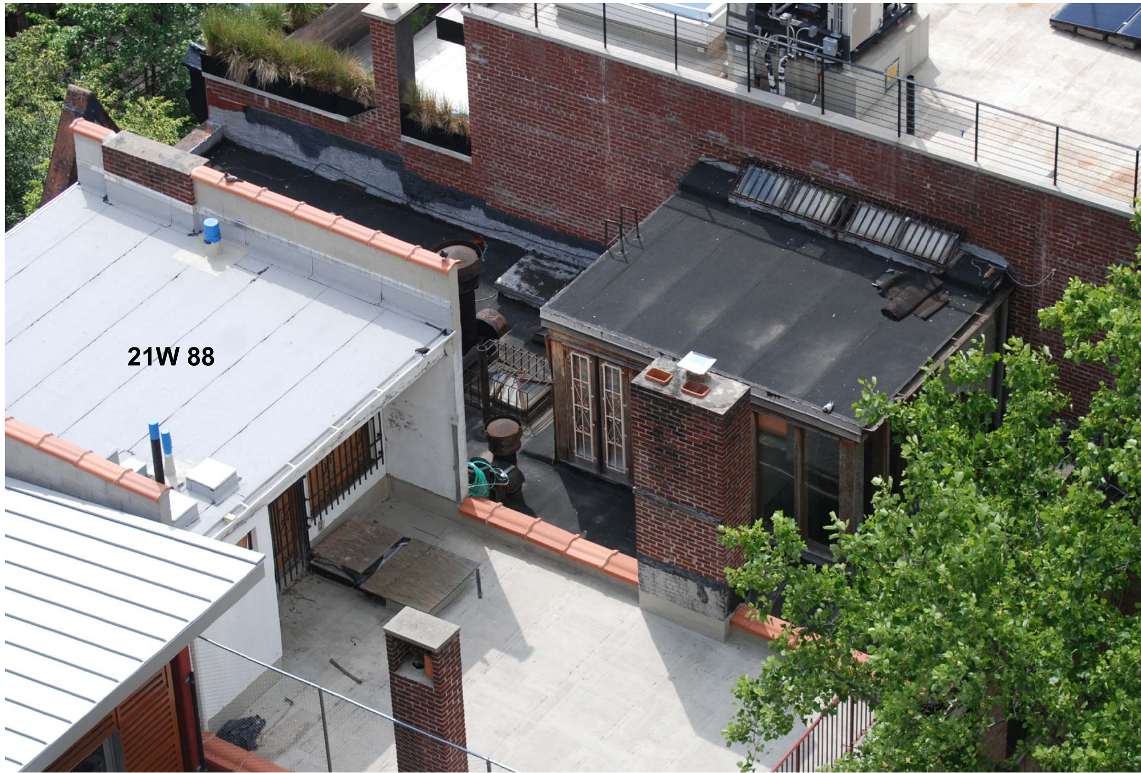
3 PENTHOUSE - EXISTING 21W, 23W & 25W 88TH STREET
