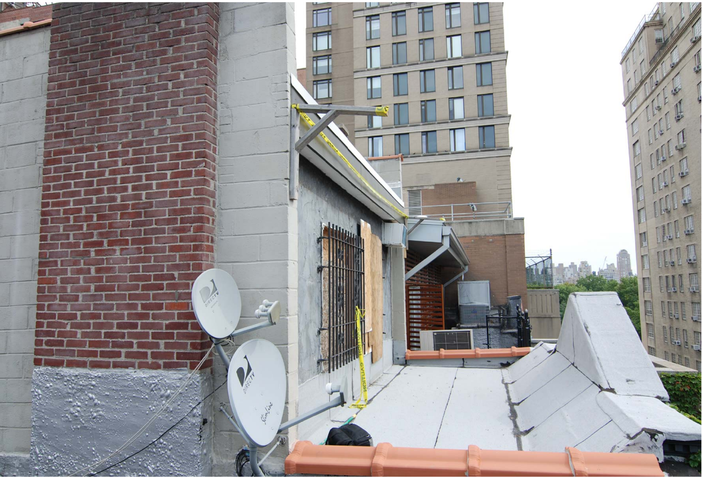
2 MOCK UP - VIEW LOOKING EAST ON ROOF 17-19 W + 21 W 88
