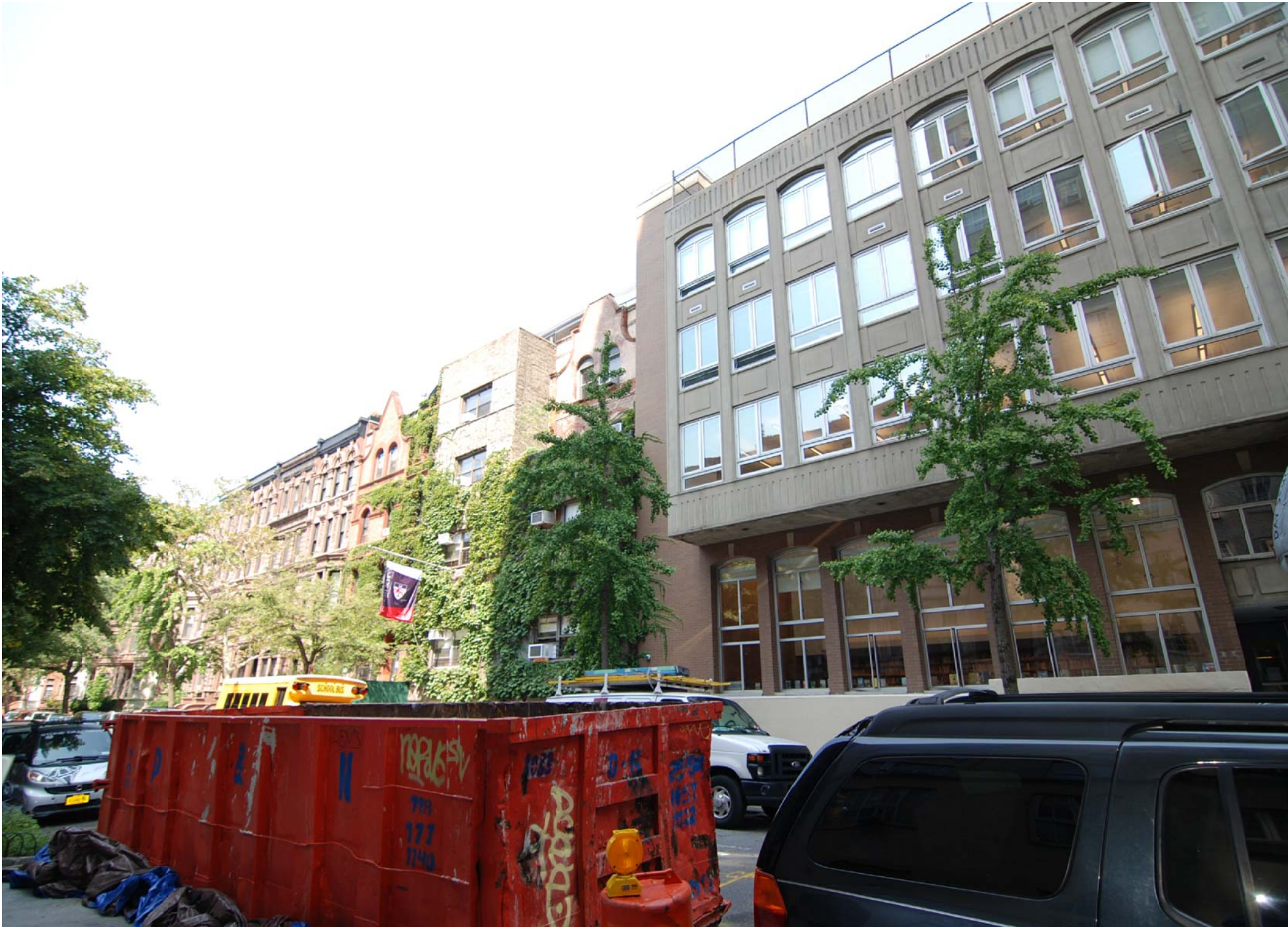
1 FRONT ELEVATION - VIEW LOOKING WEST 17-19 W + 21 W 88
