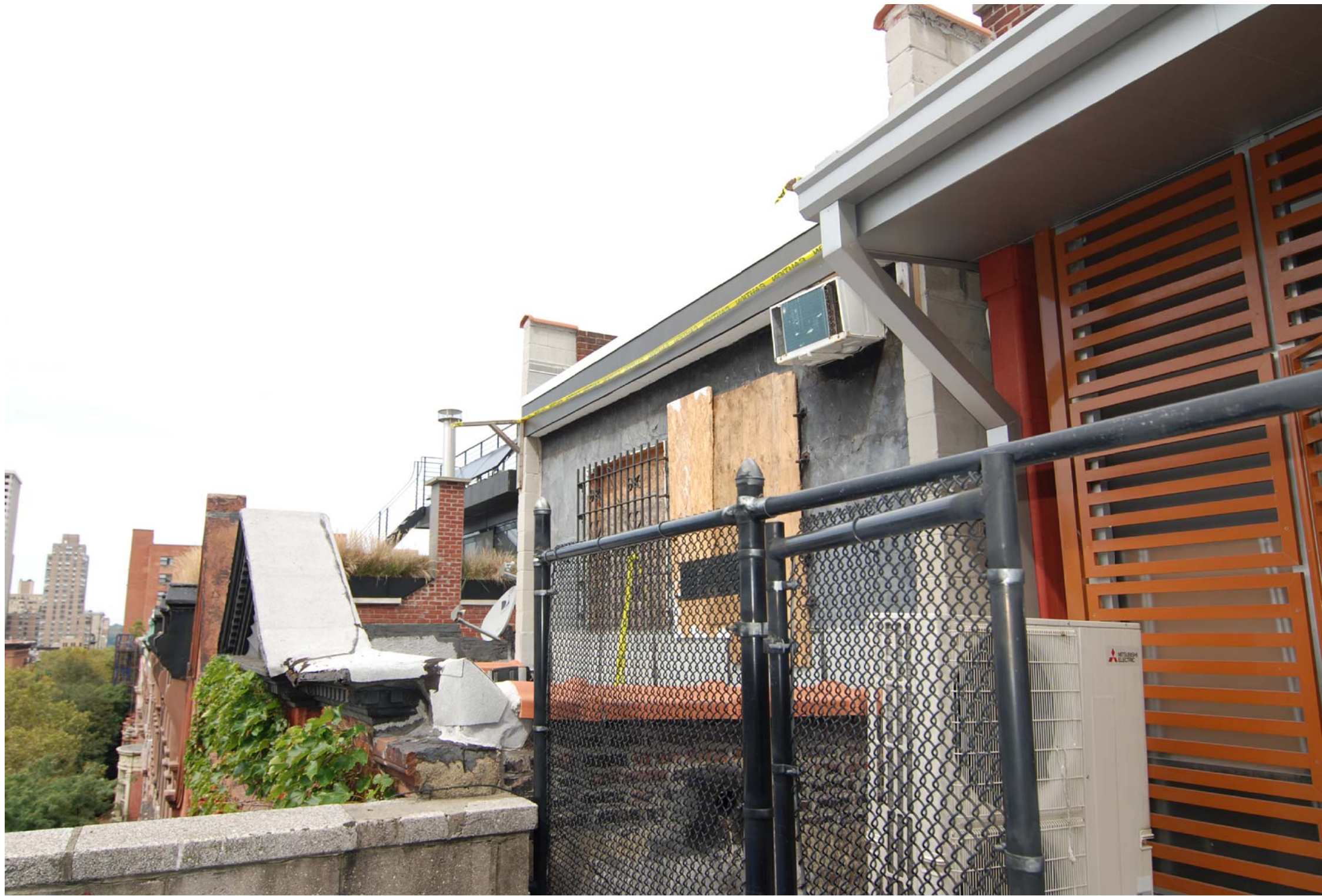
1 MOCK UP - VIEW LOOKING WEST ON ROOF 17-19 W + 21 W 88
