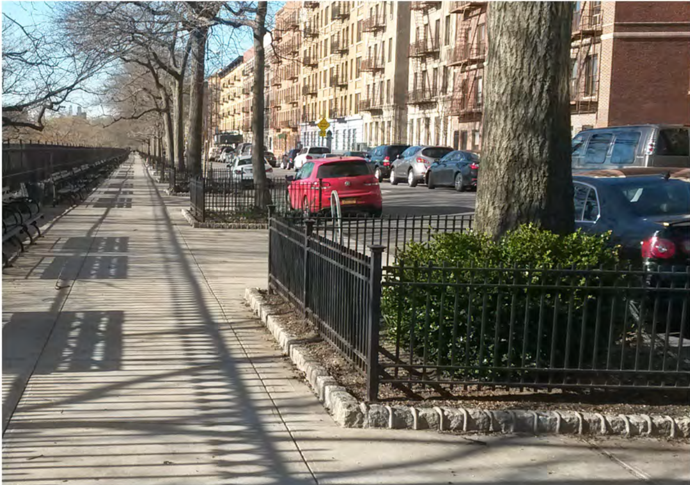
EXISTING CONDITIONS (NORTH) - GENEROUS TREE BEDS WITH STEEL GUARD AND BELGIAN BLOCK EDGE
