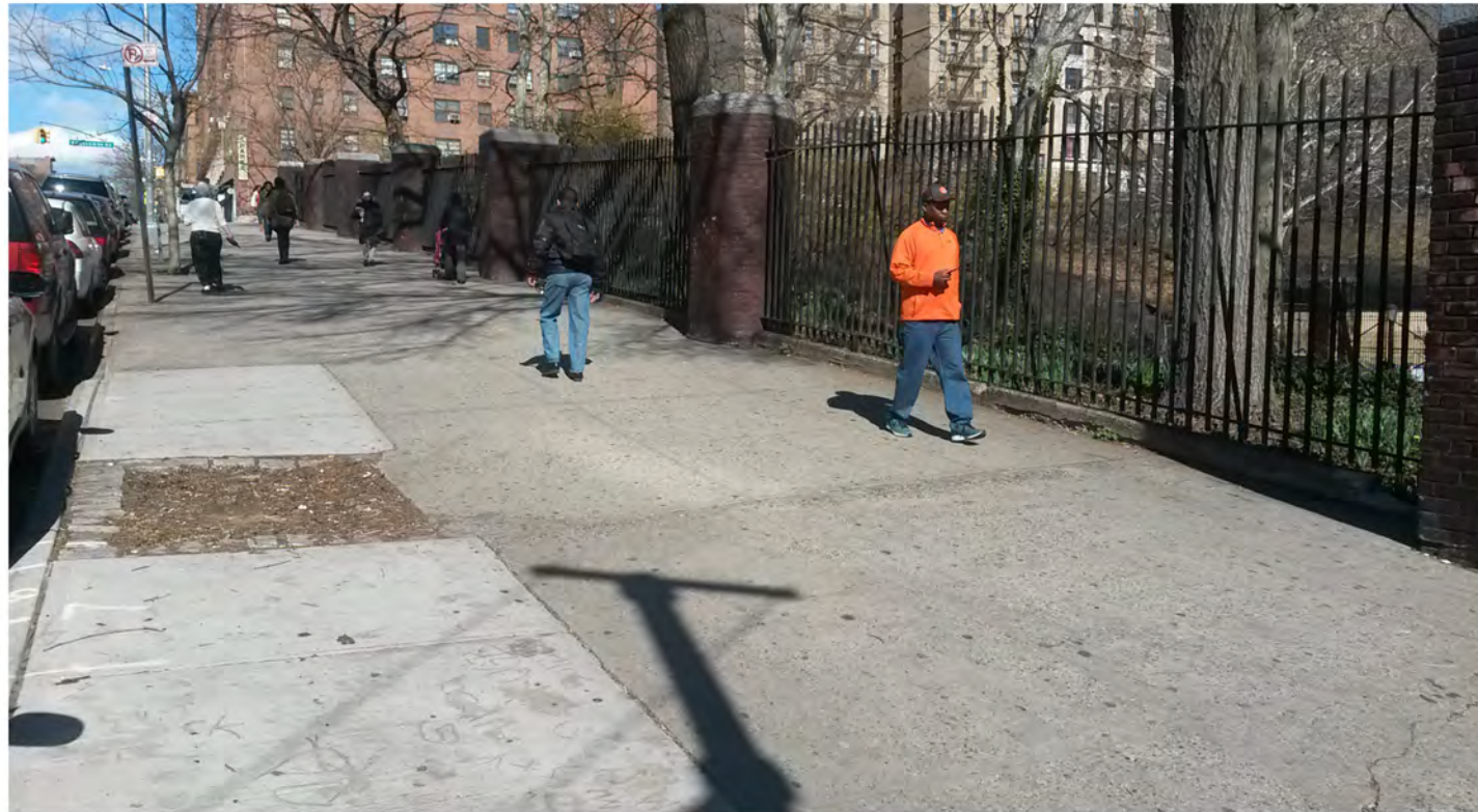
EXISTING CONDITIONS - 145TH STREET BORDER
