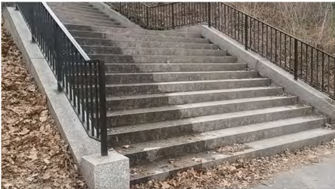
STAIRWAY HANDRAIL (ADA)
