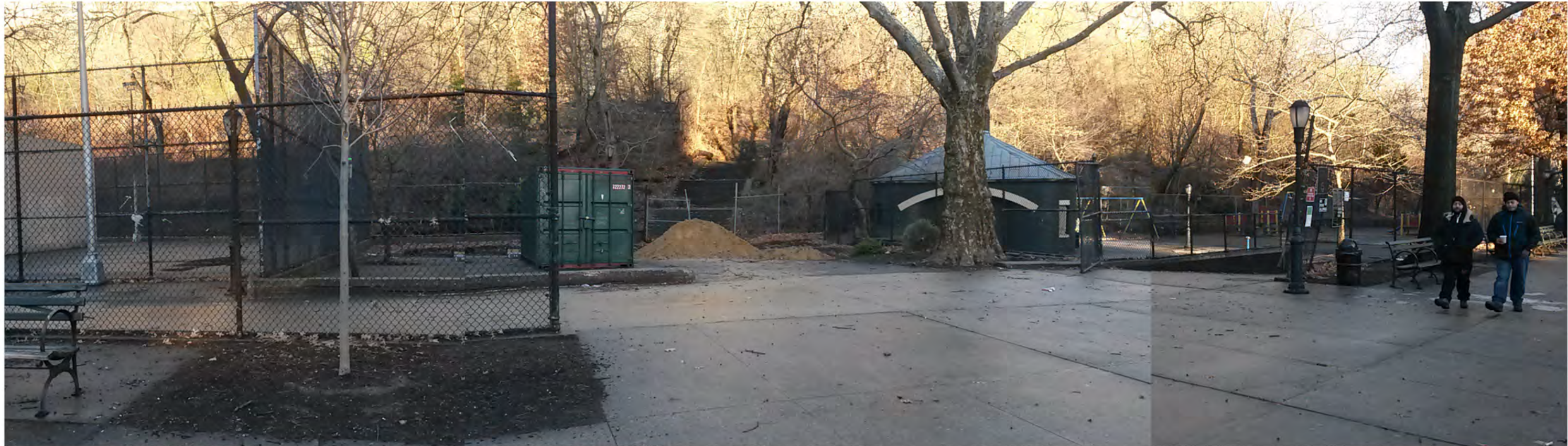
EXISTING ENTRANCE AT 152ND STREET AND BRADHURST AVENUE (PARTIALLY CLOSED)
