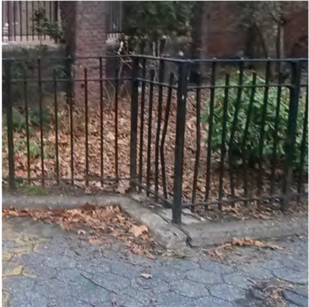
4 FT STEEL FENCE
