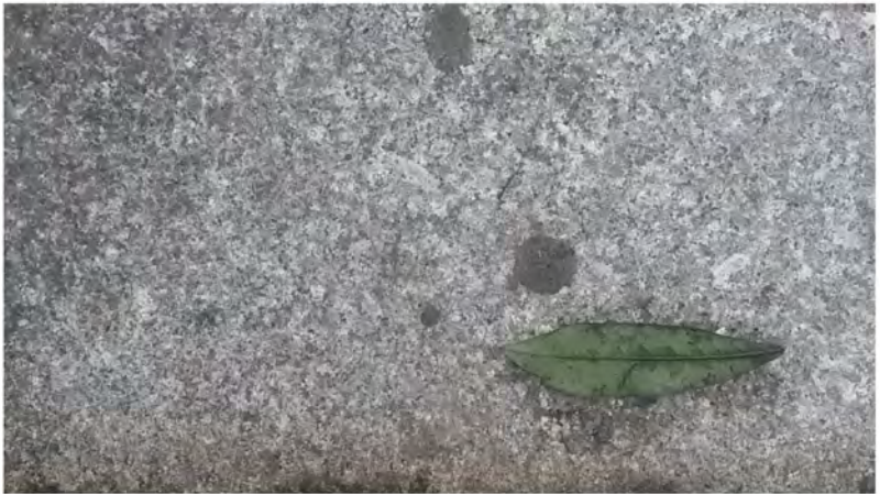
MATERIAL FOR RECONSTRUCTED STAIRWAY AT 155TH STREET AND EDGECOMBE AVENUE ENTRANCE TO MATCH EXISTING GRANITE STEPS AT ENTRANCE FROM EDGECOMBE AVENUE NEAR 150TH STREET.
