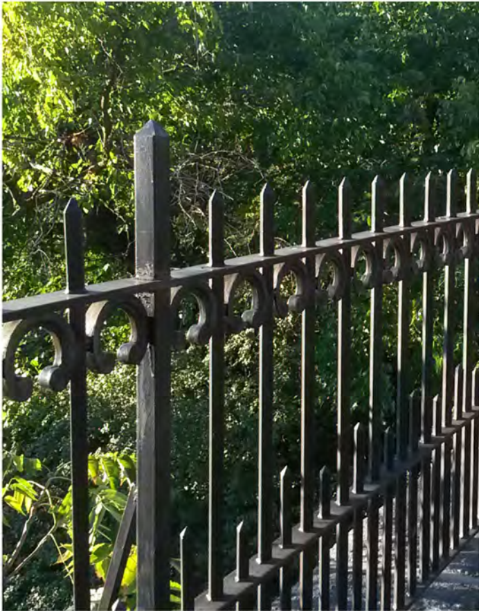
4'-0" HT DECORATIVE STEEL FENCE WITH CAST HORSESHOES, HISTORICALLY EXTENDED THE FULL LENGTH OF EDGECOMBE AVENUE. CURRENTLY FOUND ALONG EDGECOMBE AVENUE ONLY NORTH OF 150TH STREET.
