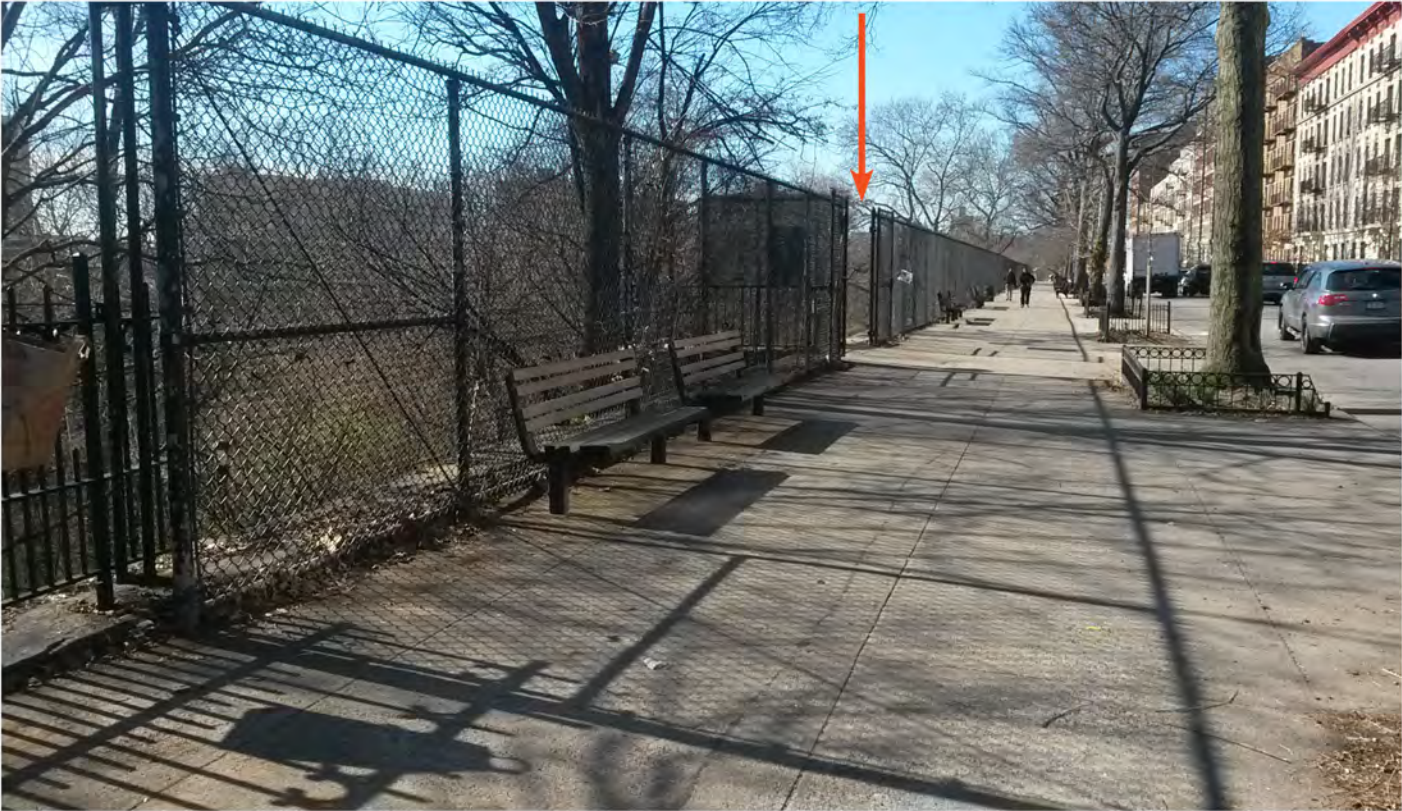
EXISTING CONDITIONS - VIEW TOWARDS ENTRANCE
