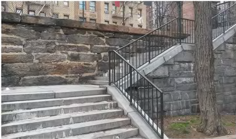
MATERIAL FOR RECONSTRUCTED STAIRWAY AT 155TH STREET AND EDGECOMBE AVENUE ENTRANCE TO MATCH EXISTING GRANITE STEPS AT ENTRANCE FROM EDGECOMBE AVENUE NEAR 150TH STREET.
