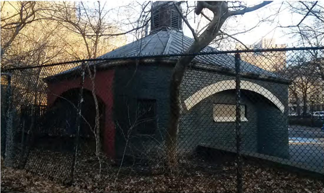
8 FT CHAIN LINK FENCE AROUND PLAYGROUND
