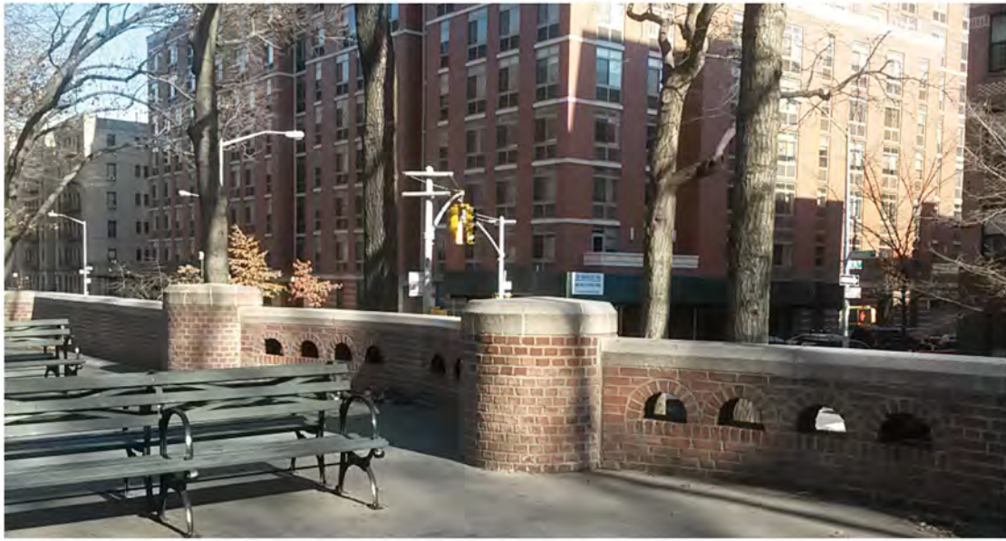
BRICKWORK AT NEARBY BANDSHELL PLAZA
