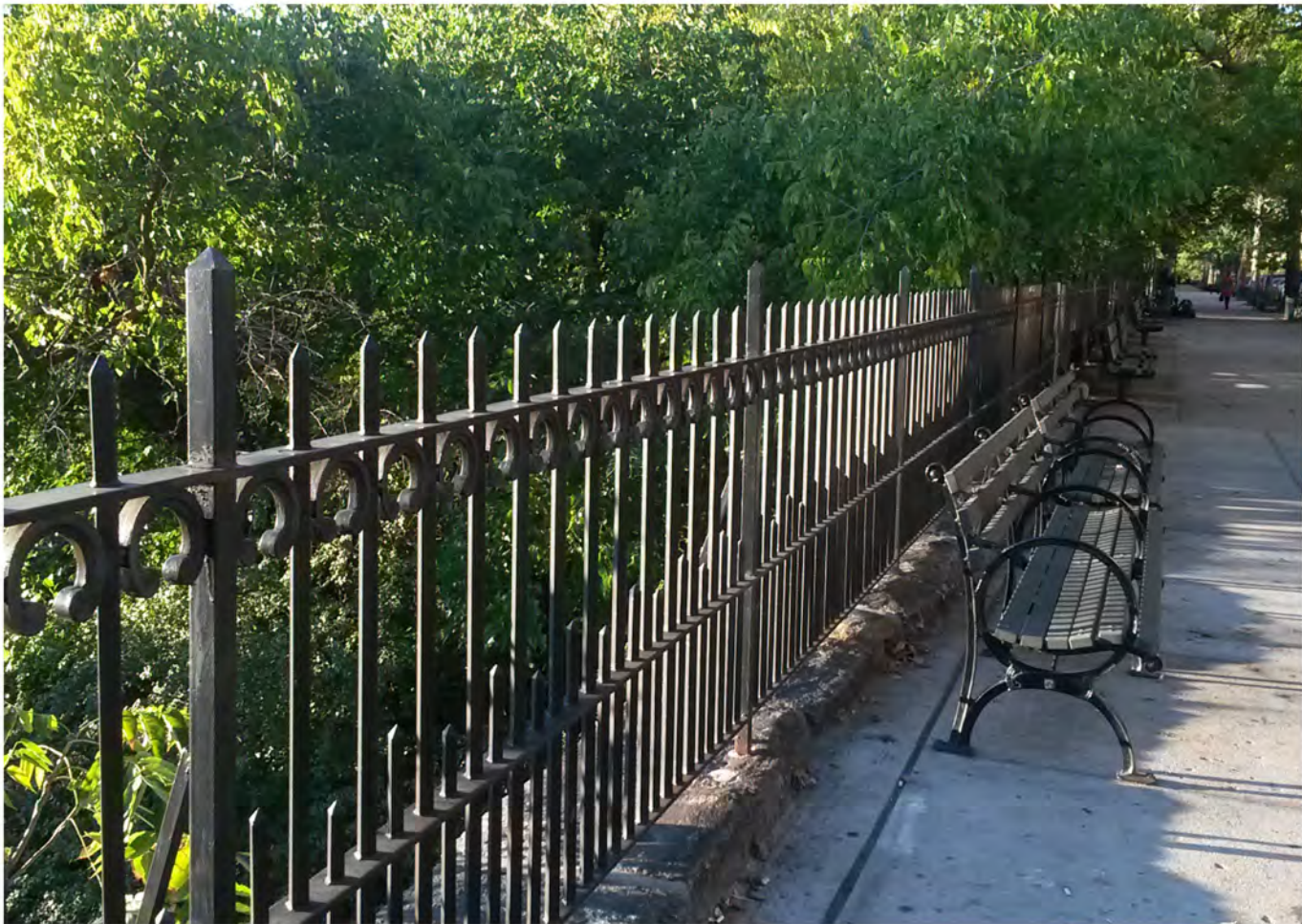
EXISTING CONDITIONS - DECORATIVE STEEL 'HORSESHOE' FENCE AND 1939 WORLD'S FAIR BENCHES
