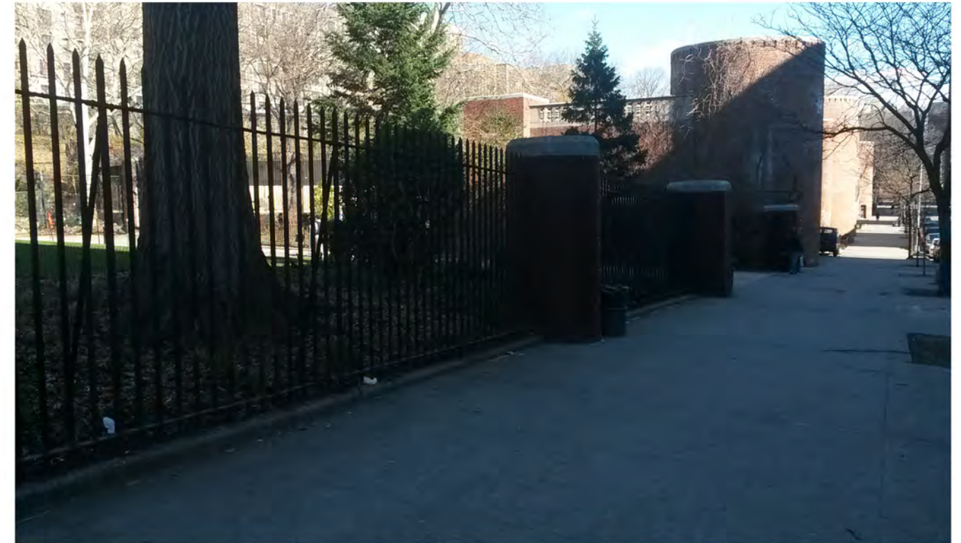
EXISTING CONDITIONS - BRADHURST AVENUE BORDER BELOW 146TH STREET
