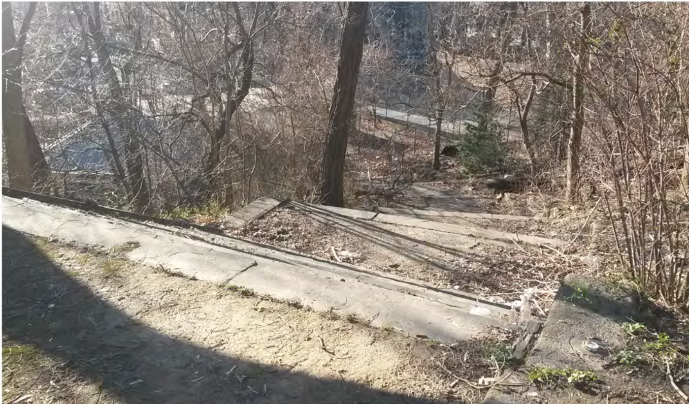
EXISTING CONDITIONS - BLUESTONE STEPS TO 152ND STREET AND BRADHURST AVENUE (CLOSED)
