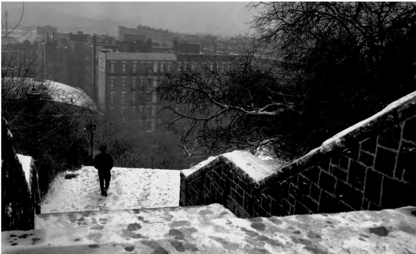
ENTRANCE STAIRWAY AT 155TH STREET AND EDGECOMBE AVENUE NORTH-WEST CORNER JACKIE ROBINSON PARK c. 1968 (NOW CLOSED) NYC Parks photo archive
