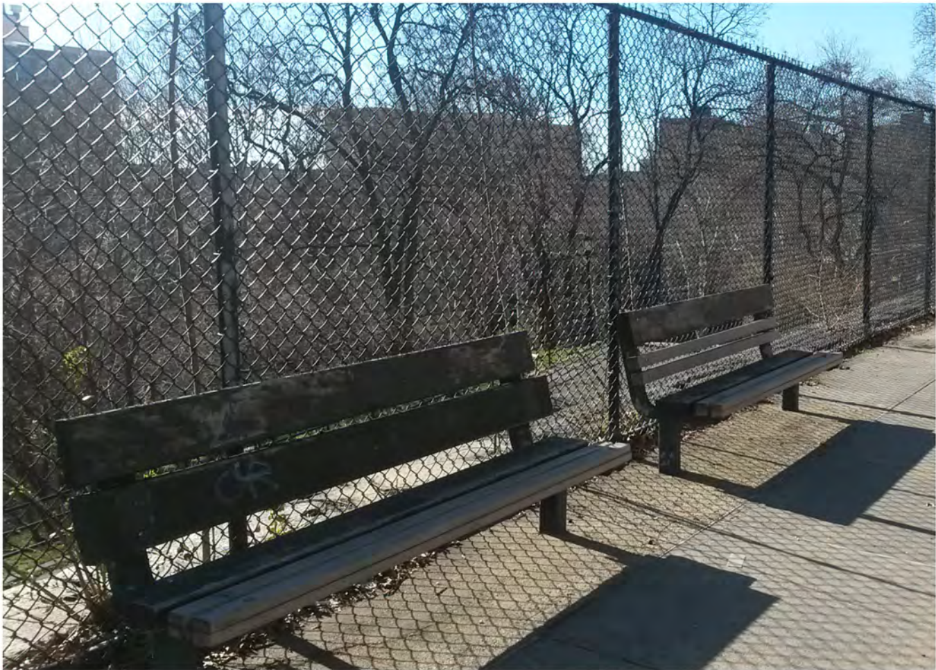
EXISTING CONDITIONS - 8FT CHAIN LINK FENCE ALONG EDGECOMBE AVENUE PROMENADE (SOUTH)
