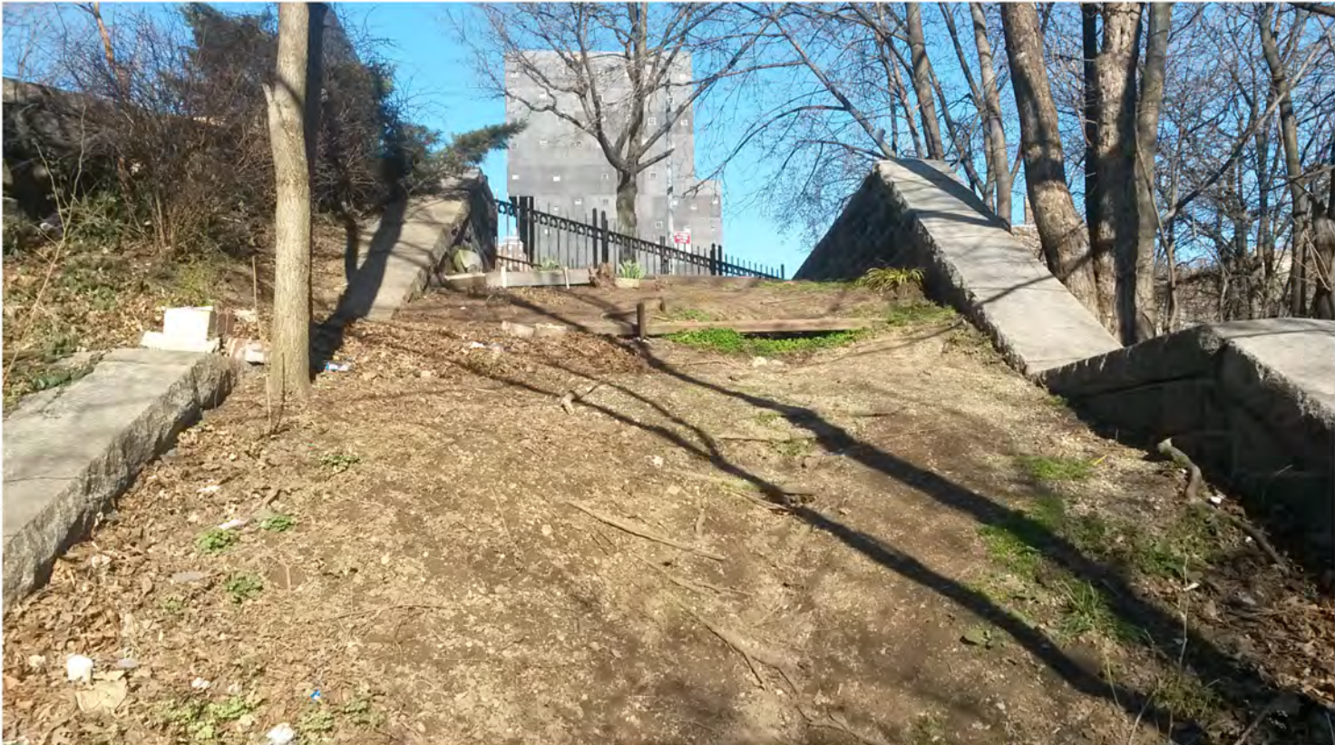
EXISTING ENTRANCE STAIRWAY AT 155TH STREET AND EDGECOMBE AVENUE (CLOSED)
