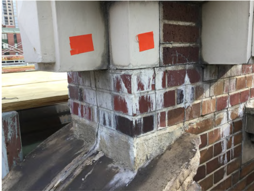
The brick below is completely cracked. The GFRP is efflorescing down the face causing salt damage to the rest of the structure and contributing to the corrosion.
