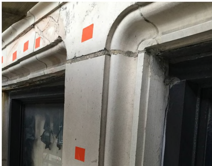
Directly below the gables, almost the entire 6 th floor lintels have completely corroded and rust jacked causing the terra cotta to crack under the pressure of the corroded steel.
