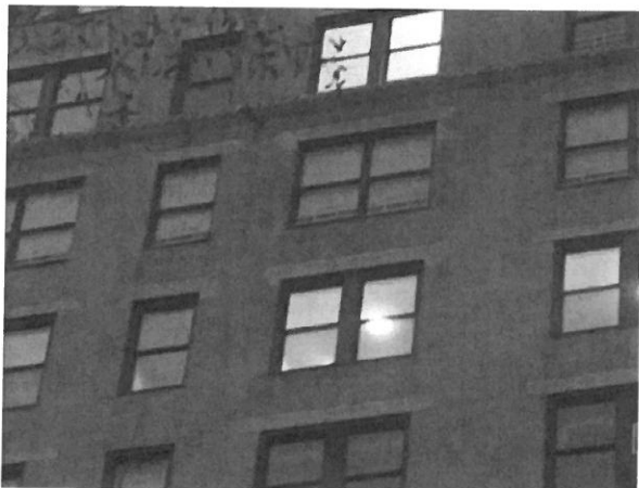
Figure 1 showing side-by-side/adjacent double-hung windows where one apartment (the one with the blinds down) has a substantially increased glass surface area. Those wider double-hung windows (with a narrower vertical mullion) allow more daylight to enter the apartment and hence reduce electricity usage and greenhouse gas emissions. The wider double-hung windows should be required by the LPC, not the narrower ones.
