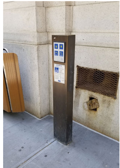
A freestanding post with a push plate door actuator, installed through non-historic paving.
