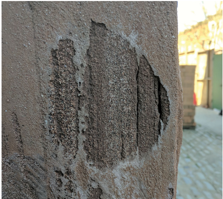
Example of a minor probe. A very small portion was carefully removed to determine the condition of the underlying material. This type of probe would not require a permit.
