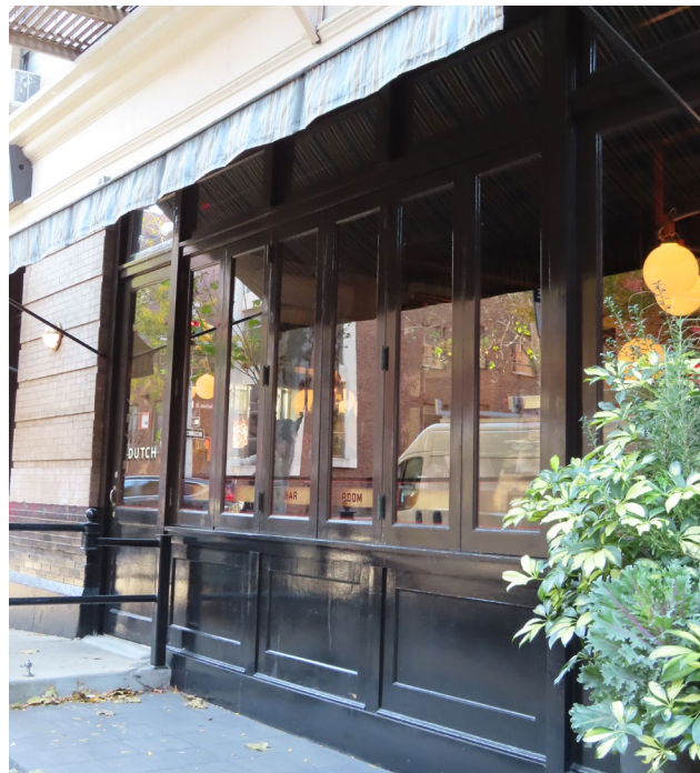
New operable storefront window featuring fixed transom windows and mullions.
