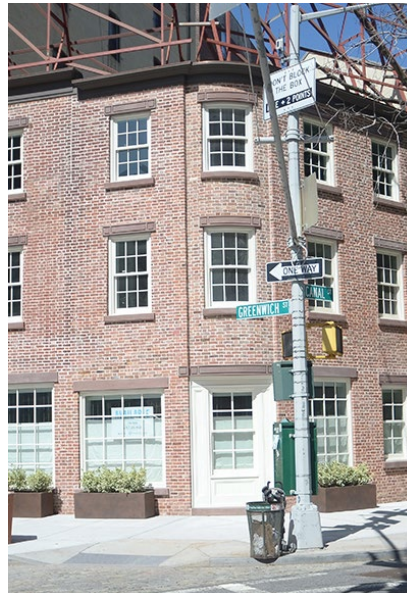
After facade reconstruction.
