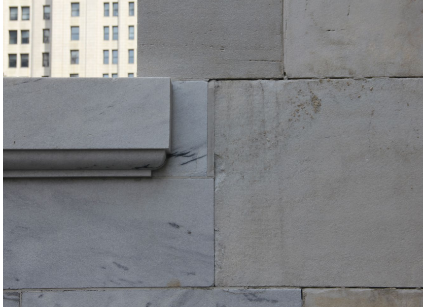
The replacement masonry (on the left) matches the historic masonry.
