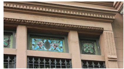
Special window featuring leaded stained glazing.
