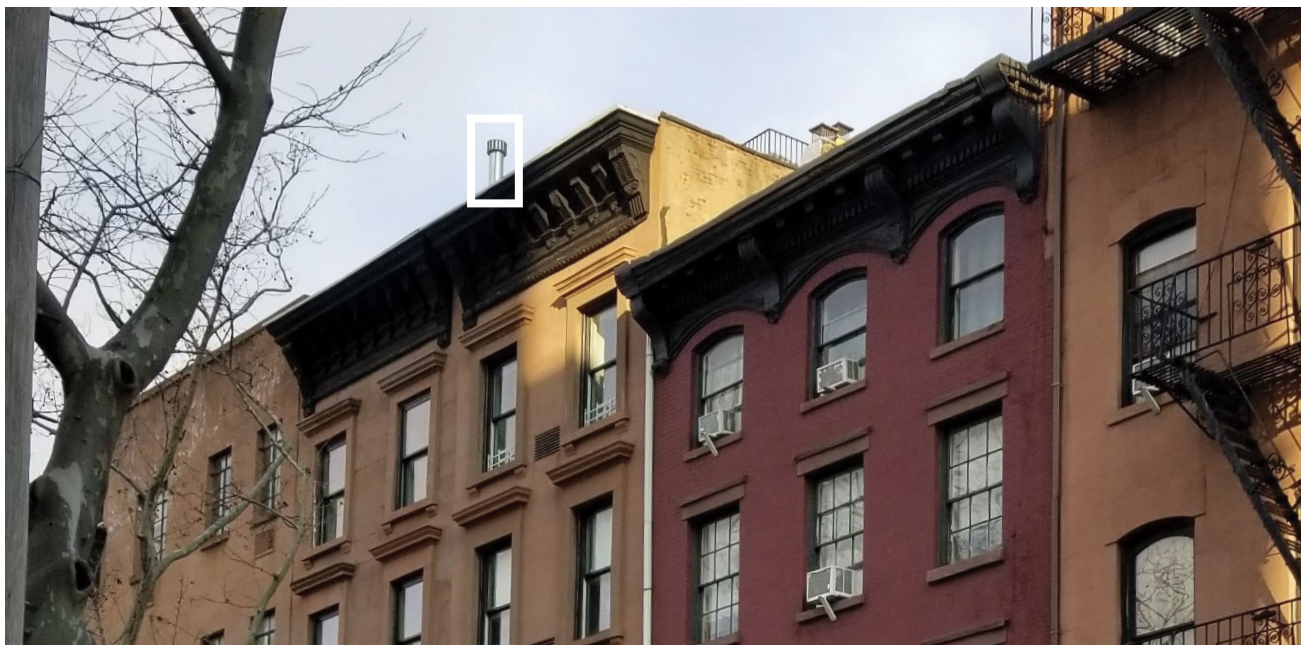
A photograph showing a chimney flue extension seen over the front facade of a row house as a result of a new rooftop bulkhead. The bulkhead itself is not visible from public thoroughfares.
