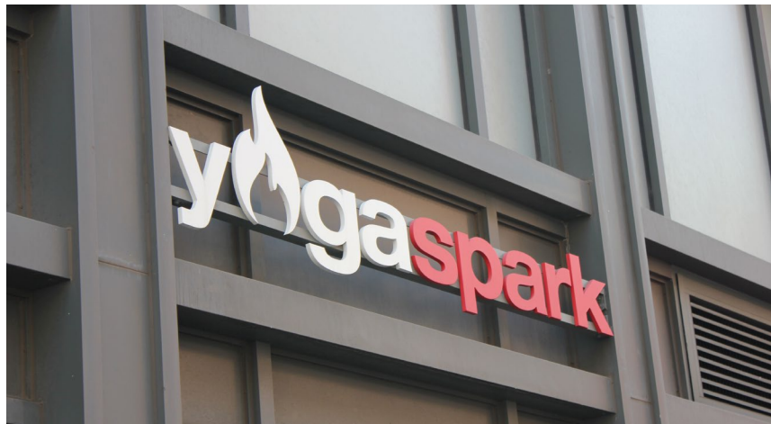
Lettering mounted on a metal channel within a transom.
