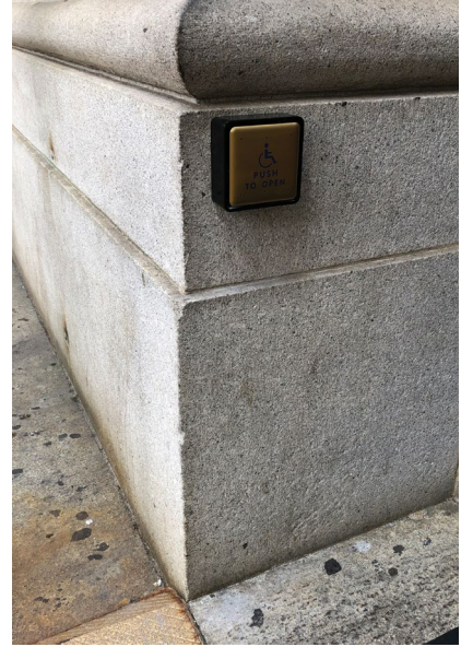
A push plate door actuator installed at an area of plain masonry.
