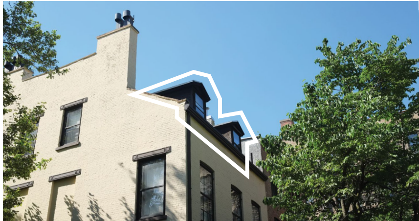
Dormers at a pitched roof facing the rear yard.
