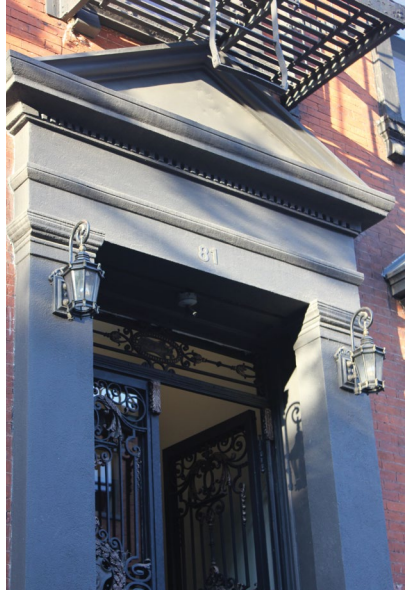
Staff can approve light fixtures installed at plain masonry adjacent to a door opening, as seen here, or within the opening.
