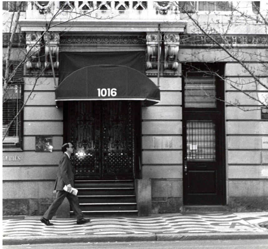
A decorative terrazzo (concrete and marble chips) sidewalk designed by artist Alexander Calder in the Metropolitan Museum Historic District.
