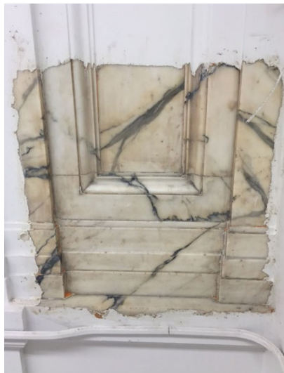
Coating removal without damaging the historic material
