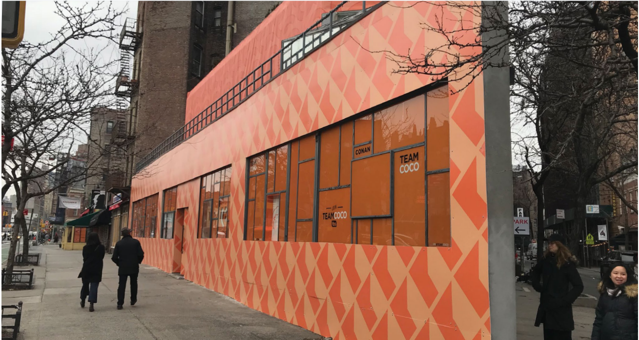
Vinyl panels and window films temporarily installed at a primary facade.
