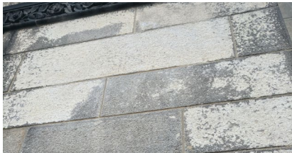
Heavy sandblasting scarred the surface of the masonry, contributing to its deterioration.
