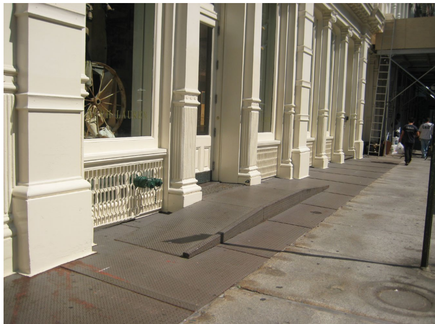
A simple ramp designed in steel diamond plate without handrails in the SoHo-Cast Iron Historic District.
