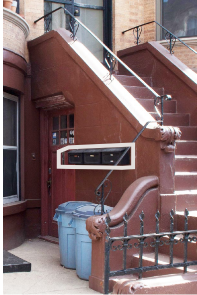
Mailboxes can be installed at a plain masonry stoop wall adjacent to a basement-level entrance door.
