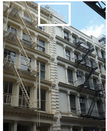
An elevator bulkhead visible over a front facade in the SoHo Historic District.
