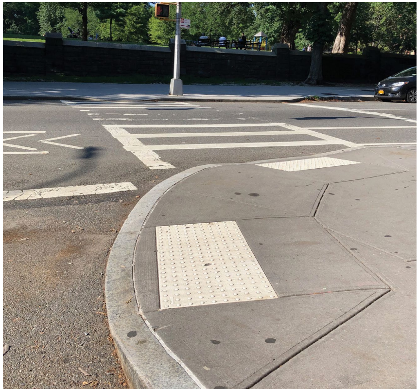
Detectable warning units embedded in a concrete pedestrian ramp.
