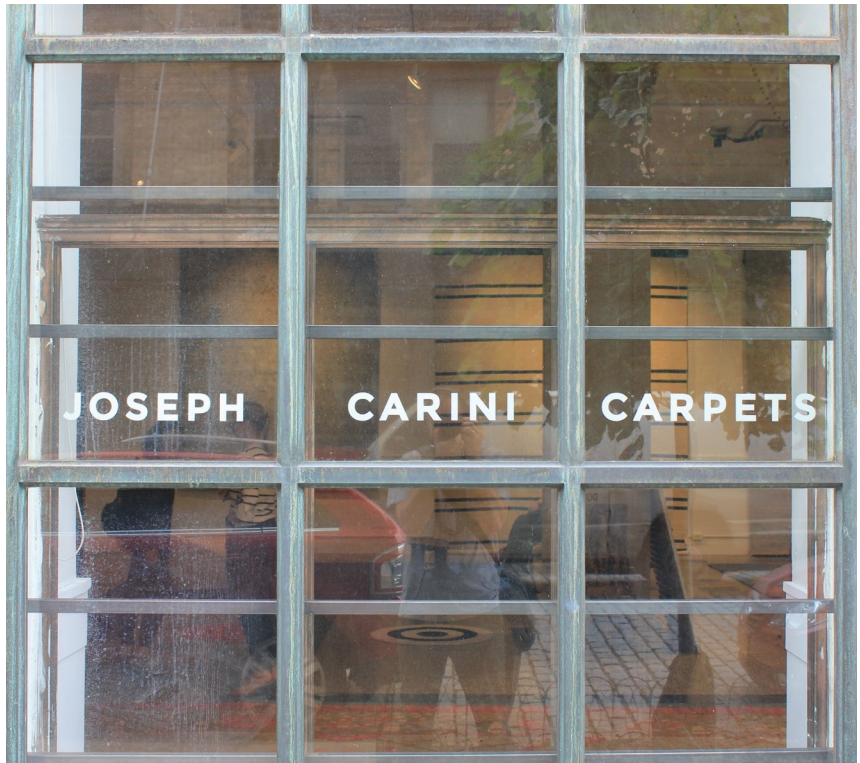
Vinyl lettering applied to storefront glazing.
