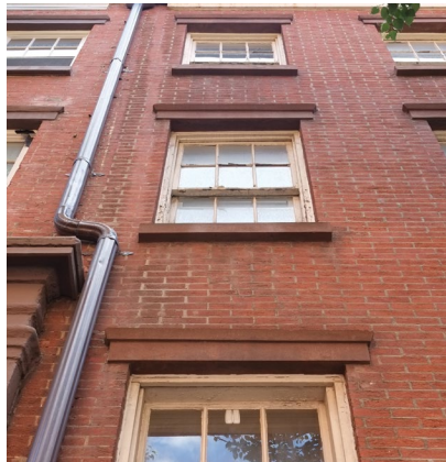
Original windows that date from 1850 or earlier are special windows.
