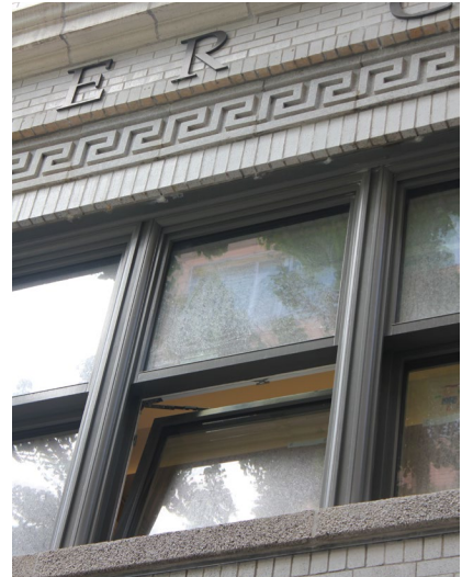
A high-performance simulated double-hung window with its lower sash tilted in is an acceptable variation in window operation.
