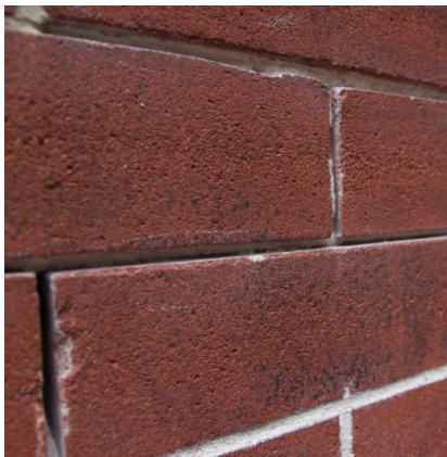
An example of careful mortar joint removal.
