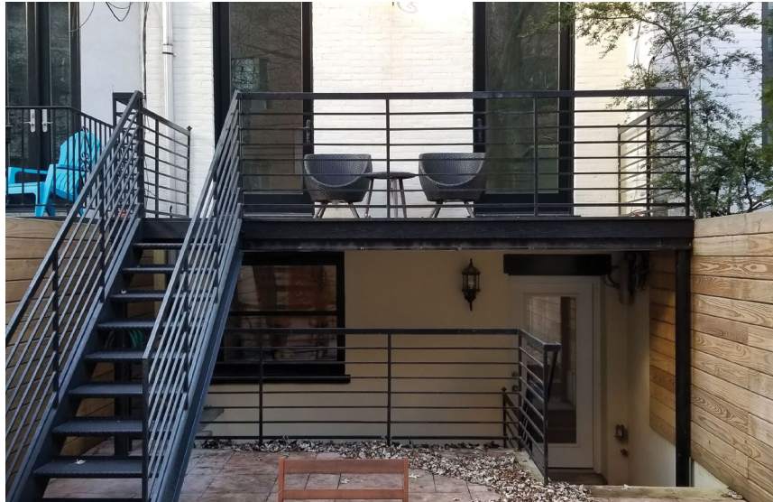
This metal deck extends eight feet from the rear facade, plus stairs.
