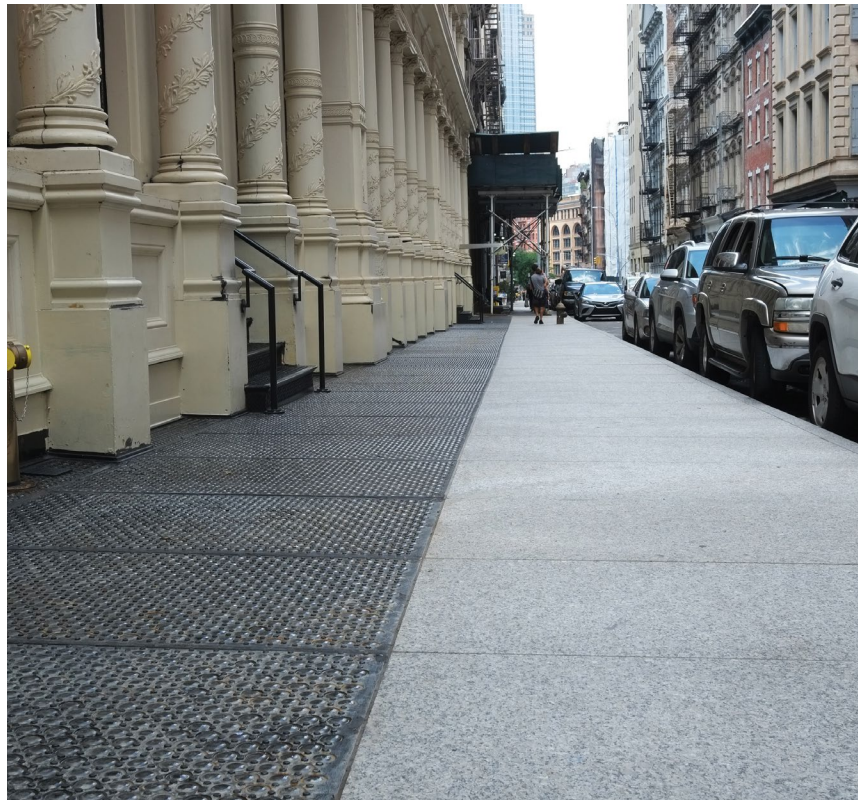
A new granite sidewalk installed next to cast iron vault lights.
