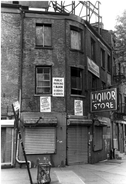
Before facade reconstruction.
