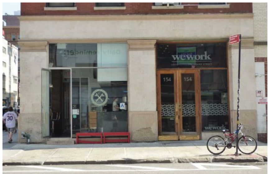
A storefront display window, top, was renovated to include a new door opening, bottom.
