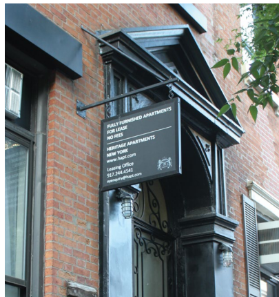
A bracket sign temporarily affixed to a facade.
