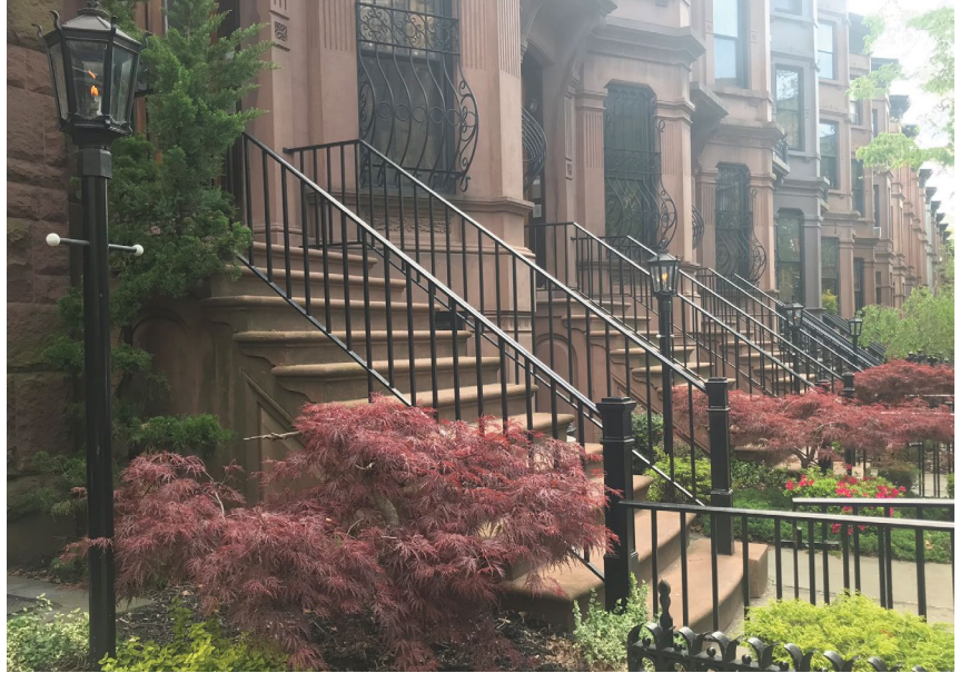
Lampposts in a black painted finish installed in a rowhouse areaway.
