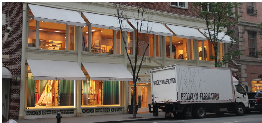
Awnings on second-story display windows are subject to the same criteria as awnings on ground-floor storefronts.
