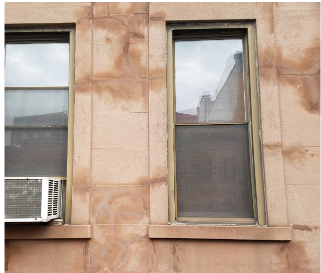
Example of inappropriate coating. Repair mortars and patching compounds should be tinted to match the original material, not the coated and/or stained materials.
