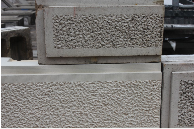
Replacement terra cotta unit (bottom) next to a piece of historic terra cotta (top).
