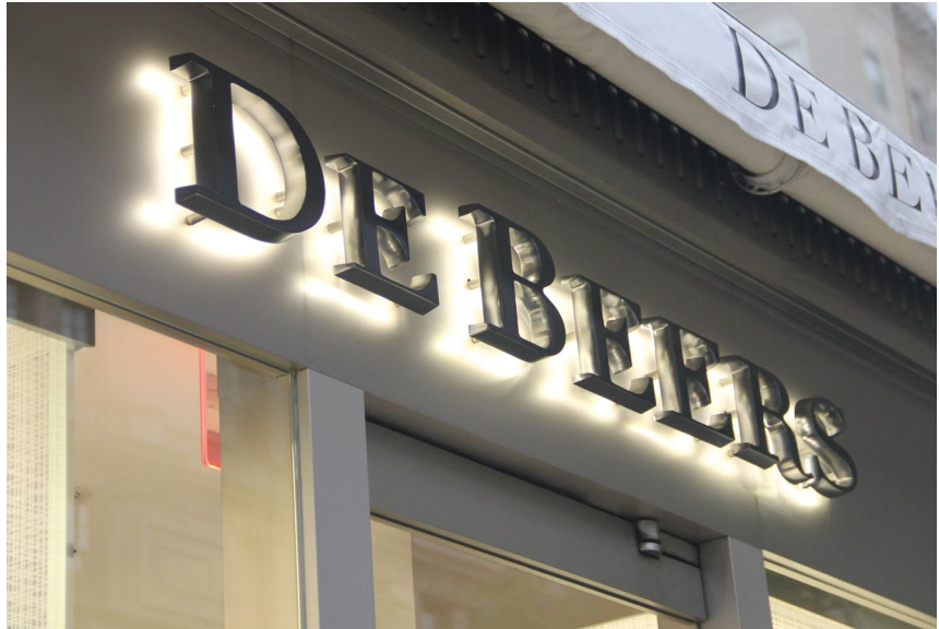
Halo-lit, pin-mounted lettering at a signband.
