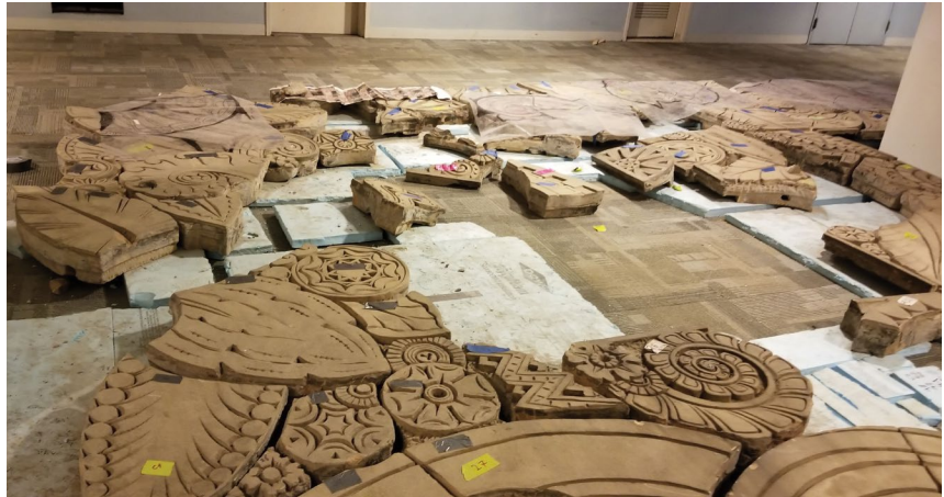
Architectural features, such as these decorative terra cotta spandrels, may be temporarily removed and stored while construction is in progress.
