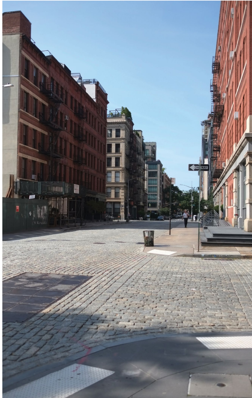
An intersection with tinted concrete paving, granite curbs and detectable warning units next to Belgian block streets.
