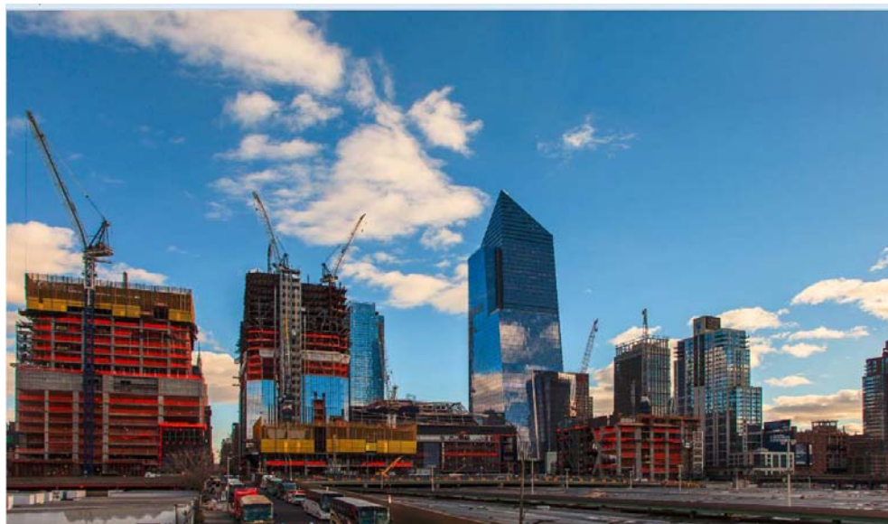
View of Hudson Yards construction, looking east from Twelfth Avenue and West 33 rd Street
