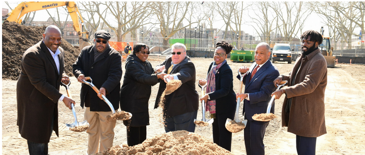
Above: Community leaders, elected officials, and City representatives at the groundbreaking for the start of Betsy Head Park renovations. Photo courtesy of NYC Parks.
