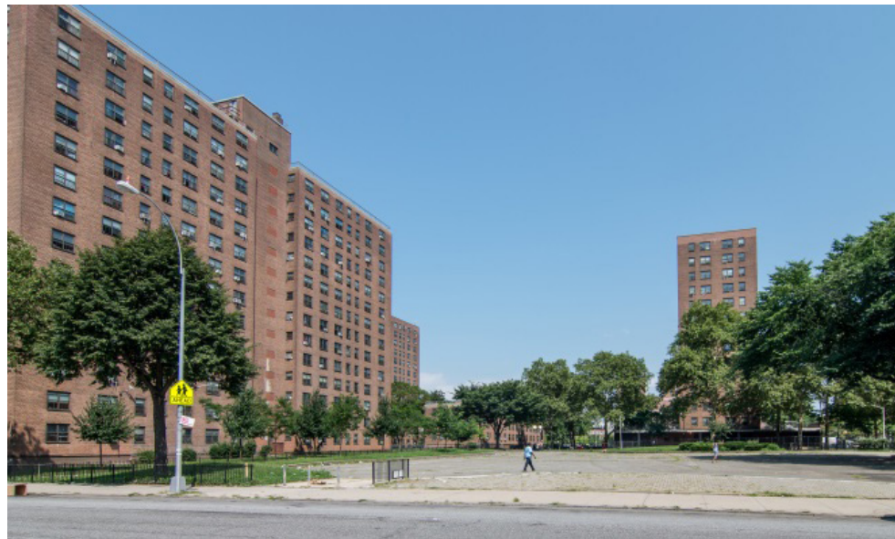
Fig. 4 Van Dyke Houses, Photo courtesy of Brownsville 100 Days.
