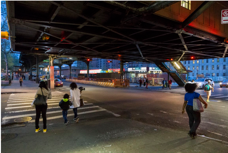
Rockaway Ave station under the elevated train - DOT
