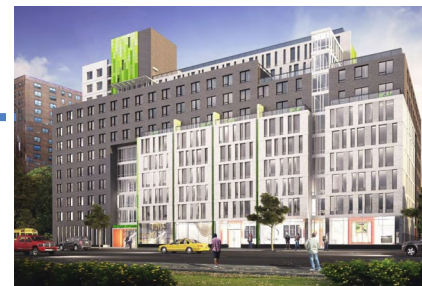
VAN DYKE III (UNDR CONSTR)
