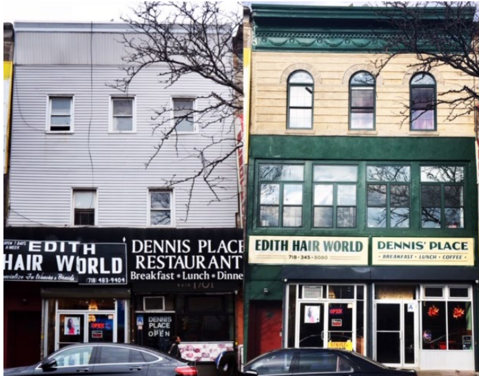
Storefront improvements of 1701 Pitkin (before and after)
