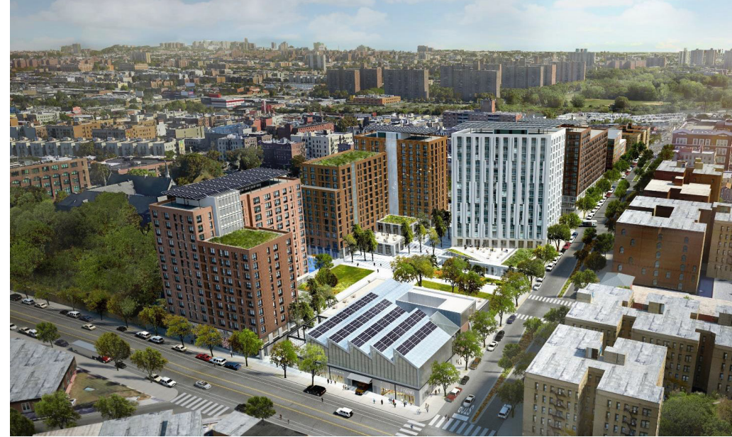
Spofford Detention Center will be a mixed use 100% affordable housing development as part of the larger redevelopment of the former Spofford Juvenile Detention Center located in the Hunts Point section of the Bronx. HIF financed the demolition of the detention center, environmental remediation, foundation work and the construction of a public plaza space.
