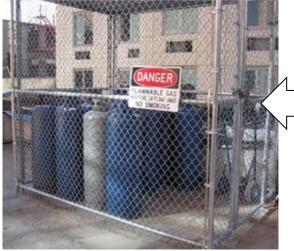
The propane cylinders must be stored in a well-ventilated outdoor enclosure secured by a lock. They must not be stored in any below grade area.
